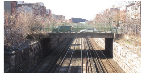
East 188th St Bridge
