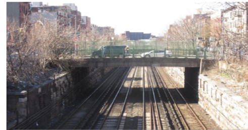
East 188th St Bridge
