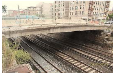
East 183 rd St Bridge
