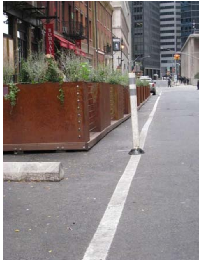
Flexible bollards, striping and parking stop at the Pearl Street site
