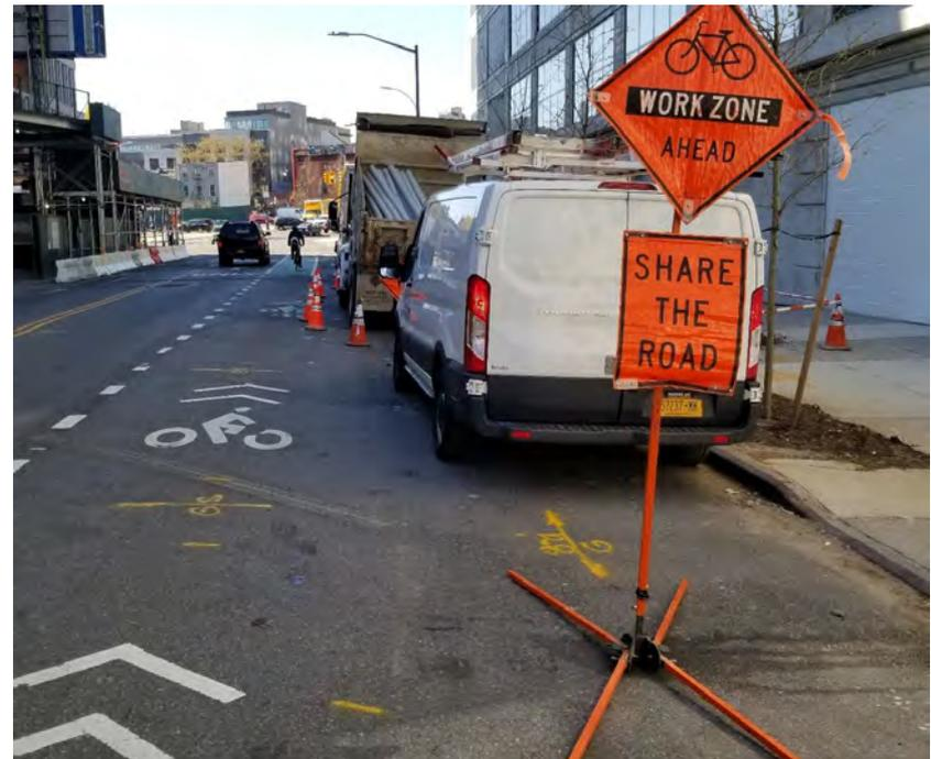
Correct assembly of Work Zone Ahead and placement
