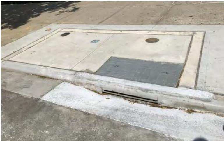
Left: Infiltration Basin with Concrete Top
