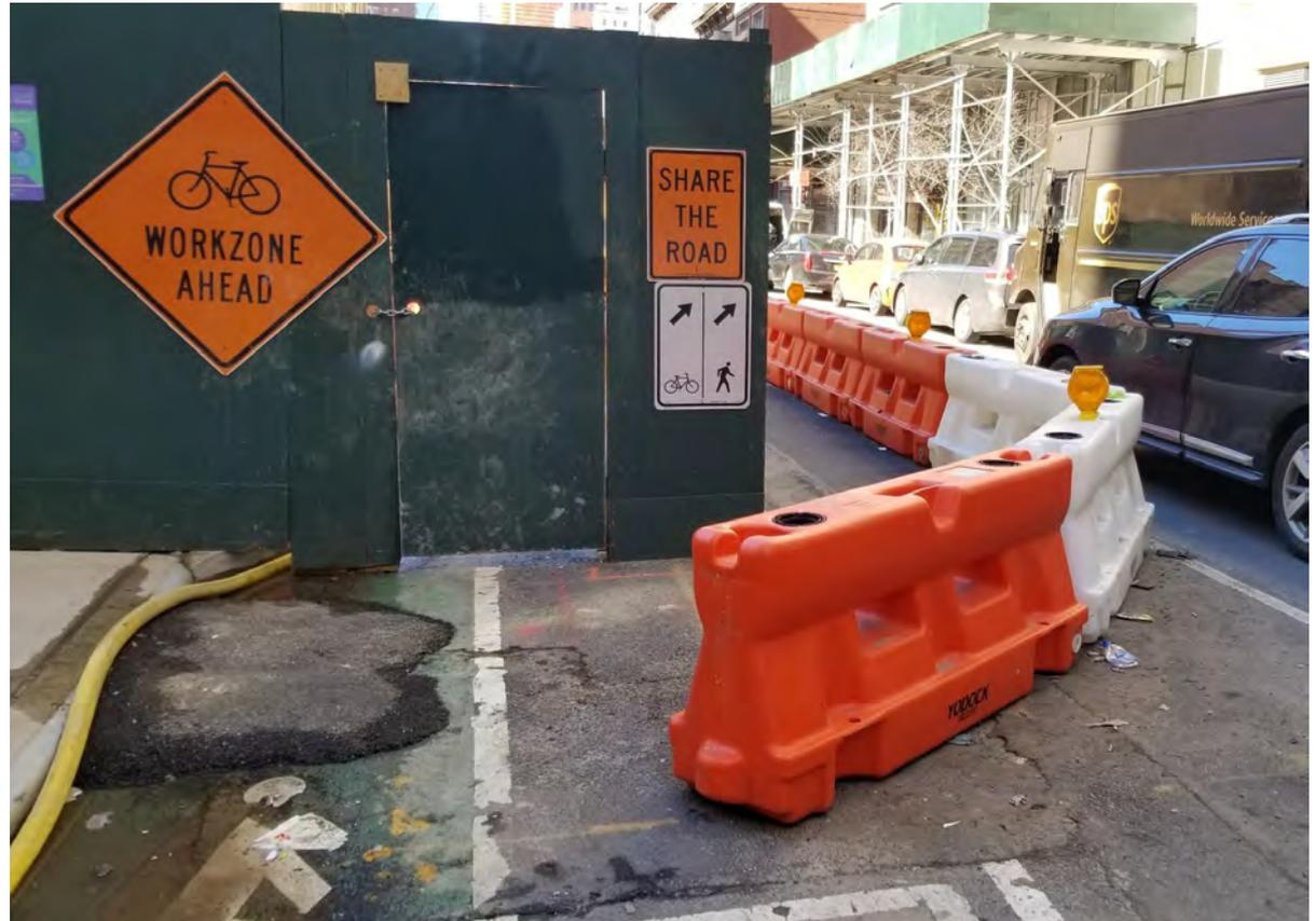
Work zone ahead sign is placed at the work zone. The bicycle and pedestrian signage is confusing about where to go, To further confuse the situation is the Share the Road sign.
