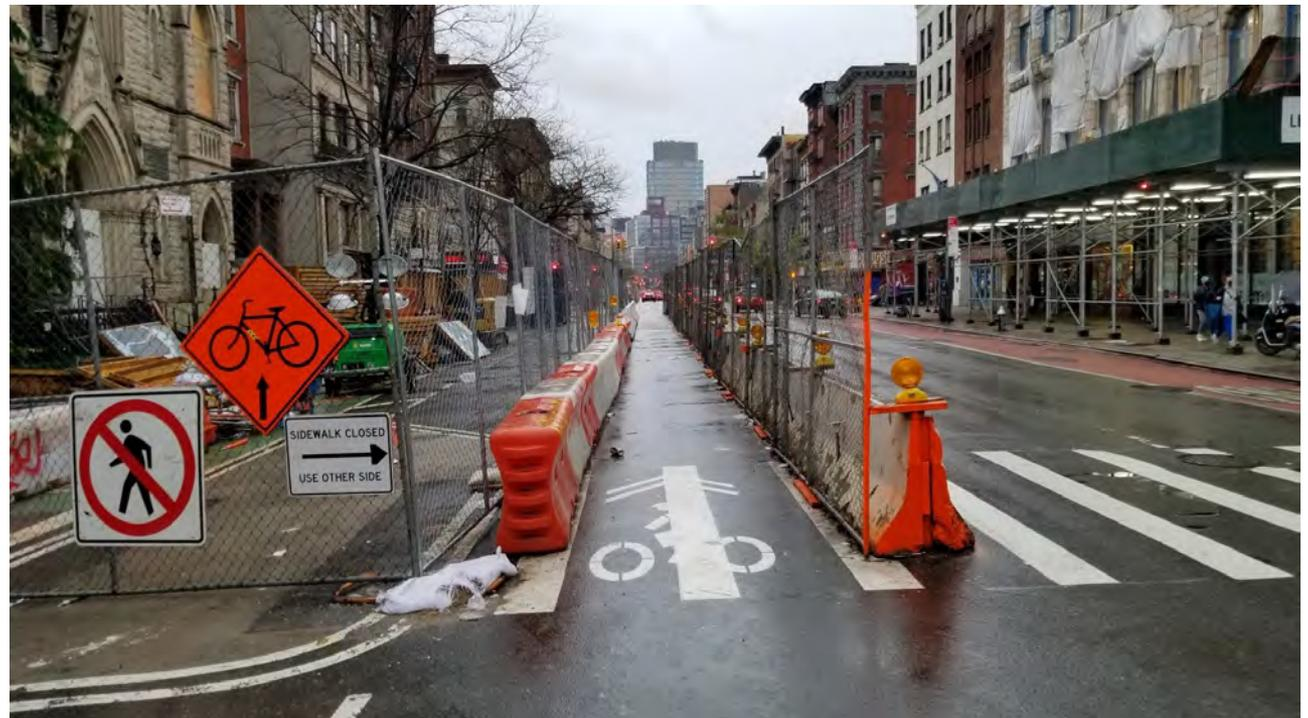
Placement of markings and type of markings is incorrectly installed making the information illegible.
