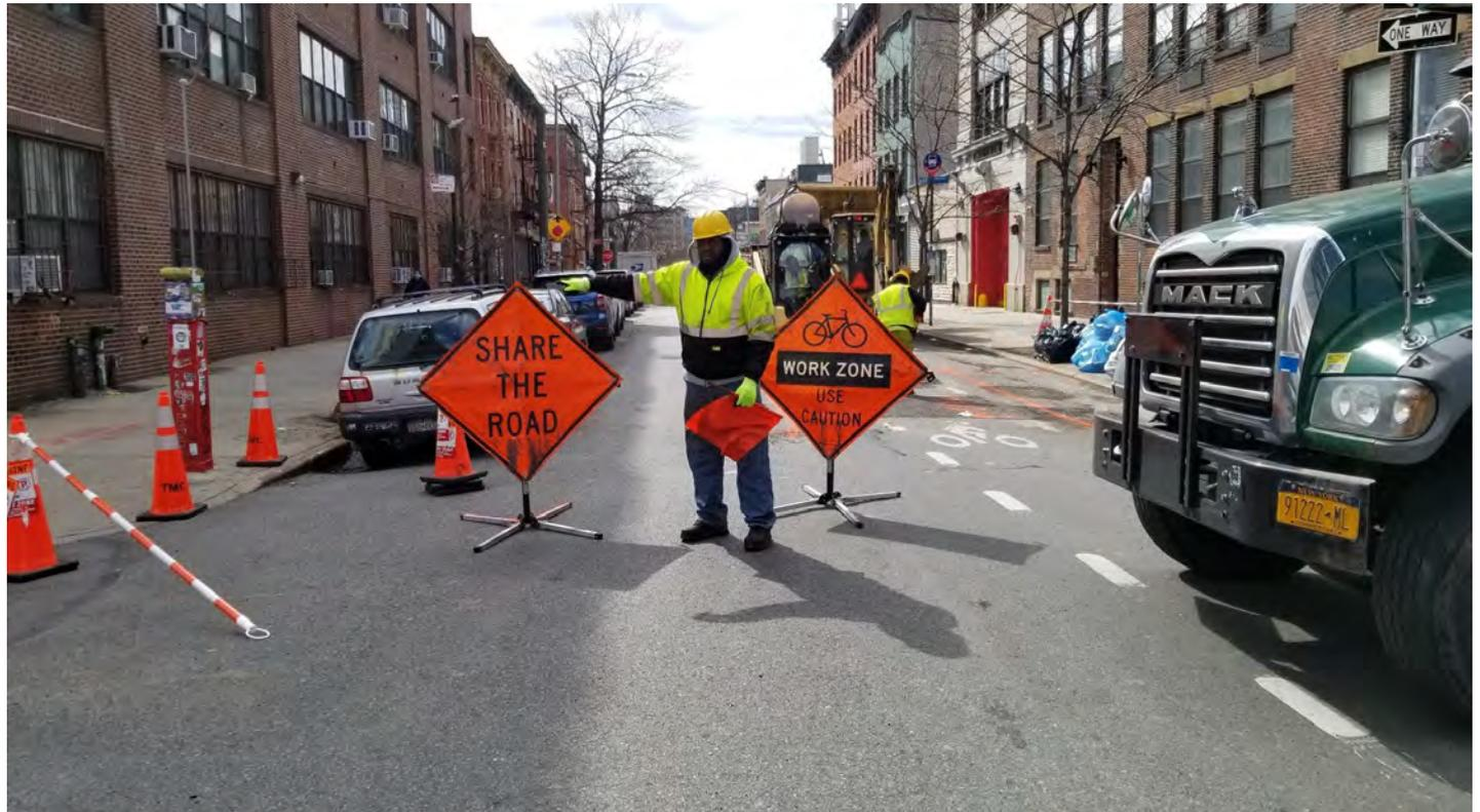
The signage indicates one direction, but the flagger is directing cyclist to perform a different maneuver . Also, signage requires better placement.
