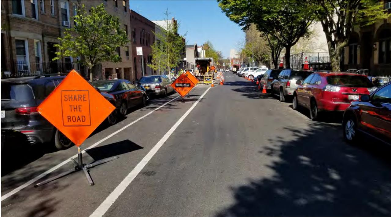
First sign is incorrectly place. It's also blocking the bike lane when it should be within the parking lane
