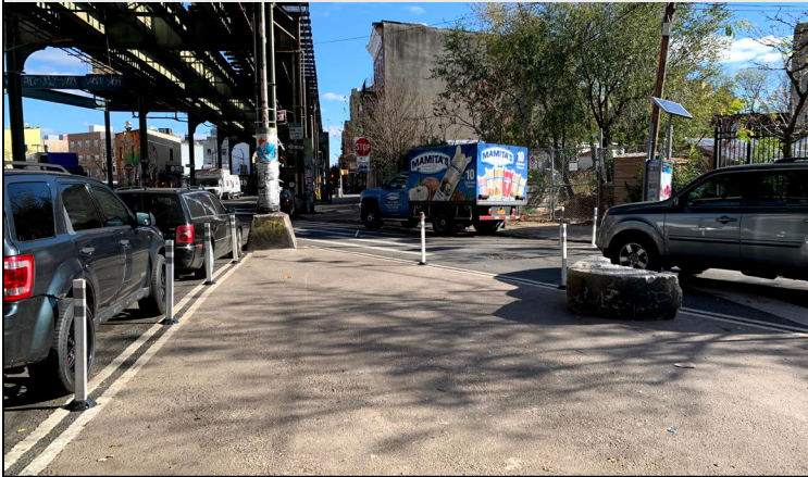
Painted Curb Extensions
