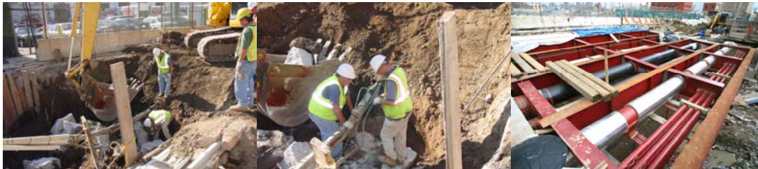
Third Avenue Bridge Under Rehabilitation in September 2007 and February 2008.
