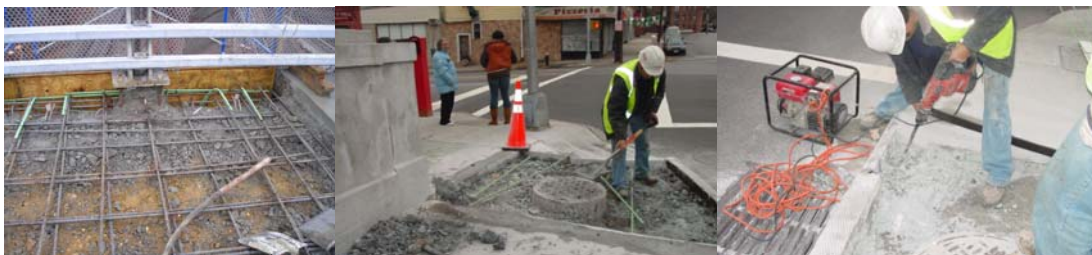
East 238 th Street: North Sidewalk Repairs in 2007. Sidewalk Repairs in 2008.
