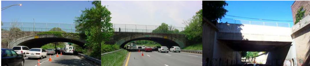
Merrick Boulevard Bridges over Laurelton Parkway (NB and SB), 149 th Street Bridge over LIRR. (Credit: NYSDOT)
