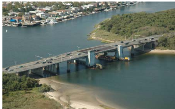
Aerial View of the Belt Parkway Over Mill Basin Bridge.
