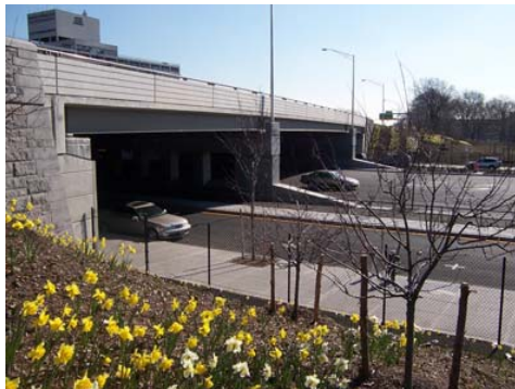
Belt Parkway Bridge in Spring 2005.
