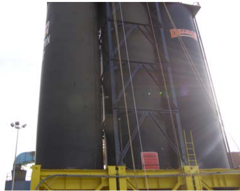
The Completed Project. (Credit: Earlene Powell)
