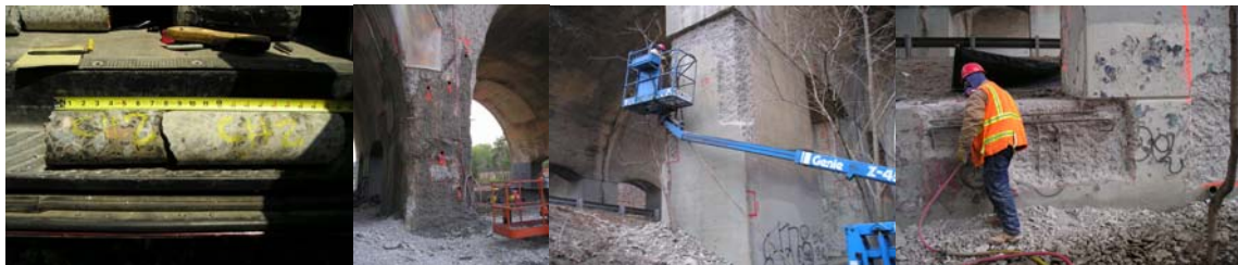
East 238 th Street: Coring at Pier #9 in 2006. Underdeck at Span #3 in 2006.
