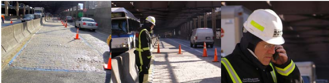
Waterproof Membrane on the Approach. Executive Director of Bridge Preventive Maintenance and Repair Thomas Whitehouse Inspecting the Work. (Credit: Clara Medina)
