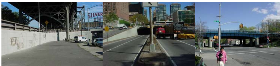
Queensboro Bridge Ramp over 11th Street & Terrain, Approach to United Nations Plaza – 1st Avenue Tunnel, Belt Parkway Bridge over Ocean Avenue. (Credit: NYSDOT)
