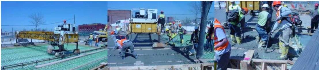
Deck Slab Concrete Pour at the Third Avenue Bridge in April 2008.
