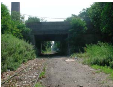
Ocean Avenue Bridge over LIRR Bay Ridge. (Credit: NYSDOT)
