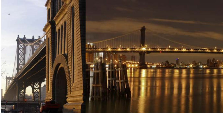
Manhattan Bridge. (Credit: Bojidar Yanev) Bridge at Night in May 2008. (Credit: Jason Bax)
