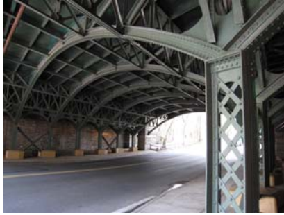
Riverside Drive Bridge in Spring 2008. (Credit: Russell Holcomb)
