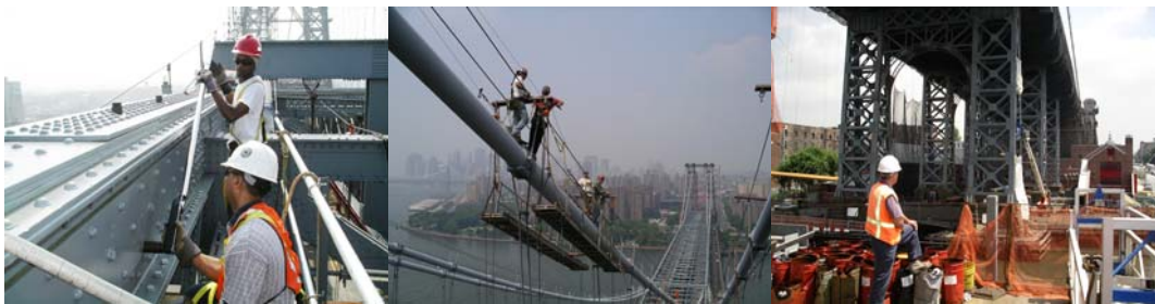
Contract #8 in 2004: High Strength Bolt Torque Inspection. Cable Band Bolt Retensioning. Steel Bracing Replacement Operation at the Brooklyn Intermediate Towers.
