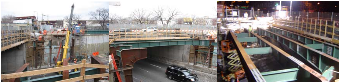
Installation of South Steinway Street Bridge Steel Frame Posts and Steel Erection in March 2007.
