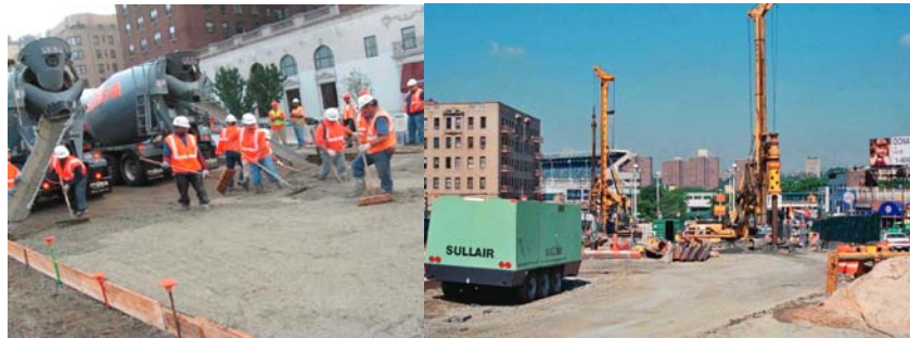
Pouring Concrete for Pavement. Rigs in Lou Gehrig Plaza Drilling and Installing Cantilever Soldier Piles.
