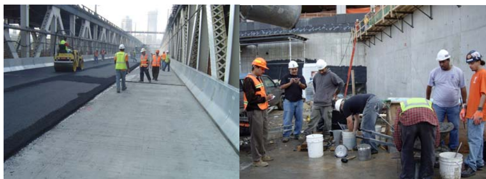
Quality Assurance Engineers Yuliy Zak and Javed Sarwar Inspecting the Asphalt and Concrete on the Manhattan Approach of the Manhattan Bridge. (Credit: Masroor Mahmood) Quality Assurance Engineer Masroor Mahmood Inspecting the Concrete for the West Abutment Wall of the New 63 rd Street Bridge. (Credit: Yuliy Zak)
