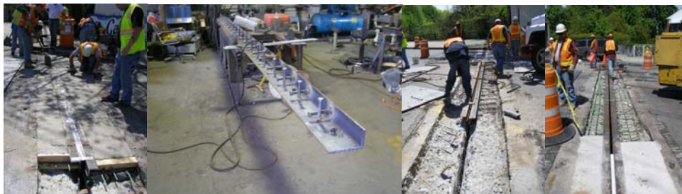
Newly Poured Eastchester Bridge Concrete Header Joint. Preparing the Steel. Installing New Steel Joint Angles. New Reinforcement.
