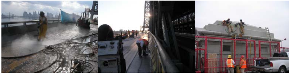
Contract #8 in 2006: Water Blasting. Curb Angle Cleanup and Tack Coat. Core Drilling The Brooklyn North Comfort Station.
