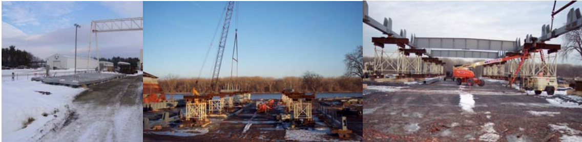
2005: Precast Deck Units for the 145 th Street Bridge at the Fabrication Facility. Placing the Bottom Chord of the Swing Span on the Supporting Towers.
