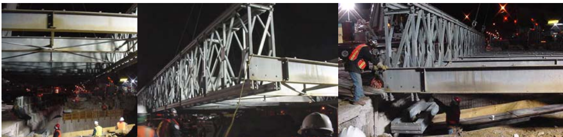
2004: Erection of the North Steinway Street Temporary Bridge.
