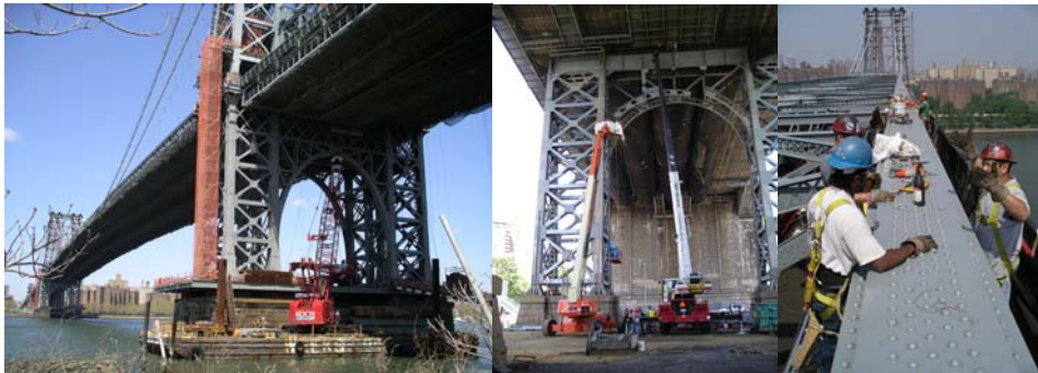
Contract #8 in 2004: Pier Stationed & Barge Mounted Cranes at Brooklyn Main Tower Pier. Steel Arch Replacement. Looking West at the North Truss Top Chord Steel Rehabilitation.
