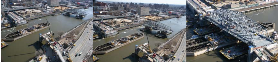
Floating In the New 145 th Street Span in February 2007.
