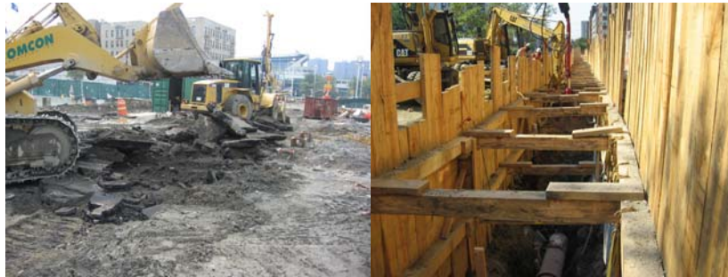
2006: Removing Asphalt and Concrete Roadway. Installing Sewer Between East 165 th and East 166 th Streets.
