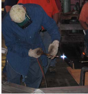
Bridge Repairer and Riveter David Collins Demonstrating Heat Straightening Techniques. (Credit: George Klein)
