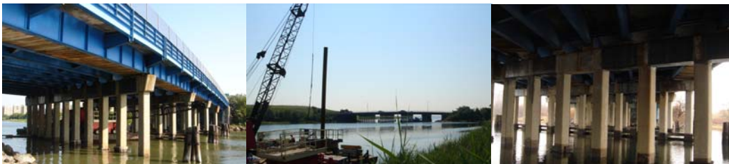
Finishing the Fiber Wrapping of the Four Piers. Removing the Scaffolding and Other Materials from the Bridge Site. View of Rehabilitated Cap Beams.
