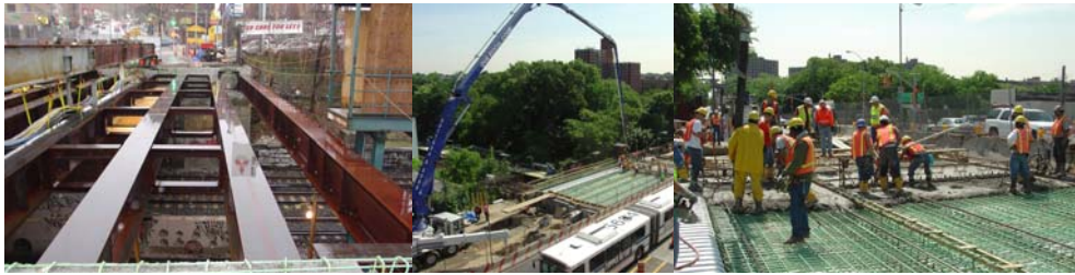
April 2007: Looking West – Gun Hill Road Bridge Stage III Girders and Temporary Support for Existing ECS Cables. June 2007: Using a Pump to Place Stage III Bridge Deck Concrete.
