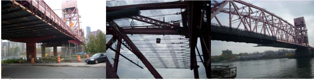
Construction of the Below Deck Shield for the Queens Approach of the Roosevelt Island Bridge. Above Deck Containment on the Lift Span. The Lift Span Shield Looking Northeast.
