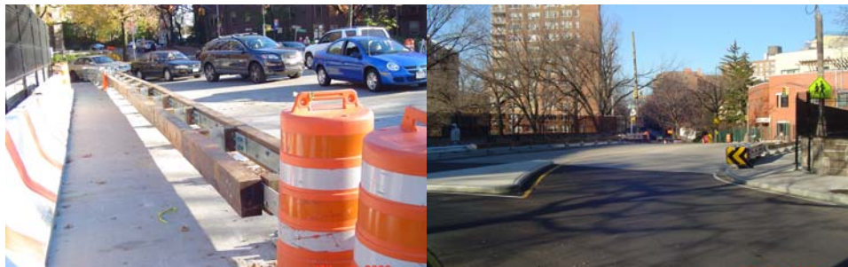
Newly Installed Steel-Backed Timber Guide Rail at West 239 th Street Bridge. Completed Bridge.
