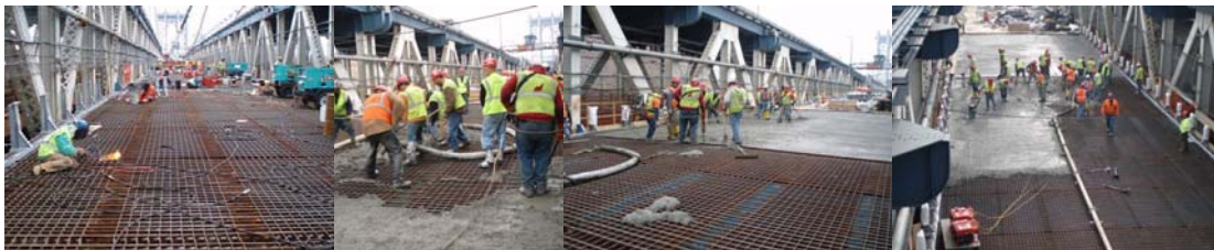
Contract #11 in 2006: Installation of Full Width Grid Deck Panels. Lower Roadway Grid Deck Concrete Pour in December 2006.
