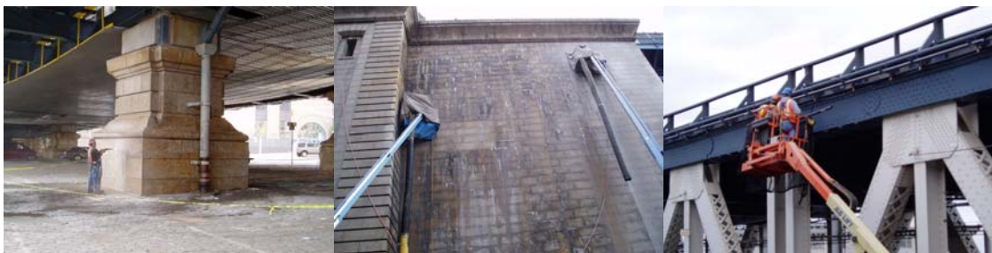
Contract #11 in 2005: Masonry Cleaning of the Brooklyn Granite Pier and of the North Face of the Brooklyn Anchorage. Installing Conduit for the New North Upper Roadway Street Lighting.
