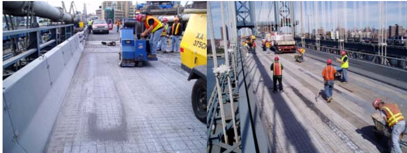
Contract #11 in 2005: Preparing the Deck for New Microsurfacing on the South Upper Roadway.
