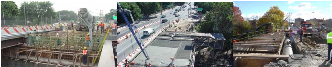
July 2006: Looking East - Placing Concrete for The Gun Hill Road Bridge East Abutment Backwall, and a Quality Assurance Engineer Inspecting the Work. September 2006: Stage 2 Construction Zone, Placing Concrete for the Deck. November 2006: Looking East - Removing the Existing Water Main Pipe on the Bridge.
