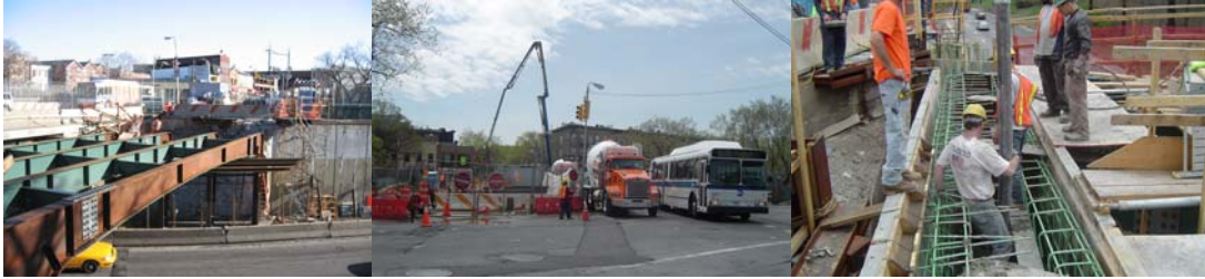
Installed Steinway Street Bridge Diaphragms in March 2007. Concrete Placement at the North Abutment of the South Bridge.
