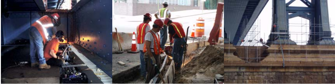
Contract #11 in 2006: Ironworkers Removing Existing Rivets in Preparation for Replacement of Lower Roadway. Installing Steel-Faced Curb for Sands Street Realignment. Erecting Scaffold to Build Painting Containment at Base of Brooklyn Tower.
