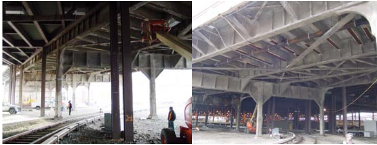
Removing Loose Overhead Concrete at the Staten Island Ferry Terminal Bus Ramps.
