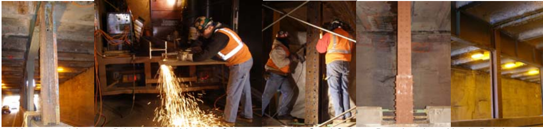
Hempstead Avenue Bridge Repairing the Column. Existing Steel Column Deterioration. Newly Reinforced Column. General View of the Repaired Area.
