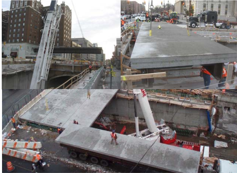
2006: Installing the Precast Panels.
