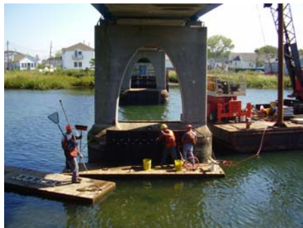
Starting the New Timber Fender Protection for Pier 6 of the 163 rd Street Bridge.
