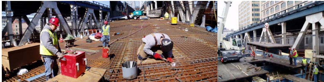
Contract #11 in 2007: Bending a Reinforcing Bar for the New Lower Roadway Grid Deck. Welding of the New Lower Roadway Grid Deck. Removal of the Existing Lower Roadway Grid Deck and Stringers on the Brooklyn Approach Span.
