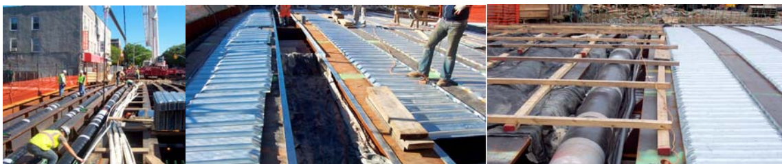
Installing the Gas Main Under the 20 th Avenue Bridge North Sidewalk in September 2007. Installing Metal Forms for the Bridge Deck in November 2007. Gas Mains Prior to Modification in December 2007.
