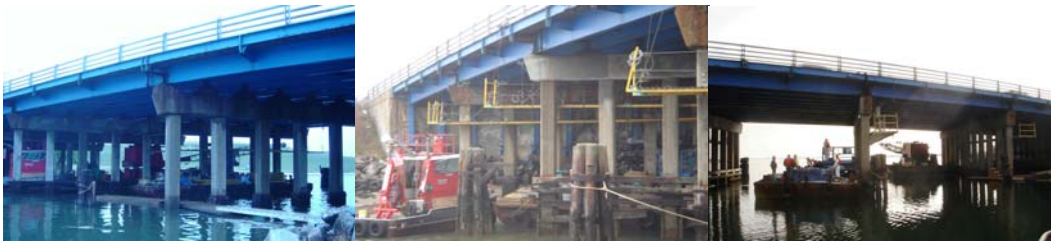
Working Under the Bridge at Low Tide. Scaffolding System Utilized to Work on the Concrete Pier Structures.
