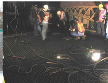
Bridge Operator Mary Harrigan at the Union Street Bridge. (Credit: Adal Maldonado) Bridge Repairer/Riveters Repairing the Willis Avenue Bridge Grating. (Credit: Reza Taheri)
