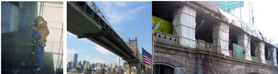
Abrasive Blasting. Platform Installed for Painting of the Queensboro Bridge (Credit: Vadim Sokolovsky) Containment on Queensboro Bridge Manhattan Ramp. (Credit: Peter Basich)
