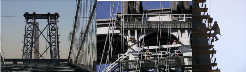
Contract #8 in 2004: Looking East at the Brooklyn Main Tower Temporary Work Platforms. Manhattan Main Tower Temporary Platform Erection. Strengthening Plate Operation on Brooklyn Main Tower.
