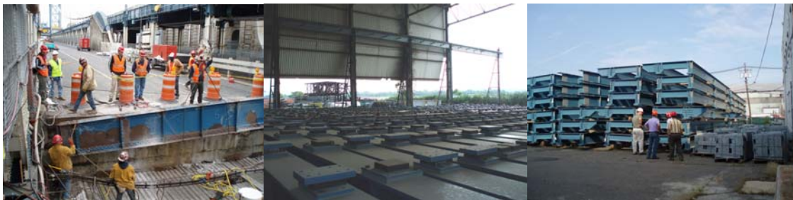
Contract #11 in 2006: Removal of First Floorbeam for Lower Roadway Reconstruction. The Fabricated Steel, Complete With Bearings, In The Contractor's Storage Yard.
