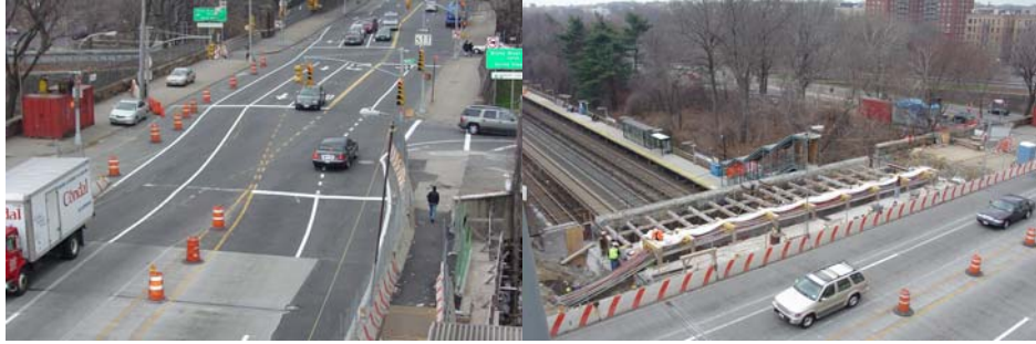
Gun Hill Road Bridge in December 2006: Looking East at the Stage III Traffic Shift, and Looking Northeast at Laborers Securing Plastic Covers on ECS Cables.
