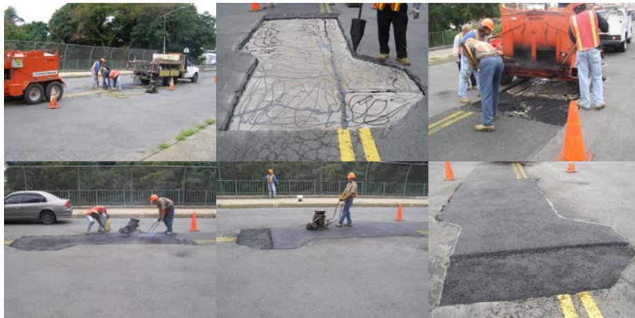
Repairing the Center Roadway Asphalt Overlay of the 14 th Avenue Bridge.
