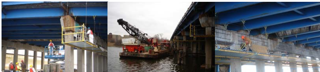
Reinforcing the Newly Restored Fresh Creek Bridge Concrete Pier Structure With Fiber Wrapping. Positioning the Barge Between the Piers. Removing and Repairing the Concrete for Each Pier.
