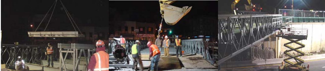
2004: Erection of the South Steinway Street Temporary Bridge.
