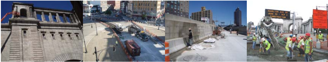
Contract #11 in 2007: Masonry Cleaning of the Upper Section of the South Face of the Manhattan Anchorage. Milling of the Existing Lower Roadway Pavement at the Manhattan Plaza. Masonry Cleaning of the Lower Roadway Wall at the Brooklyn Transition. Concrete Placement in Manhattan Plaza at the Entrance to the Lower Roadway.
