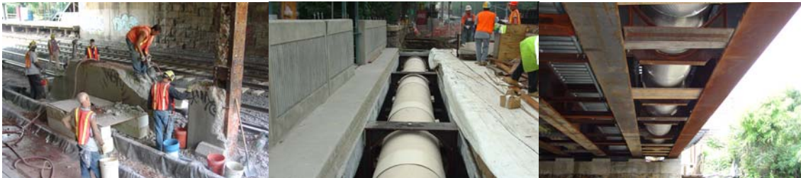
Gun Hill Road Bridge in June 2007: Looking Southwest at Laborers Demolishing the Existing Center Pier. July and August 2007: Installing a New Water Main.
