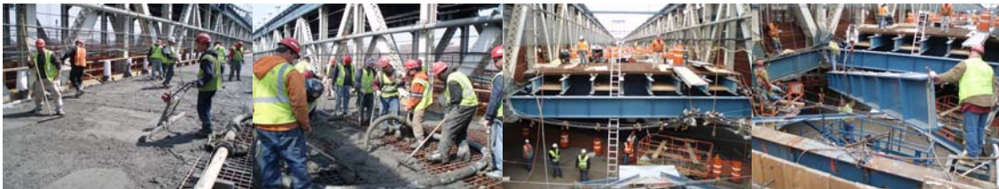
Contract #11 in 2007: Concrete Placement in the New Lower Roadway Grid Deck on the Main Span. New Lower Roadway Floorbeams, Stringers and Grid Deck on the Brooklyn Approach Span.
