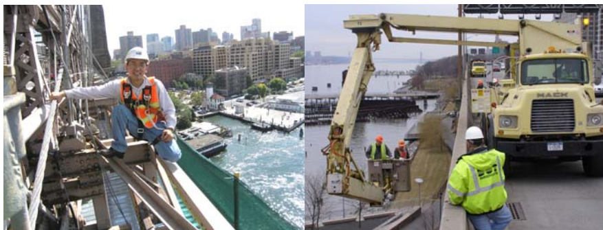
Assistant Civil Engineer Andrew Hoang Inspecting the Brooklyn Bridge. (Credit: Clara Medina) Snooper Truck Utilized in March 2007 During an Emergency Inspection of the Northbound Henry Hudson Parkway.
