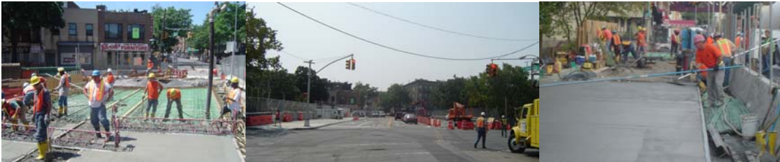
Deck Placement on the Steinway Street One-Third structure in June 2007. Shifting Traffic to the Eastern Side of the Bridges. Concrete Placement for the West Sidewalk in October 2007.
