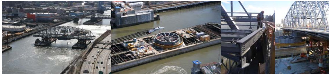
Floating In the New 145th Street Span in February 2007. (Close-up Credit: Bojidar Yaney)
