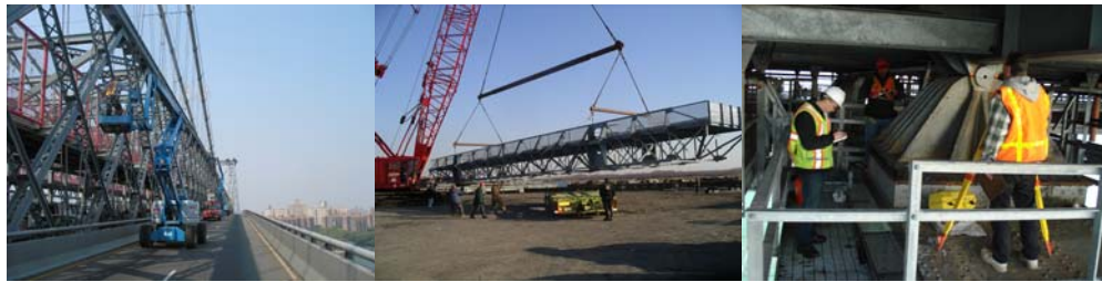
Contract #8 in 2006: Touchup Painting on the North Truss. First Traveler Platform. Bearing Survey.
