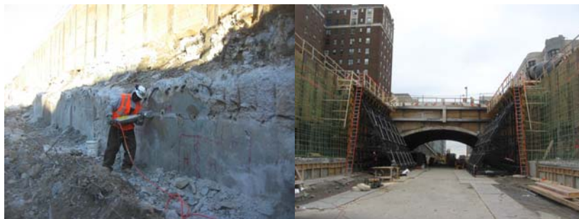
2006: Removing Concrete at the Springline of the South Abutment Stem. Formwork and Concrete Placement at South Abutment.
