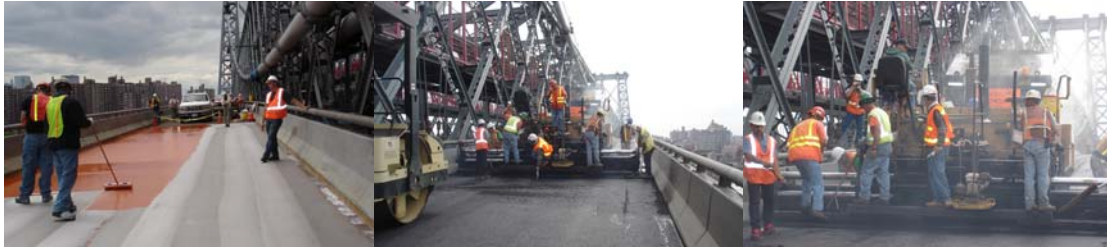
Contract #8 in 2006: Priming Application and Asphalt Paving Operation on the South Outer Roadway.
