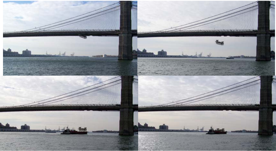
Removing the Brooklyn Bridge Main Span Travelers.
