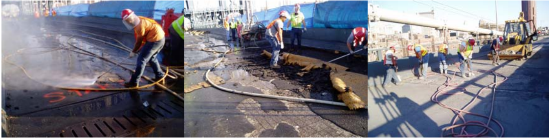
Contract #11 in 2005: Waterblasting to Remove Existing Microsurfacing From the South Upper Roadway. Manually Removing the Microsurfacing.
