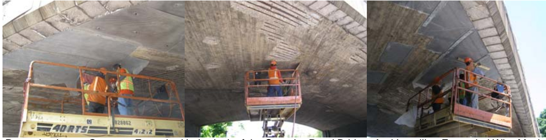
Removing Loose Concrete From the Underdeck of the Superior Road Bridge, And Installing Expanded Wire Mesh.
