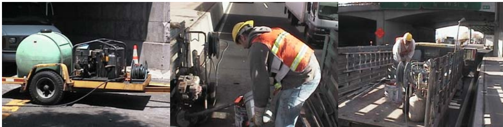
Pressure Washing Machine Used for Graffiti Removal. It is Set to 2500 psi and 212° F. Bridge Painters Frank Duic and Russell Newme Feeding the Spray Pump and Preparing the Paint.
