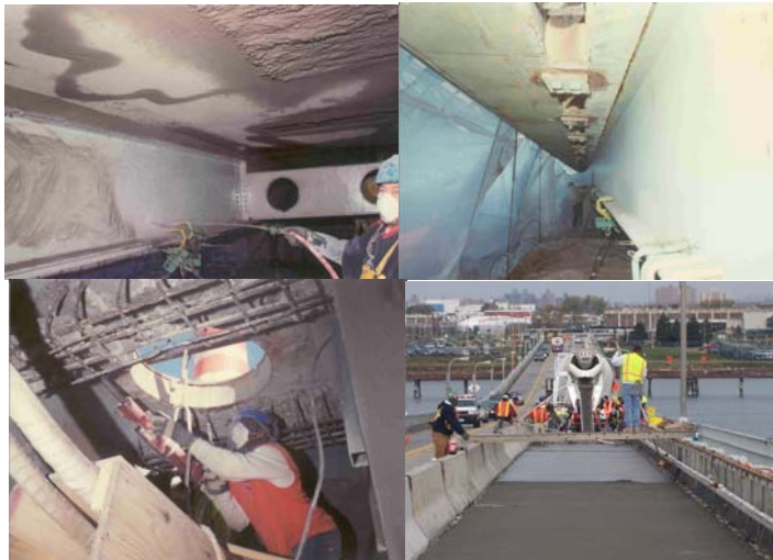
2006: Performing Underdeck Repairs. Working Inside the West Rebar Box Frame. Beam Repair. Concrete Placement.
