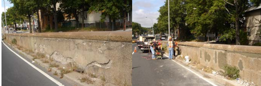
Missing Grout on the Woodhaven Boulevard Bridge Parapet Wall. Repairing the Grout.
