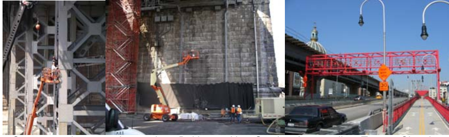
Contract #8 in 2004: Ironworkers Bolting up New Steel on Intermediate Tower. Cleaning the Brooklyn Anchorage Exterior Granite Surface. Entrance to North Walkway. (Walkway Credit: Peter Basich)
