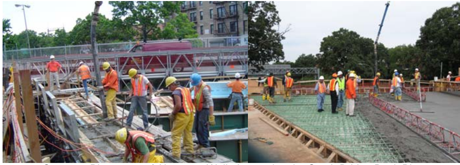
2006: Concrete Placement of Abutment Wall. Inspecting the South Bridge Deck Placement.
