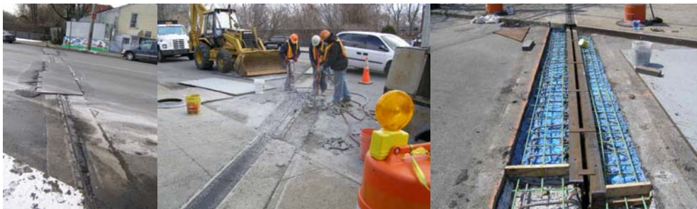
Existing Eastchester Road Bridge Joint Condition Covered With Roadway Plates. Removal of Existing Concrete Header. Newly Installed Concrete Header Reinforcement.
