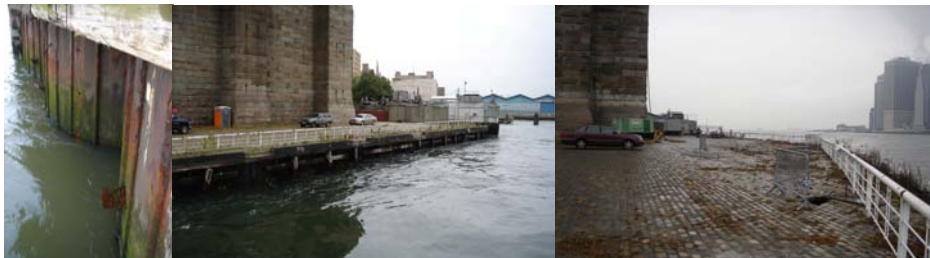
Holes in the Steel Sheet Cofferdam of the Brooklyn Bridge Esplanade. View of the Work Area. View of the Pavers Before Work Began to Stabilize the Area.
