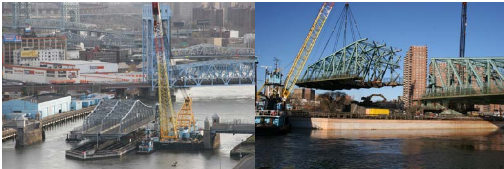
2006: Barge Carrying Crane Passing The Open Madison Avenue Bridge on the Way to Dismantle the Old 145 th Street Swing Span. Dismantling the Truss.
