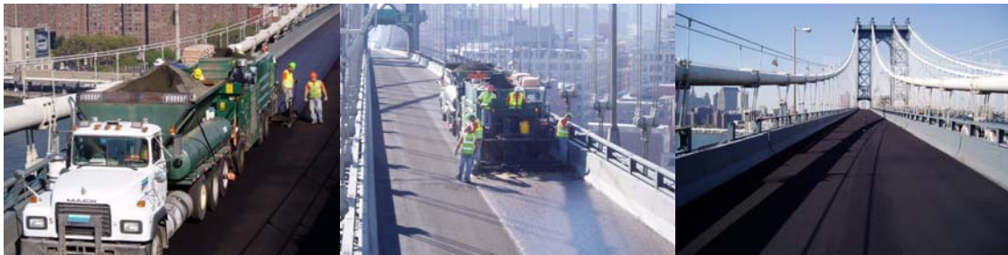
Contract #11 in 2005: Placing the New Microsurfacing on the South Upper Roadway. Newly Resurfaced Roadway.
