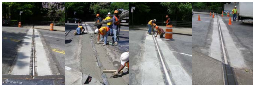
Eastchester Bridge Concrete Header and Steel Joint Angle Prior to Rubber Seal. Pouring Concrete for the New Joint Headers. Installing the Seal. Completed Project.
