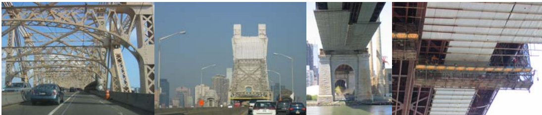
Protective Coating in 2005: Newly Painted Section Along the Upper Roadway. Containment on the Queens Side Tower. (Credit: Peter Basich) Queensboro Bridge Work Platform. Painters Arriving at the Platform. (Credit: Michele N. Vulcan)
