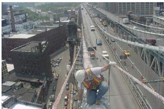
Inspector on Manhattan Bridge Cable. (Credit: NYSDOT)
