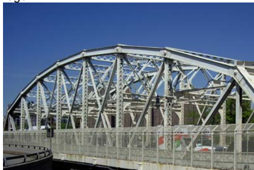
Macombs Dam Camelback Truss.
