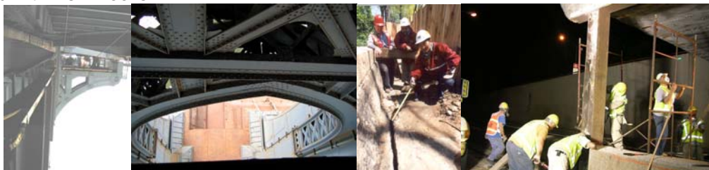
Flag Engineers Inspecting a Red Flag (Floor Beam Web) on the Tower Structure of the Manhattan Bridge. Closeup of the Location. (Credit: Bojidar Yanev) Flag Engineers Inspecting a Red Flag on the Central Drive Bridge over Transverse Road #1-- the West Fascia Had a Long Crack Running From the South Abutment Wall to the North Abutment Wall. (Credit: Peter Basich) Red Flag Repairs at the Houston Street Bridge over the FDR Drive. (Credit: Hany Soliman)
