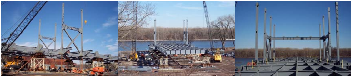
2006: Assembling the New 145 th Street Bridge Swing Span in Albany.
