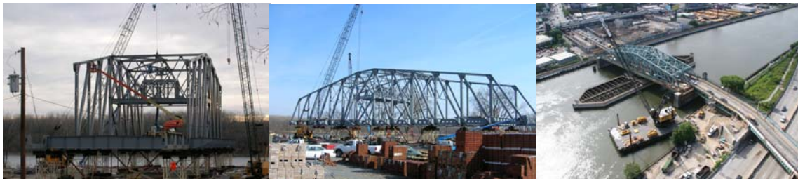
2006: Continued Assembly of the New 145 th Street Bridge Swing Span. Removing Steel Girders Over the Harlem River Drive.
