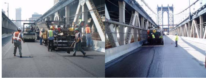
Contract #11 in 2007: Placement of New Asphalt on the Lower Roadway at the Brooklyn Approach Span. Placement of New Microsurfacing on the Lower Roadway at the Manhattan Side Span.
