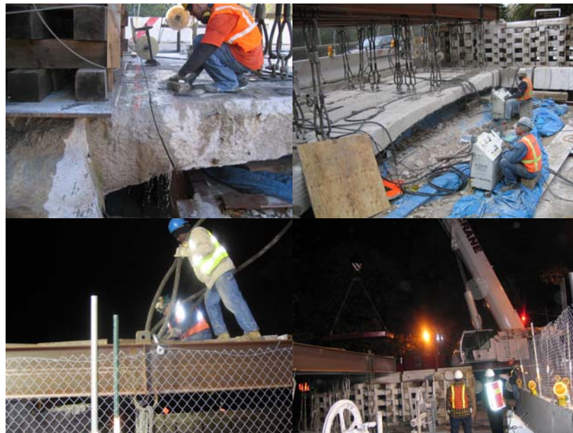
2006: Wire Sawing the Deck and Removing the Existing West 252 nd Street Bridge Sections Over the Parkway.
