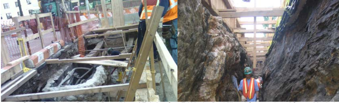
2006: Grand Concourse Bridge: Demolition of Existing Con Ed Vault. Backfill and Compaction of Sewer Manhole.
