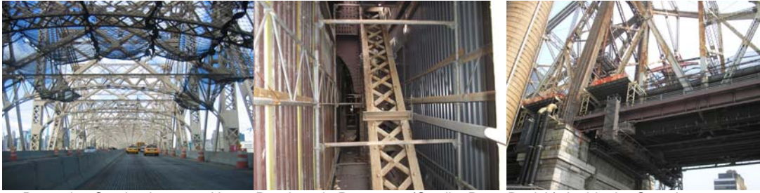
Protective Coating in 2006: Upper Roadway in Progress. (Credit: Peter Basich) Inside the Containment on the North Side of the Inner Roadway. Installed Platform Above South Outer Roadway.
