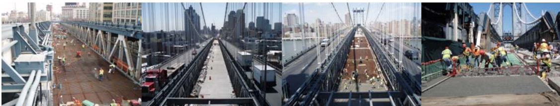
Contract #11 in 2007: The New Lower Roadway Grid Deck on the Brooklyn Approach Span. The New Lower Roadway on the Brooklyn Side Span After Concrete Placement. New Lower Roadway Concrete Placement on the Brooklyn Main Span, and at the Brooklyn Anchorage.
