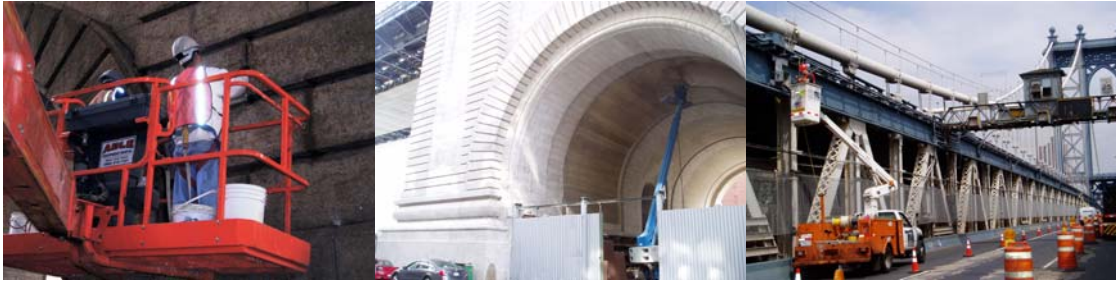
Contract #11 in 2006: Pointing Joints on East Face of Brooklyn Anchorage. Masonry Cleaning Inside Archway of Brooklyn Anchorage. Installing Conduit and Wire for New Lower Roadway Lighting.
