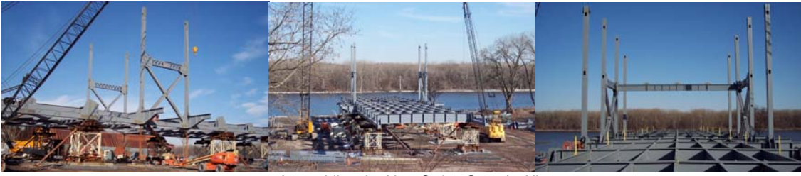
2006: Assembling the New Swing Span in Albany.
