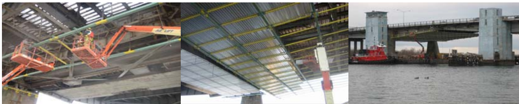
Installing the Hangers, Tubes, and Decking of the Underdeck Shielding. Marine Work.
