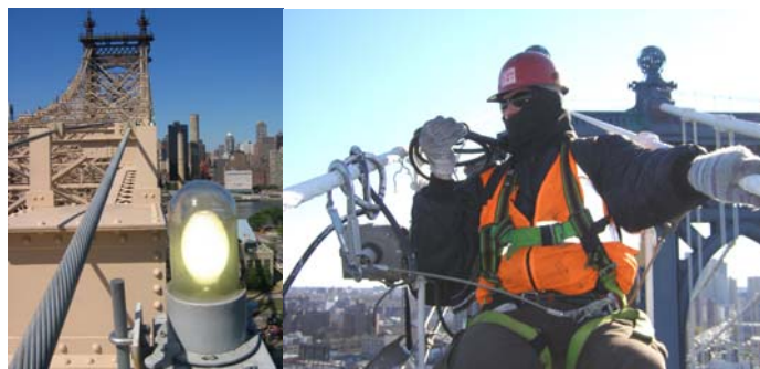
A Bulb of the Queensboro Bridge Necklace Lights. (Credit: Peter Basich) Repairing a Manhattan Bridge Necklace Light. (Credit: Hany Soliman)
