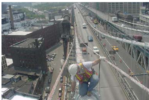
Inspector on Manhattan Bridge Cable. (Credit: NYSDOT)
