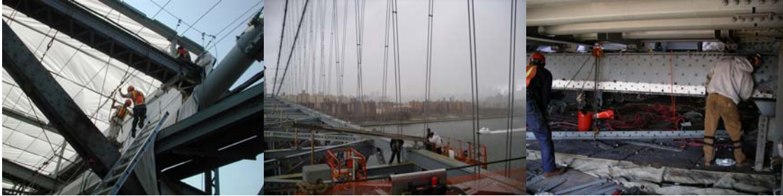
Contract #8 in 2003: North Stiffening Truss Containment Erection and Removal. South Truss Bottom Chord Rehabilitation.
