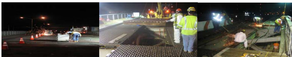
Sawcutting And Removing Deck Panels. Surface Preparation After Panel Removal.
