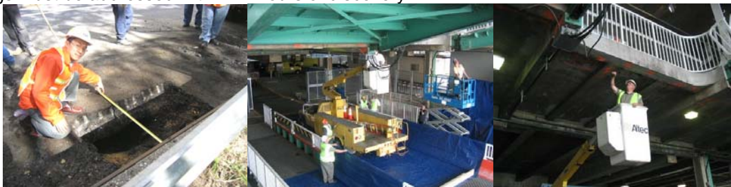
Assistant Civil Engineer Andrew Hoang Measuring a Safety PIA Flag Condition (a Sinkhole in A Ramp's Roadway Slab) After the Removal of Delaminated Concrete But Before Repairs Begin. Executive Director of Bridge Preventive Maintenance and Repair Tom Whitehouse (White Hardhat) Ensuring the Proper Setup of Containment Procedures at the St. George Ferry Terminal Landing Slips Before the Masons Address A PIA Flag (Falling Concrete). Inspecting the Flagged Condition.
