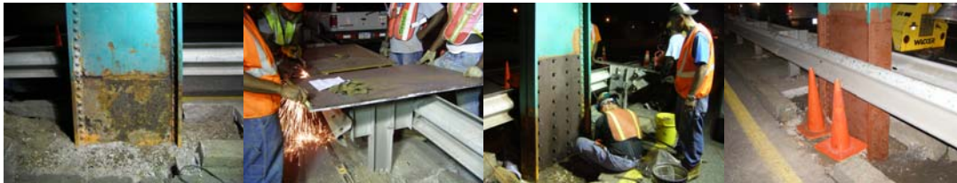
Nighttime Installation of Steel Column Web Reinforcement at the East 111 th Street Pedestrian Bridge Over the FDR Drive. Completed Repair.
