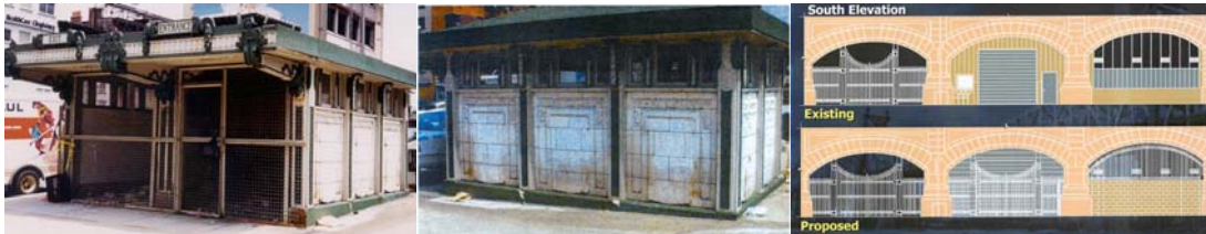
Views of the Queensboro Plaza Kiosk. Proposed Rehabilitation of the Arch Infill for the Sanitation Department.
