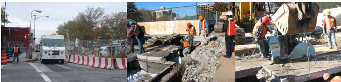
Old Congress Street Bridge. Bridge Deck Demolition. (Demolition Credit: Carlos Ramirez)
