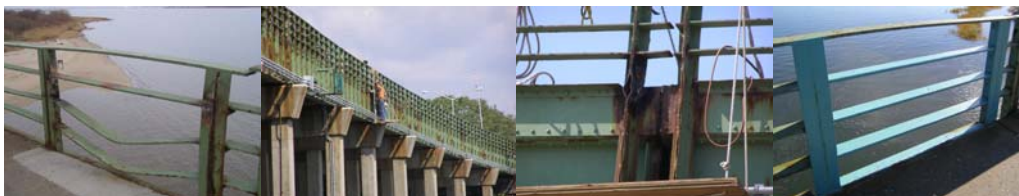
Repairing the Railings at the Belt Parkway Bridge Over Paerdegat Basin. Completed Repairs.
