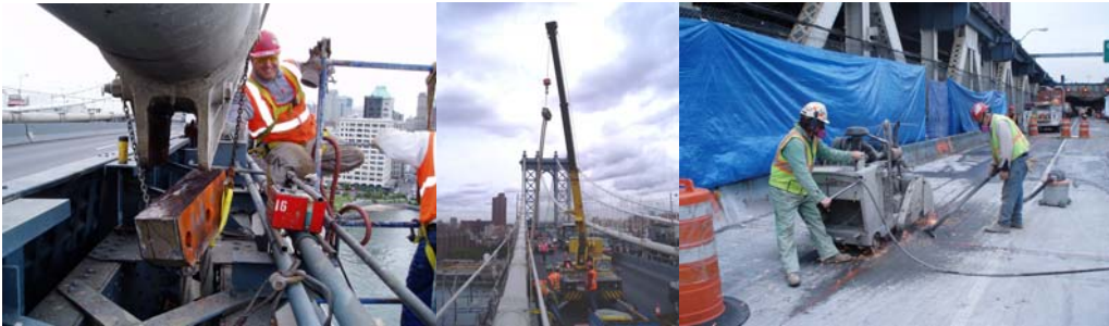
Contract #11 in 2006: Removal of Existing Suspender Rope From Cable Band on Main Span. Sawcutting Lower Roadway Deck on Manhattan Approach Span.
