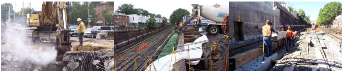
Demolition of the 17 th Avenue Bridge Deck. Casting the New East Abutment Wall. Installing Precast Concrete Footings.
