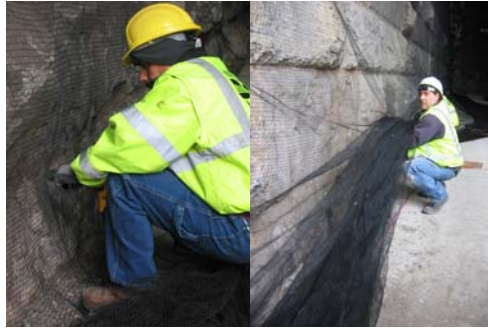
Installing Pigeon Proofing at the Anti-Icing Platform. (Credit: Peter Basich)
