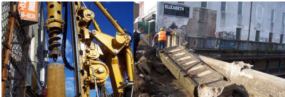
Removing The 20 th Avenue Bridge Arch Overburden.
