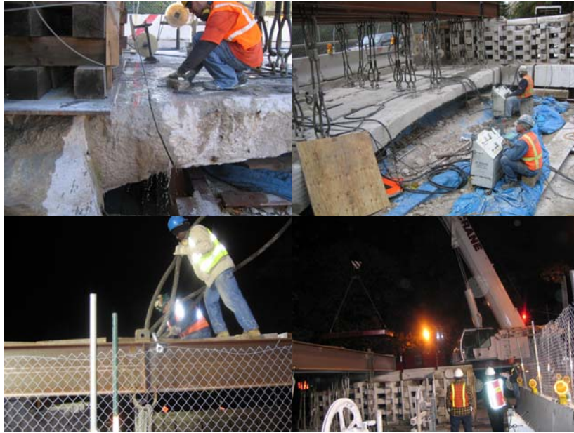
Wire Sawing the Deck and Removing the Existing Bridge Sections Over the Parkway.
