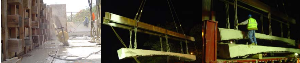
Cutting and Removing the Existing Bridge Sections Over the Parkway.
