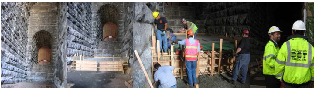
Installing an Anti-icing Tank Platform under the Brooklyn Bridge. Deputy Chief Engineer Russell Holcomb Observing The Work. (Credit: Peter Basich)
