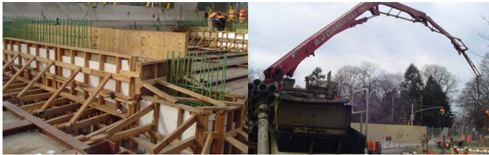
West 252 nd Street Bridge Formwork and Rebar Fabrication at the Pier and West Abutment. Concrete Placement in Progress.
