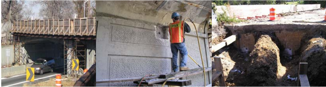
Bridge Prior to Demolition. Installing Tie Back Rods at the North Abutment of the East Bridge.
