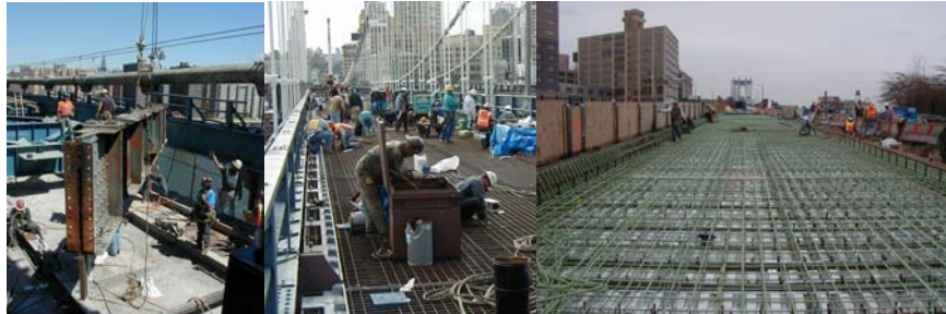
Contract #10 Removing an Existing North Upper Roadway Floorbeam on the Main Span of the Bridge. Installing the New Grid Deck for the North Upper Roadway on the Brooklyn Side Span. Preparing the Brooklyn Elevated Structure Grid Deck for Concrete Placement.
