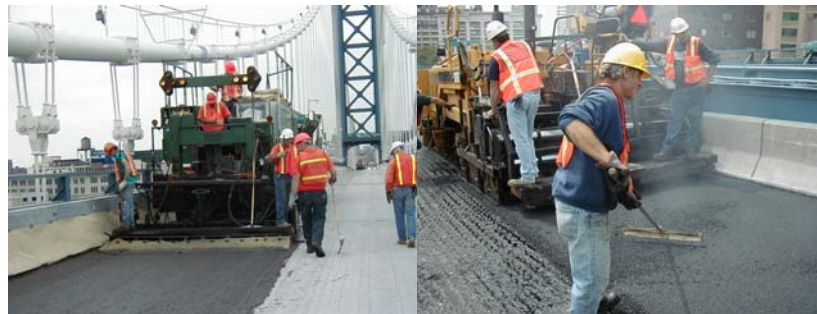
Contract #10 Placing the Microsurfacing Overlay on the Main Span. Placing the Asphalt Overlay on the Brooklyn Approach Span.
