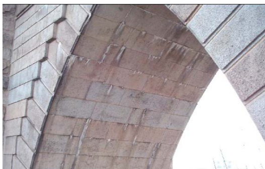
Moderate Efflorescence on the Brooklyn Bridge Brooklyn Tower North Gothic Arch in 2004. (Credit: NYSDOT)
