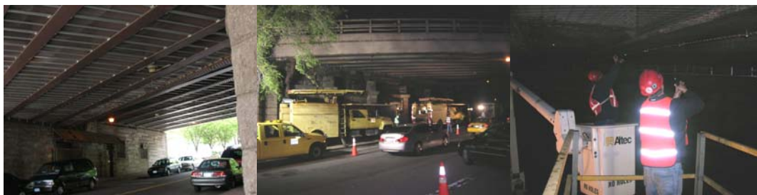
Installing Pigeon Proofing Under the Brooklyn Queens Expressway Over Prospect Street. (Credit: Joseph Vaccaro)
