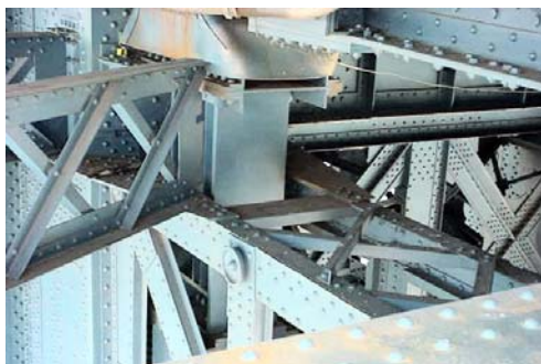
Truss Bearing on Manhattan Bridge. (Credit: NYSDOT)
