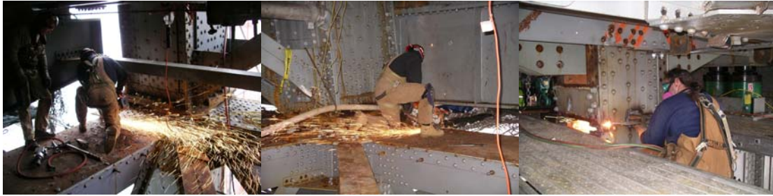
Contract #8 in 2005: Rehabilitation of the Brooklyn Main Tower Steel. Torch Cutting on the Tower.
