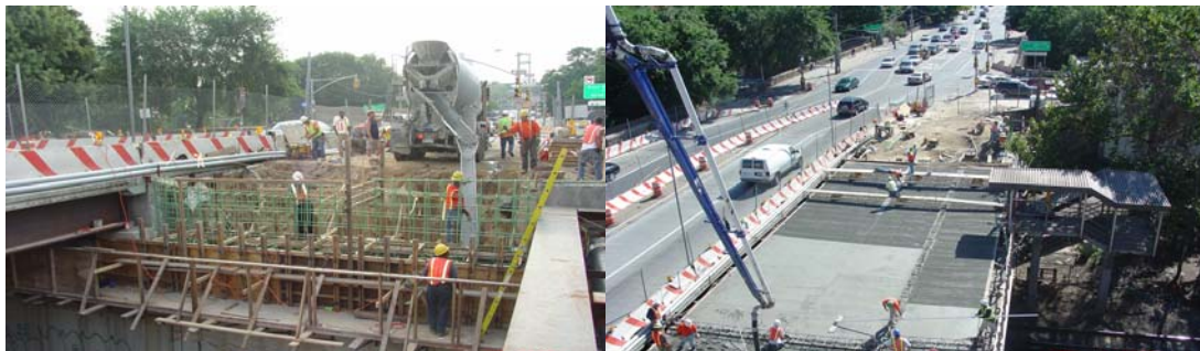
July 2006: Looking East - Placing Concrete for The east Abutment Backwall and a Quality Assurance Engineer Inspecting The Work. September 2006: Stage 2 Construction Zone, Placing Concrete for The Deck.
