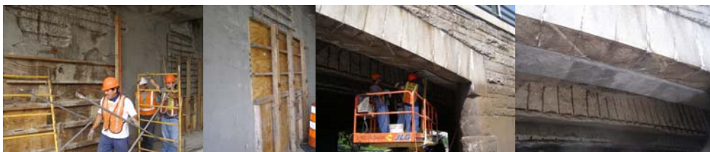
Douglaston Parkway Over Northbound Cross island Parkway: Removing Loose and Deteriorated Under-Deck Concrete, and Installing Expanded Metal Mesh.
