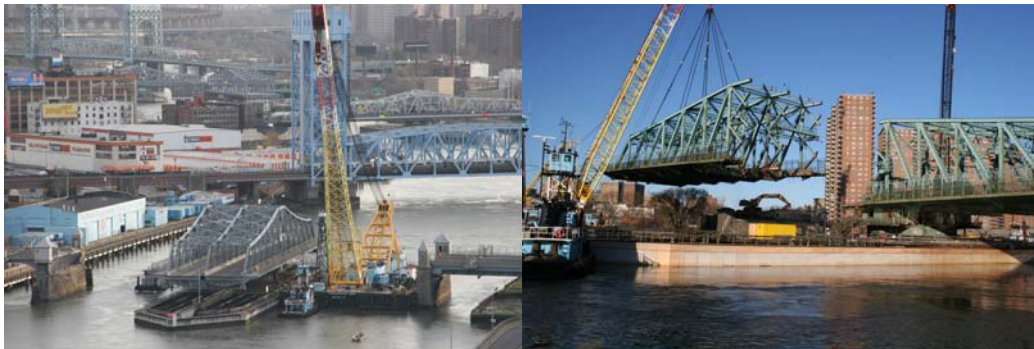
Barge Carrying Crane Passing The Open Madison Avenue Bridge on the Way to Dismantle the Old 145 th Street Swing Span. Dismantling the Truss.
