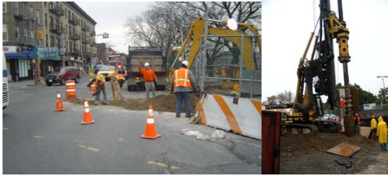
2005: Utility Workers Excavating a Trench In Order to Deactivate the Feeder Cables in the Manholes Along Steinway Street. Driving a Sleeve for the Installation of Piles at the Center Fill Area.
