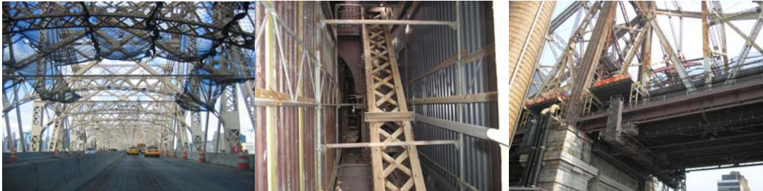
Protective Coating in 2006: Upper Roadway in Progress. (Credit: Peter Basich) Inside the Containment on the North Side of the Inner Roadway. Installed Platform Above South Outer Roadway.
