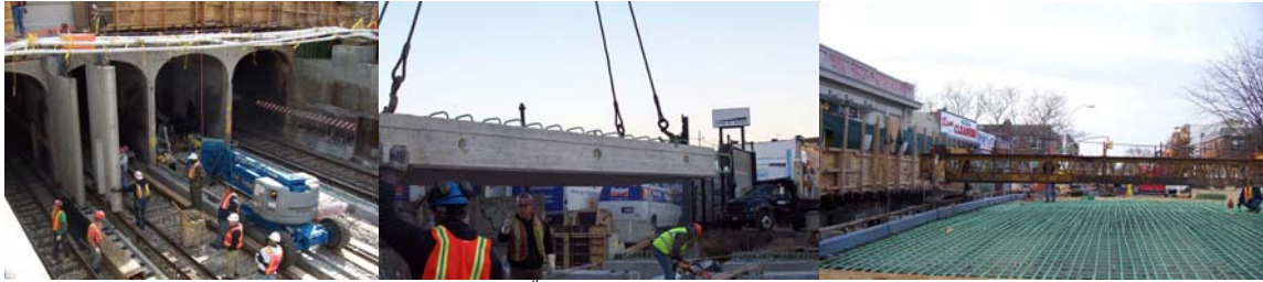
Installing Pier Walls for the 17 th Avenue Bridge. Installing Precast Deck Panels. Placing the Reinforced Concrete Bridge Deck.
