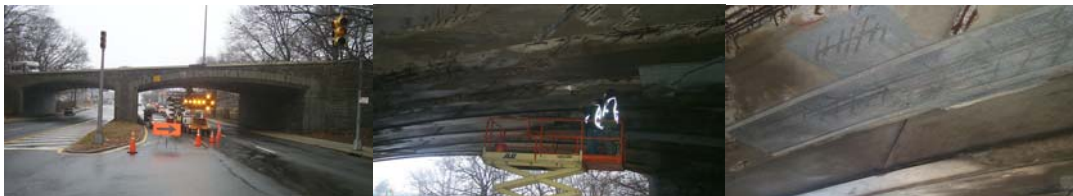
Removing Loose Concrete From the Underdeck of the Jackie Robinson Parkway Bridge Over Metropolitan Avenue, And Installing Expanded Wire Mesh.
