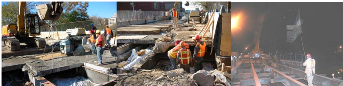
Congress Street Bridge Deck Demolition and Structural Steel Removal. (Credit: Carlos Ramirez)
