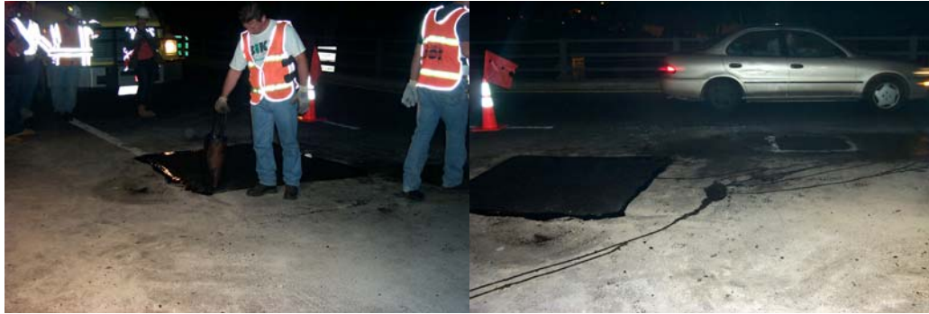
Sealing the Edges of the Cutout With Asphalt Cement to Prevent Water From Seeping In. Closeup of Part of the Completed Concrete Deck Repair on the Eastbound BQE. (Credit: Anthony Napolitano)
