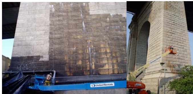
Cleaning the Masonry of the North Face of the Manhattan Bridge's Brooklyn Anchorage and of the North and East Faces of the Roosevelt Island Pier of the Queensboro Bridge.
