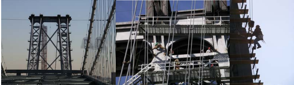
Contract #8 in 2004: Looking East at the Brooklyn Main Tower Temporary Work Platforms. Manhattan Main Tower Temporary Platform Erection. Strengthening Plate Operation on Brooklyn Main Tower.
