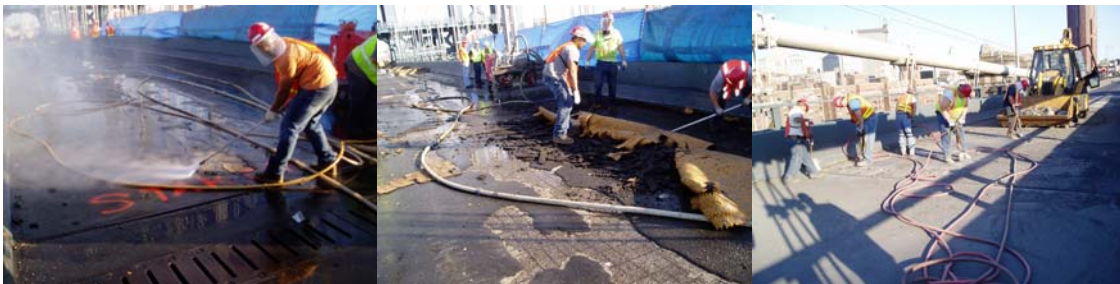
Contract #11 in 2005: Waterblasting to Remove Existing Microsurfacing From the South Upper Roadway. Manually Removing the Microsurfacing.
