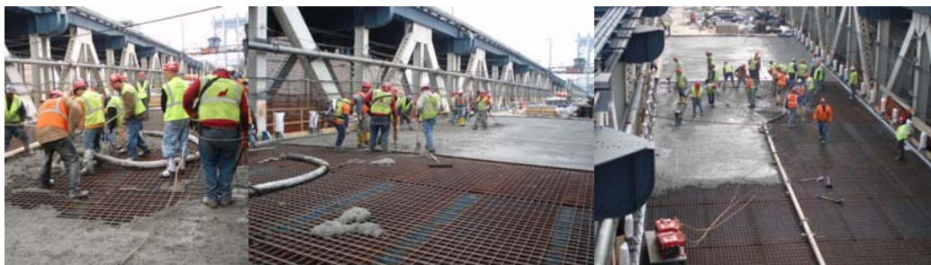
Contract #11 in 2006: Lower Roadway Grid Deck Concrete Pour in December 2006.
