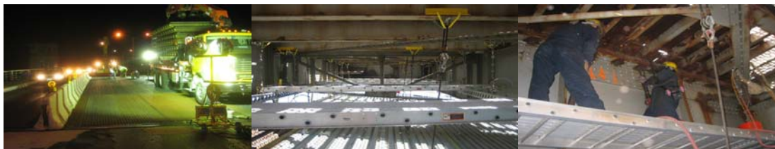
Work Zone Protection Barrier. Below Deck Access For Panel Replacement. Removing Rivets.
