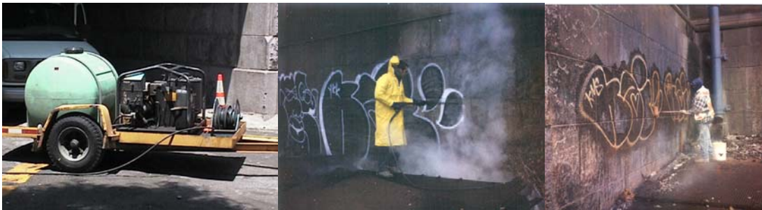
Pressure Washing Machine Used for Graffiti Removal. It is Set to 2500 psi and 212° F. Removing Graffiti From the Base of the Manhattan Bridge Facing the FDR Drive. (Manhattan Credit: Cesar Pazmino)
