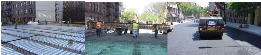
Placing Stay-in-Place Forms for The Lincoln Road Bridge Concrete Deck in March 2006. Concrete Placement for The Deck Slab in April 2006. Placing Fresh Asphalt in May 2006.
