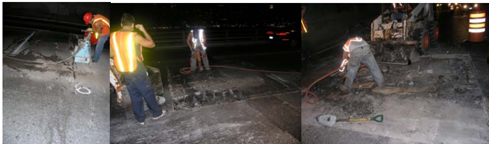
Working on The Transverse Expansion Joints.
