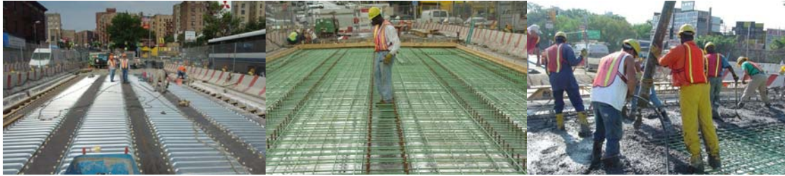
2005: Project Engineer Muhammad Siddiqui Inspecting the Stay-in-Place Formwork for the New Gun Hill Road Bridge Deck. Installing Deck Reinforcement. Concrete Placement.
