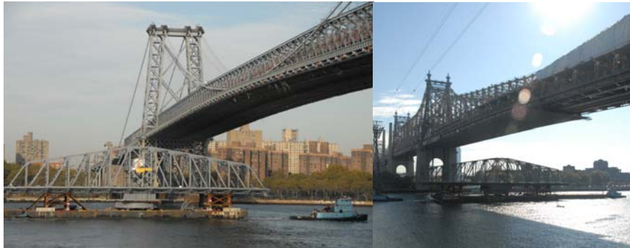
Swing Span Passing Under the Williamsburg and Queensboro Bridges. (Credit: Peter Basich)
