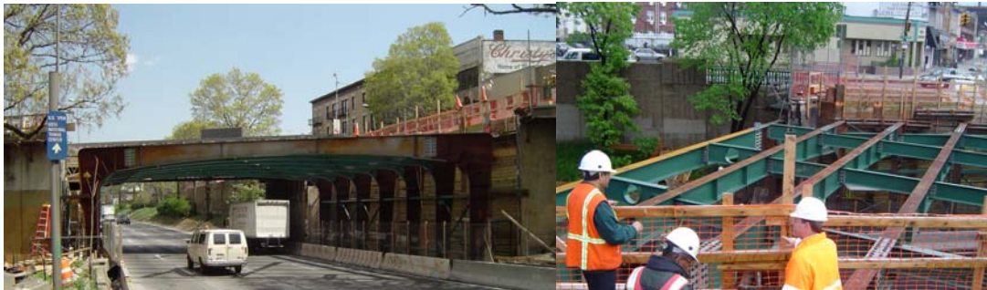
Steel Erection Over the Grand Central Parkway.
