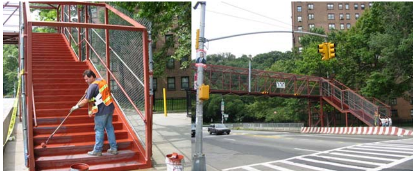
Bridge Painter Anthony Attore Painting the PS-5 Pedestrian Bridge over 10th Avenue.
