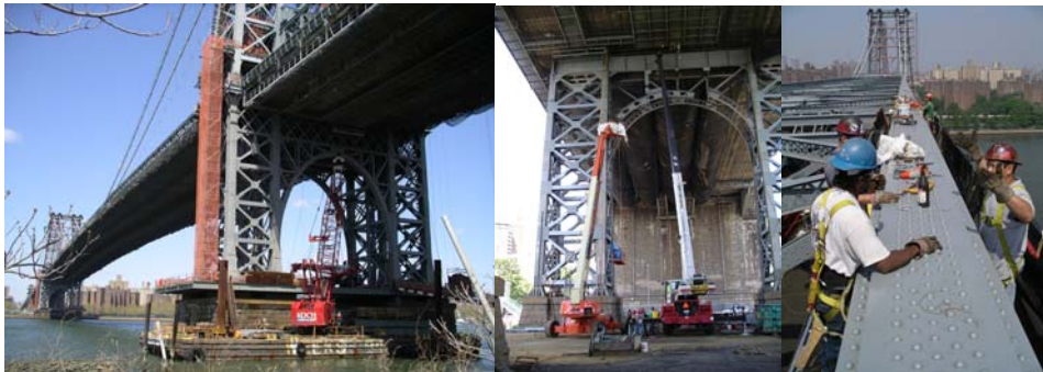
Contract #8 in 2004: Pier Stationed & Barge Mounted Cranes at Brooklyn Main Tower Pier. Steel Arch Replacement. Looking West at the North Truss Top Chord Steel Rehabilitation.
