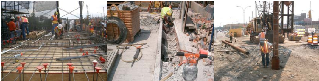
Looking East at the Rebuilding of the Operator House. Demolition of the Northwest Flanking Span of the Metropolitan Avenue Bridge. Driving Test Piles.
