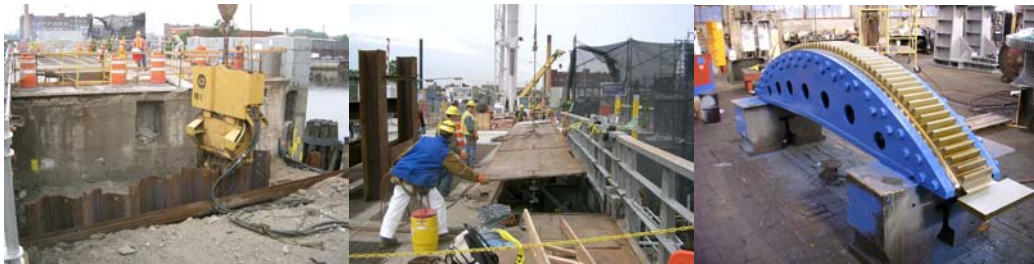
Looking West at the Installation of Sheet Piles on the Northeast Approach Slab. Looking West at the Removal of the Northwest Sidewalk. Completed New Rack Assembly in Structural Support at the Fabricator's Shop.
