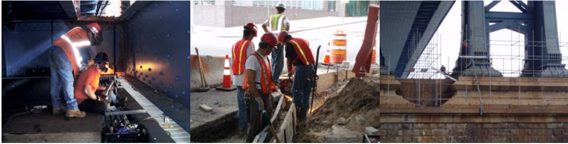
Contract #11 in 2006: Ironworkers Removing Existing Rivets in Preparation for Replacement of Lower Roadway. Installing Steel-Faced Curb for Sands Street Realignment. Erecting Scaffold to Build Painting Containment at Base of Brooklyn Tower.
