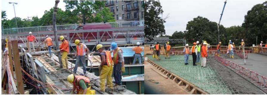
Concrete Placement of Abutment Wall. Inspecting the South Bridge Deck Placement.
