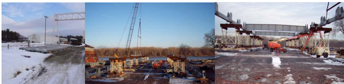
2005: Precast Deck Units at the Fabrication Facility. Placing the Bottom Chord of the Swing Span on the Supporting Towers.
