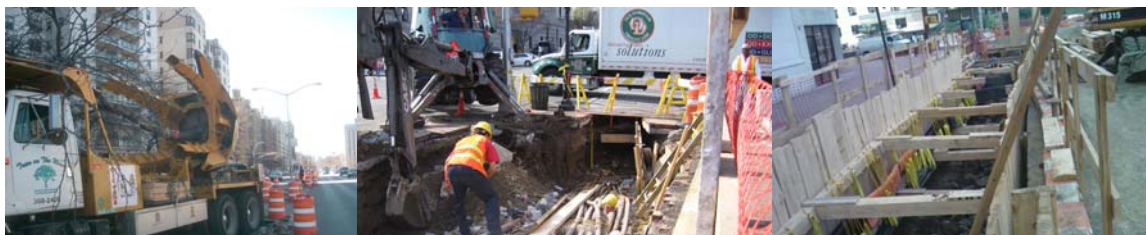
Transporting Trees From East Median for Replanting. Uncovering Live ECS Cables Above Tunnel Roof Before Bridge Demolition. Excavation for Replacement of Sewer Pipes.
