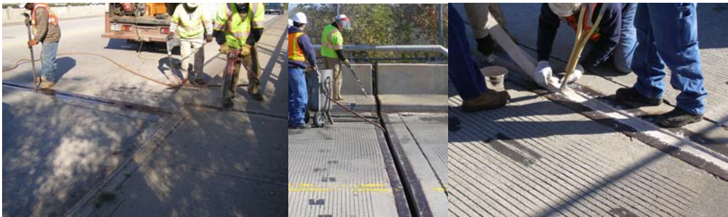
Removing Deteriorated Joint Sealer at the Page Avenue Bridge over SIRT South Shore in Preparation for its Replacement. Cleaning Steel Angle Surfaces. Installing New Joint Sealer Material.
