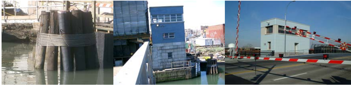
Rehabilitated Dolphins Wrapped With New Steel Cables. Old Bridge Operator House. New Bridge Operator House.
