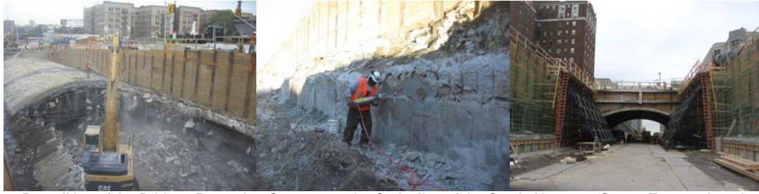
Demolition of the Bridge. Removing Concrete at the Springline of the South Abutment Stem. Formwork and Concrete Placement at South Abutment.
