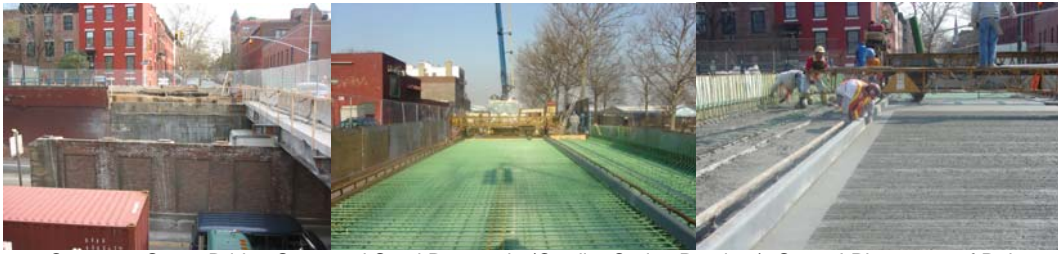
Congress Street Bridge Structural Steel Removal. (Credit: Carlos Ramirez) Stage I Placement of Rebar for Concrete. Concrete Placement for Deck Slab.
