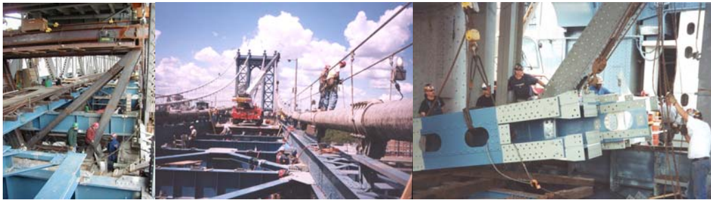
Contract #10 Temporary Truss Jacking Frame Used in the Work to Replace the Existing Truss Bearings. Replacement of Steel Stringers and Floorbeams on the North Upper Roadway Main Span. Installing a New End Frame on the Main Span Side of the Brooklyn Tower.
