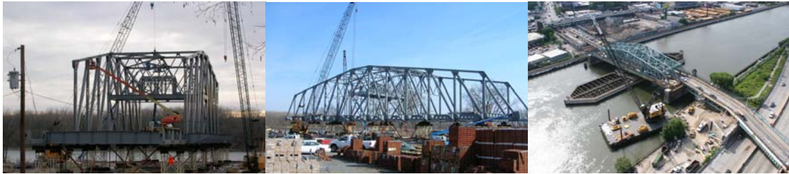
2006: Continued Assembly of the New Swing Span. Removing Steel Girders Over the Harlem River Drive.
