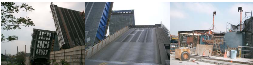
Looking West at the Open Metropolitan Avenue Bridge Before Splitting of the Leaves. Open Bridge With Split Leaves. Looking North at the Demolition of the Bridge Operator House.
