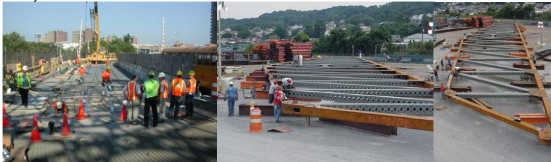
2005: Replacing Span #3. Swing Span Truss Assembly.
