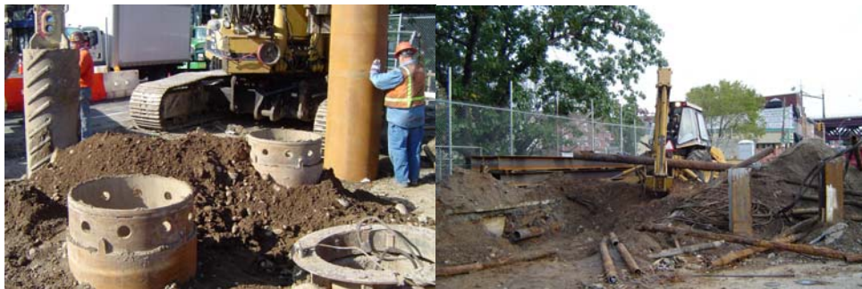
2005: Preparing to Install Piles at the Southern End of the South Bridge. Removing the Utility Conduit Pipes From the Western Side of the Steinway Street Bridges.
