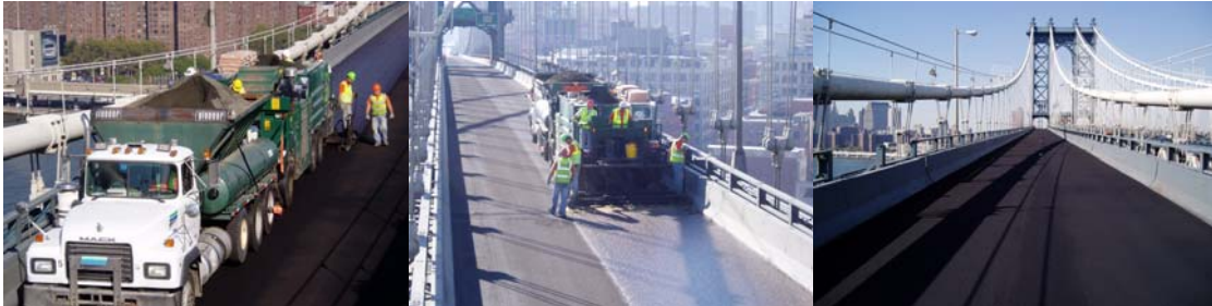
Contract #11 in 2005: Placing the New Microsurfacing on the South Upper Roadway. Newly Resurfaced Roadway.
