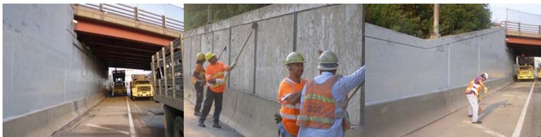
Bridge Painters Removing Graffiti From the Long Island Expressway.
