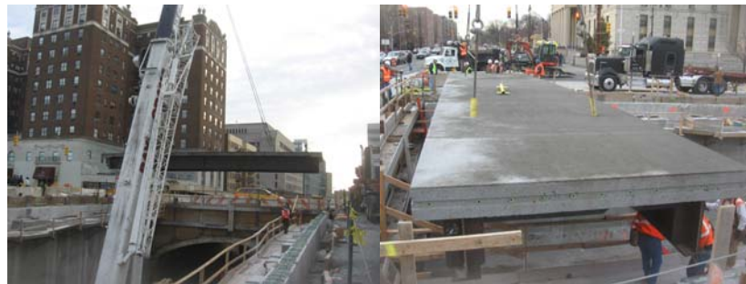
Installing the Precast Panels.
