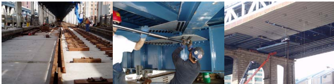
Contract #10 Installation of New Ties for the North Subway Track. Torquing the Bolts for the Installation of the Upper Laterals for the Truss Stiffening System. Installation of a Permanent Maintenance Platform Under the Bridge on the Brooklyn Approach Span.
