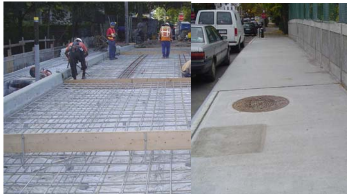
Installing Galvanized Rebar for the Approach Slab. East 3 rd Street Bridge After Reconstruction.
