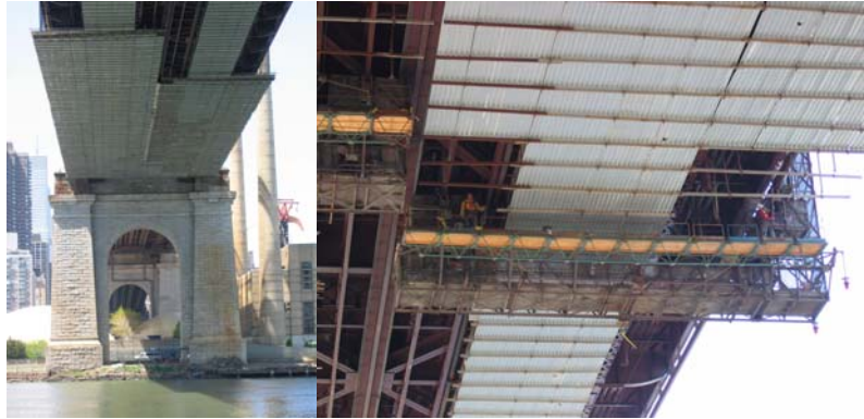
Queensboro Bridge Work Platform. Painters Arriving at the Platform. (Credit: Michele N. Vulcan)
