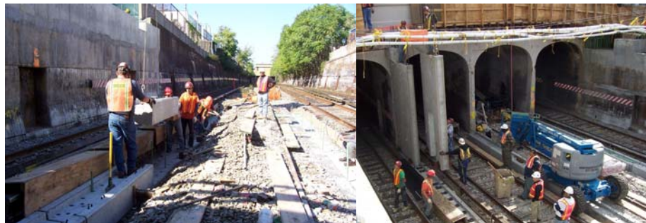
Installing Precast Concrete Footings and Pier Walls for the 17 th Avenue Bridge.
