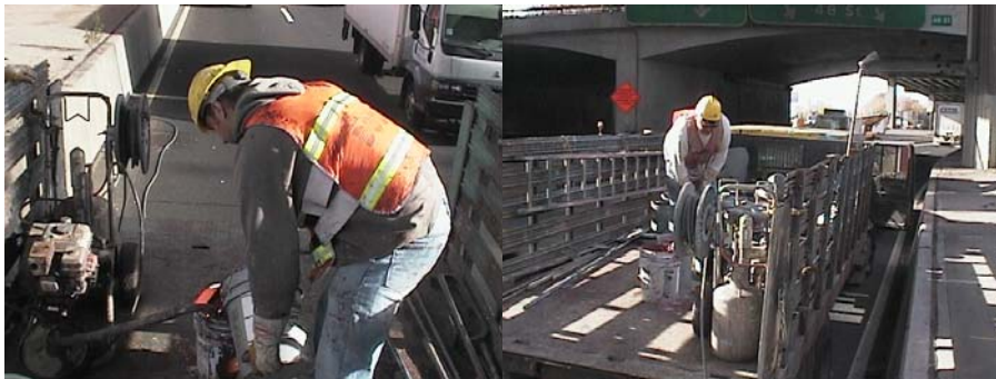
Bridge Painters Frank Duic and Russell Newme Feeding the Spray Pump And Preparing the Paint.
