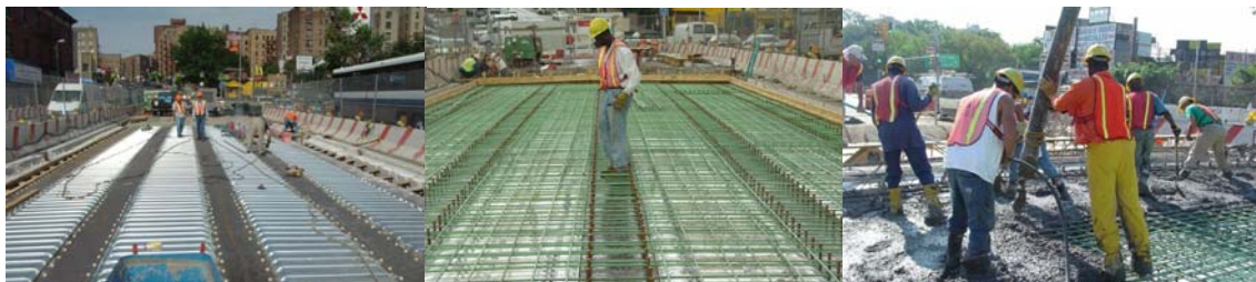
Project Engineer Muhammad Siddiqui Inspecting the Stay-in-Place Formwork for the New Gun Hill Road Bridge Deck. Installing Deck Reinforcement. Concrete Placement.
