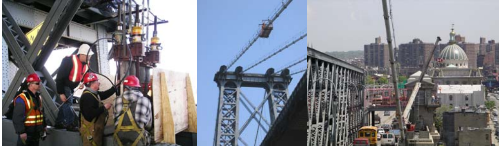
Contract #8 in 2005: Adjusting the Suspender Cables. Cable Band Bolt Retensioning. (Cable Band Credit: Bojidar Yanev) Demolition of the Brooklyn South Comfort Station Balcony.
