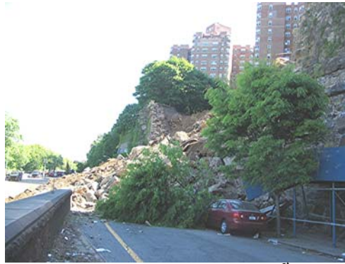
The Collapsed Retaining Wall Near 181 st Street.
