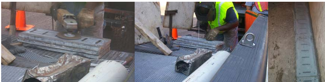
Installing Mesh Cover Strips Over the Drainage Gratings Along the Sides of the 191 st Underground Street to Broadway.
