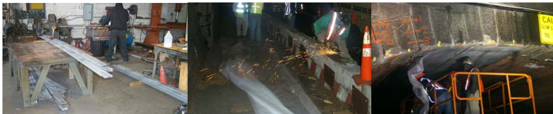
Central Drive Bridge Over Transverse Road #1: Preparing Bracing and Mesh to Protect the Bridge From Falling Debris.
