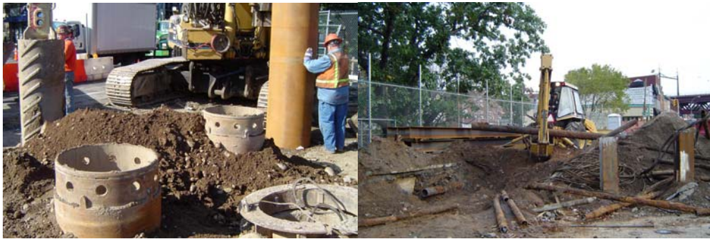
Preparing to Install Piles at the Southern End of the South Bridge. Removing the Utility Conduit Pipes From the Western Side of the Steinway Street Bridges.
