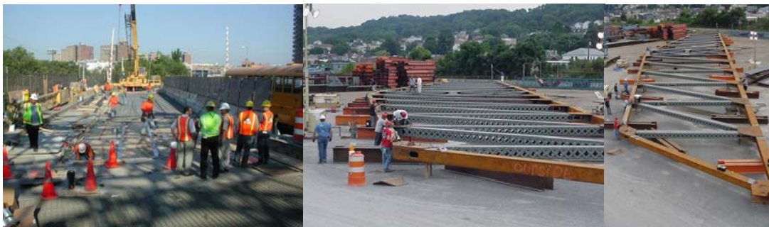
Replacing Span #3. Swing Span Truss Assembly.
