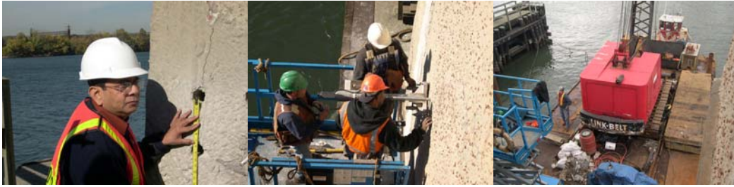
Director of the When and Where Unit Sudhir Jariwala Measuring the Diameter of Holes Drilled Through the 4-Foot Thick Walls of the Shore Road Over Hutchinson River Bridge Operator House. Drilling the Holes for Threaded Steel Rods. Working From the Barge.
