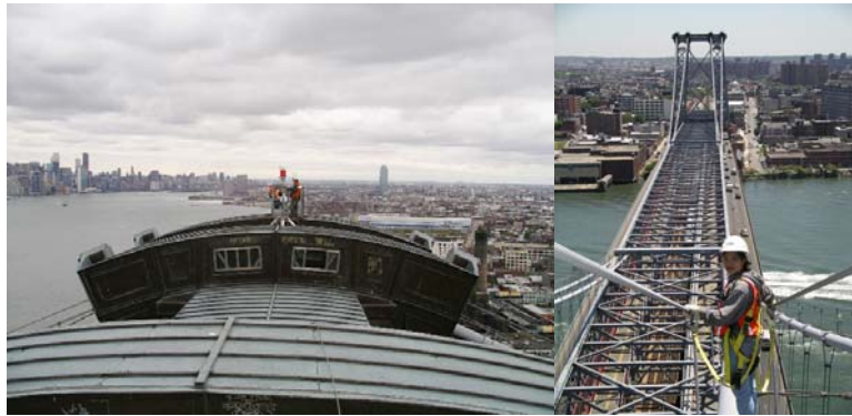
Installing Brooklyn Main Tower Aviation Lights. FHWA Engineering Intern River Hwang Inspecting the Cable Wrapping.
