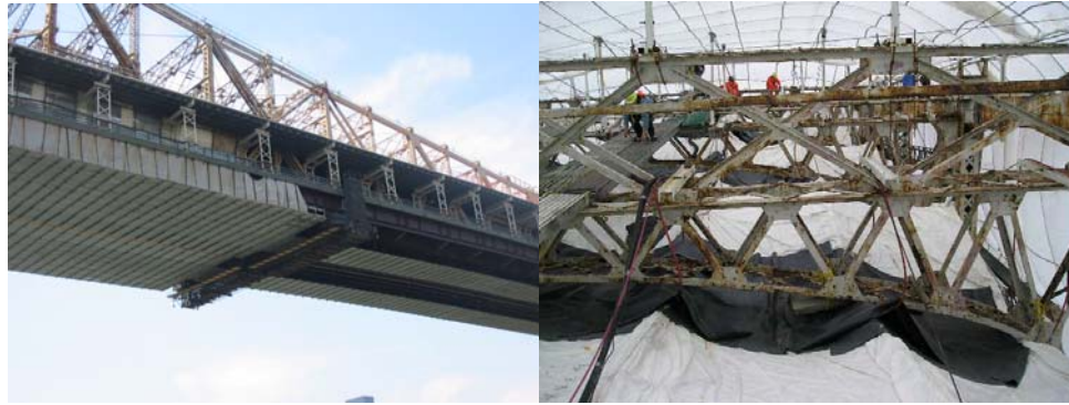
Platform Installed for Painting of the Queensboro Bridge. (Credit: Vadim Sokolovsky) Working Inside the Containment.
