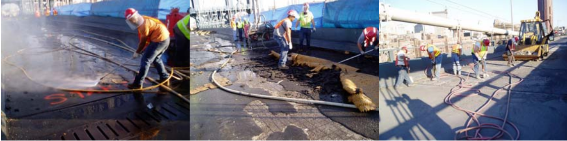
Waterblasting to Remove Existing Microsurfacing From the South Upper Roadway. Manually Removing the Microsurfacing.
