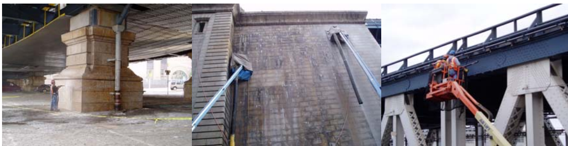
Masonry Cleaning of the Brooklyn Granite Pier and of the North Face of the Brooklyn Anchorage. Installing Conduit for the New North Upper Roadway Street Lighting.
