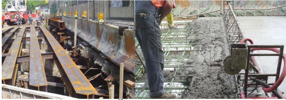
Installation of Structural Steel on 52 nd Street Bridge. Placing Concrete on the Bridge Deck.
