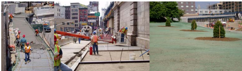
Placing Concrete on Manhattan Approach Ramp of New North Bikeway. Finishing Concrete for the Sidewalk Along Forsyth Street. Landscaping Work in Progress Along the Brooklyn Approach Ramp of the North Bikeway.
