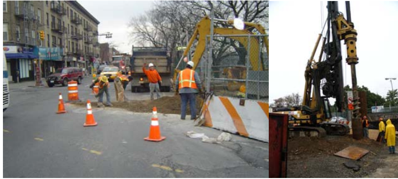
Utility Workers Excavating a Trench In Order to Deactivate the Feeder Cables in the Manholes Along Steinway Street. Driving a Sleeve for the Installation of Piles at the Center Fill Area.
