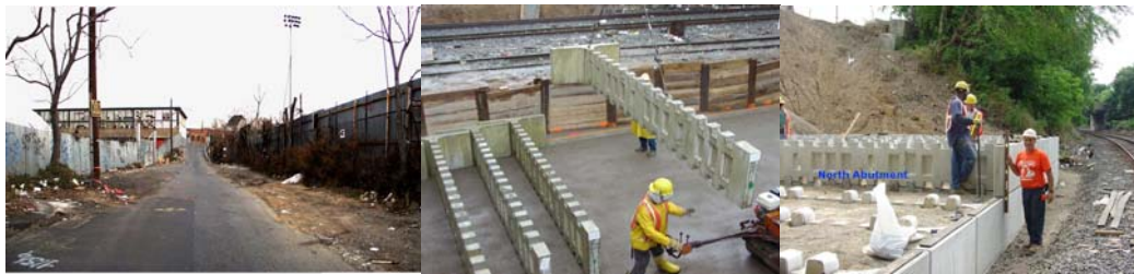
Andrews Avenue Bridge Prior To Reconstruction. Installing Pre-Cast T-Wall for the Modular Abutments. Constructing the Third Level of the Pre-Cast Abutment. (Credit: Syed Alam)
