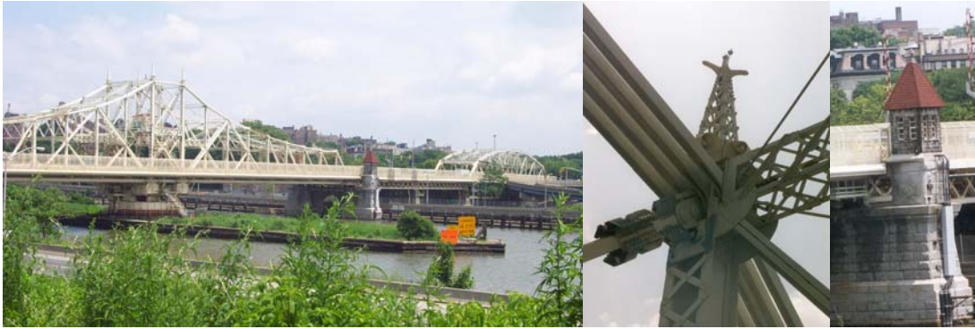
East View of Macombs Dam Bridge Swing Span and Camelback Truss. (Credit: Peter Basich)
