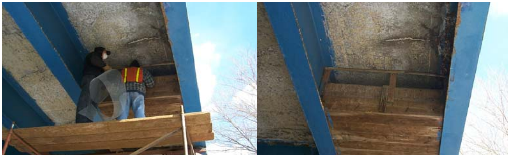
Installing Timber Shielding and Pigeon Netting at the Belt Parkway Over Rockaway Parkway Bridge.
