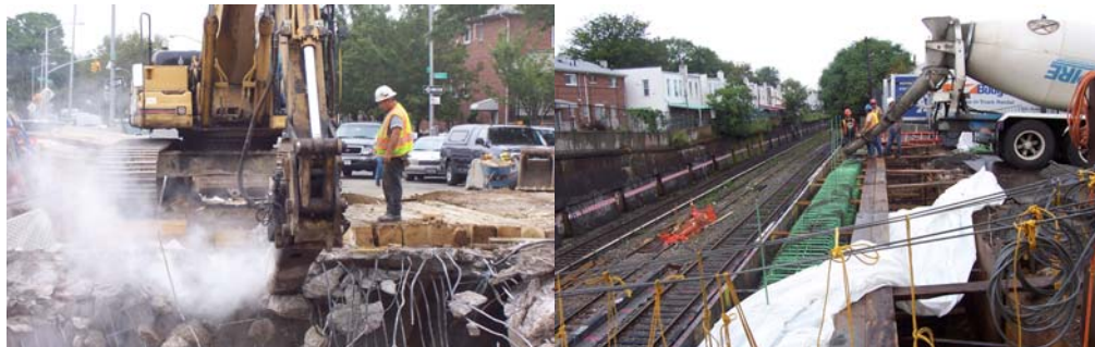
Demolition of the 17 th Avenue Bridge Deck. Casting the New East Abutment Wall.
