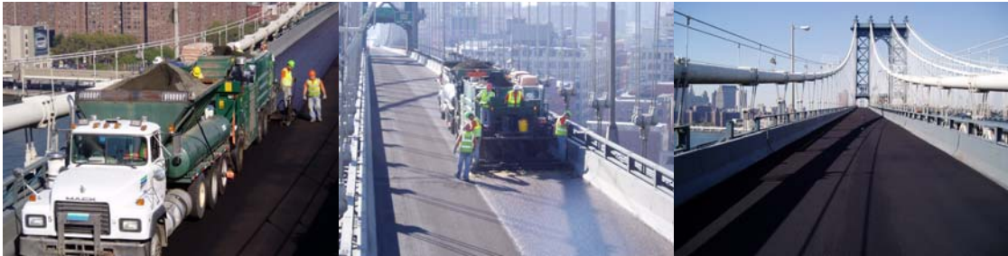
Placing the New Microsurfacing on the South Upper Roadway. Newly Resurfaced Roadway.
