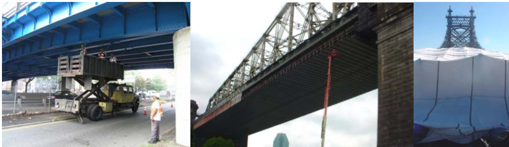
Supervisor Bridge Painter Osvaldo Lima Checking the Progress of Bridge Painters Brian Kavanagh, Thomas Jones, and Michael Scohi on the East 12 th Street Bridge Over Belt Parkway. (Credit: Sergiy Parayev) Queensboro Bridge Work Platform & Containment. (Queensboro Credit: Daniel Lima)
