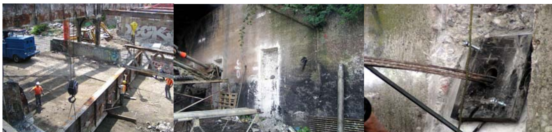
Demolishing the Old Glenmore Avenue Bridge. Installing Tiebacks at the East Abutment.
