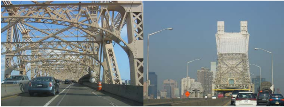
Newly Painted Section Along the Upper Roadway. Containment on the Queens Side Tower. (Credit: Peter Basich)
