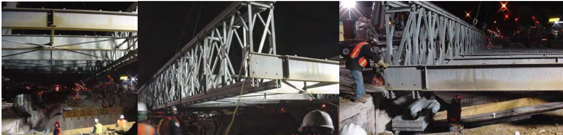
Erection of the North Temporary Bridge.
