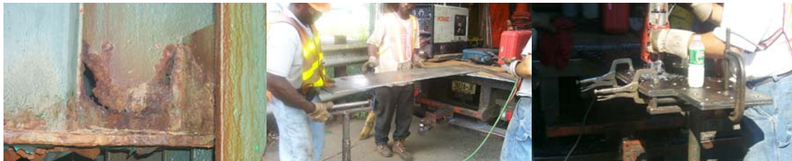
Reinforcing A Flagged Stringer Web at the Brooklyn-Queens Expressway Bridge Over Nassau Street.
