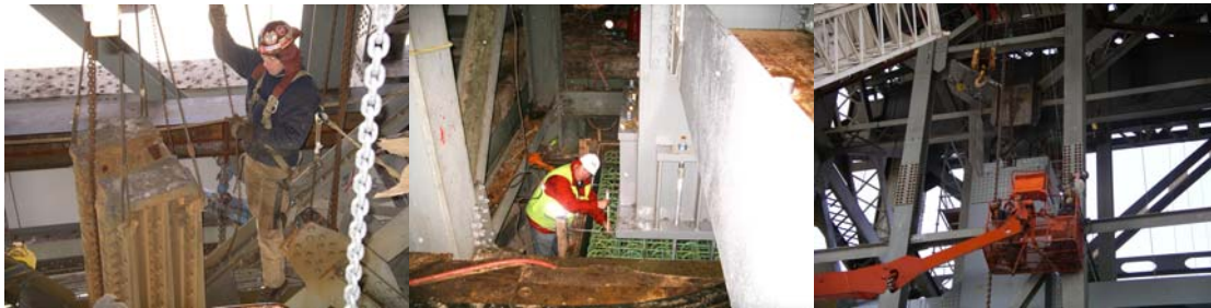
Contract #8 in 2005: Removing the Existing Steel of the Brooklyn Main Tower. Inspecting a Rebar Cage at the Manhattan Main Tower. Installing a Column at the Brooklyn Main Tower.
