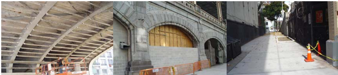
Contract #6 in 2004: Repairing Spalled Concrete at the 59 th Street Overpass. Sanitation Arch Infill Work Progressing at 60 th Street. Repaired Sidewalk Between 61 st & 62 nd Streets.
