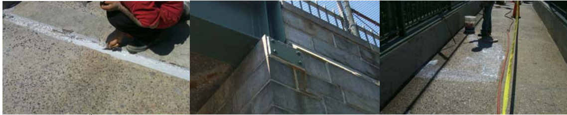
236 th Street Pedestrian Bridge over Henry Hudson Parkway: Epoxy Grout Repairs of Cracks and Between the Stones. Waterproofing the Deck.
