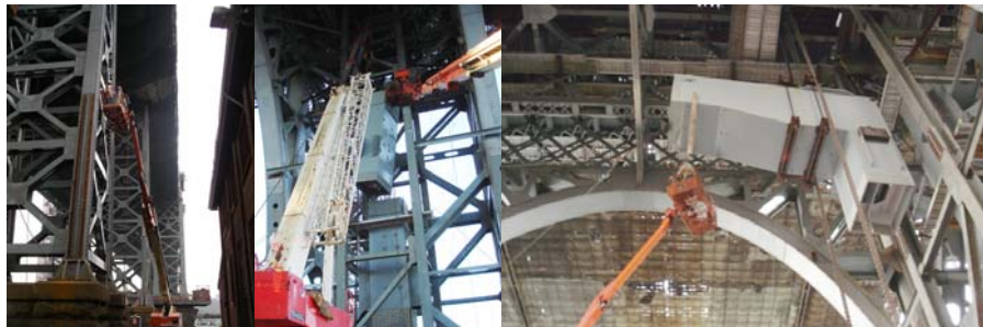
Contract #8 in 2005: Torque Testing Bolts at the Brooklyn Intermediate Tower. Erecting a Leg of the Brooklyn Main Tower. Erecting Brooklyn Main Tower Leg Bearing Support Steel.
