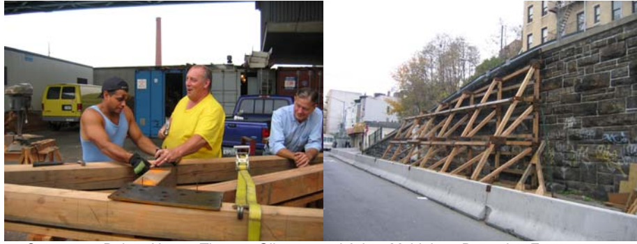
Carpenters Ruben Urena, Thomas Gilmore, and Adam Muhleisen Preparing Forms to Temporarily Shore Up the Damaged Retaining Wall at Decatur Avenue and 197 th Street. (Credit: Michele N. Vulcan) The Completed Shoring.
