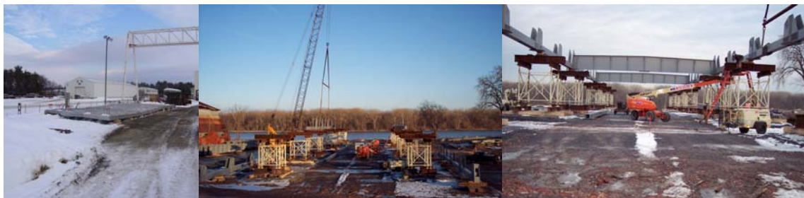
Precast Deck Units at the Fabrication Facility. Placing the Bottom Chord of the Swing Span on the Supporting Towers.
