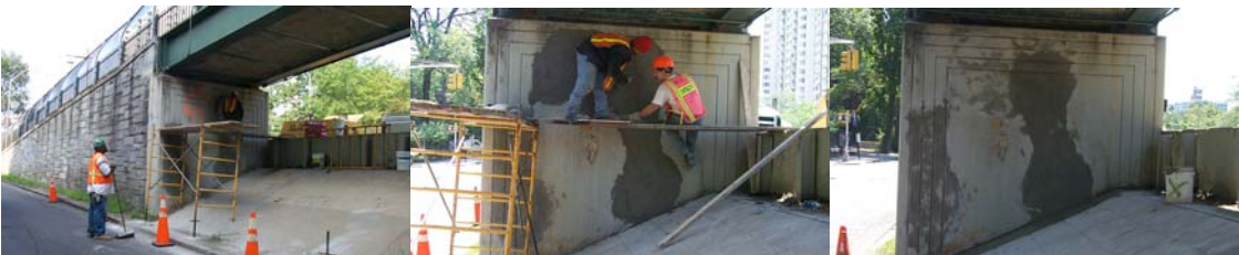
236 th Street Pedestrian Bridge over Henry Hudson Parkway: Repairing the Abutment Walls.
