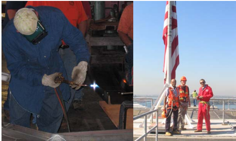
Bridge Repairer and Riveter David Collins Participating in the Demonstration of Heat Straightening Techniques for Damaged Steel Bridges at a FHWA Workshop in New Hartford, New York. (Credit: George Klein) Director of Bridge Inspection Jyotish Shah, Engineering Intern Devin Plantamura, and Executive Director of Inspections and Bridge Management Dr. Bojidar Yanev Atop the Brooklyn Tower of the Brooklyn Bridge. (Credit: Avelino Leyco)
