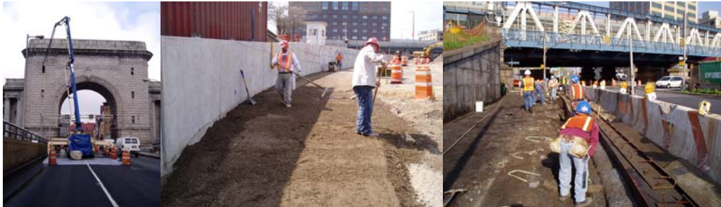
Placing Concrete for the New Interior of the Manhattan Colonnade and Arch. Preparing Subgrade for the Brooklyn Approach Ramp of the New North Bikeway and for the Path to the Bikeway Along Sands Street.
