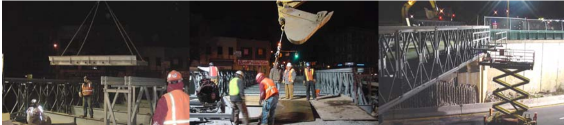
Erection of the South Temporary Bridge.
