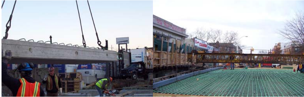
Installing Precast Deck Panels for the 17 th Avenue Bridge. Placing the Reinforced Concrete Bridge Deck.
