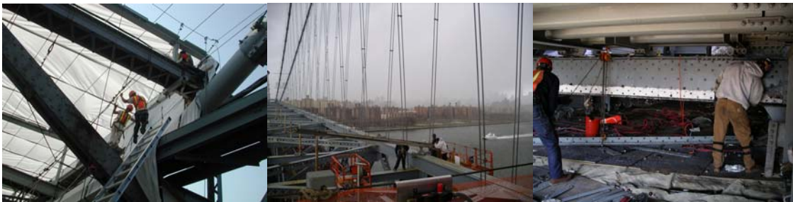
Contract #8 in 2003: North Stiffening Truss Containment Erection and Removal. South Truss Bottom Chord Rehabilitation.
