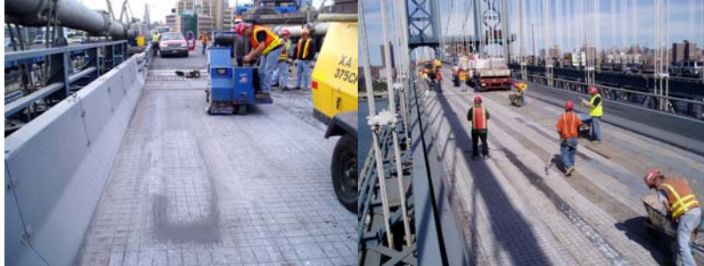
Preparing the Deck for New Microsurfacing on the South Upper Roadway.
