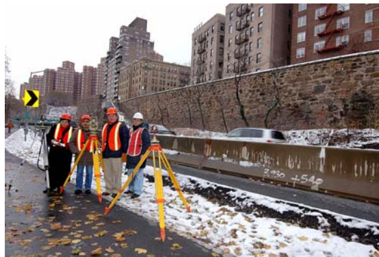
Survey Crew (Mariya Zhurakhinskaya, Aleksandr Kotlyanskiy, Alfred Lee, and Thee-Shiun Ken) Conducting Periodic Monitoring of the Retaining Wall. (Credit: Eric Ken)
