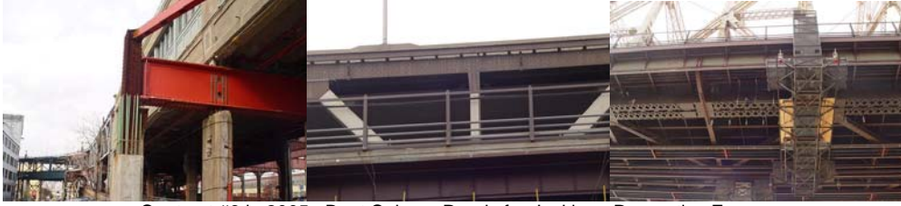
Contract #6 in 2005: Bent Column Ready for Jacking. Decorative Fence. Repairing the Drainage Pipes.
