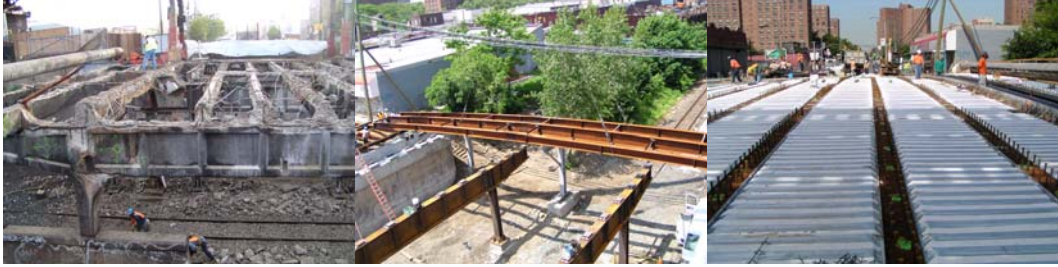
Demolishing the Old Sutter Avenue Bridge. Erecting Structural Steel. Installing Stay-in-Place Forms.
