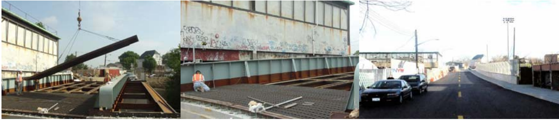
Installation of the Grid Deck. Newly Completed Andrews Avenue Bridge (Credit: Syed Alam)
