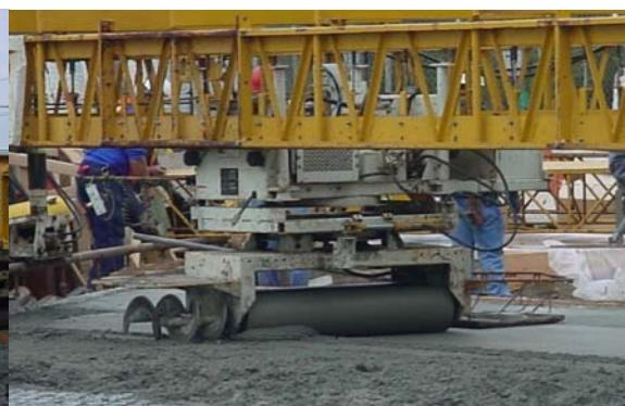
Placing Concrete for the Grid Deck of the Cross Bay Boulevard Bridge
