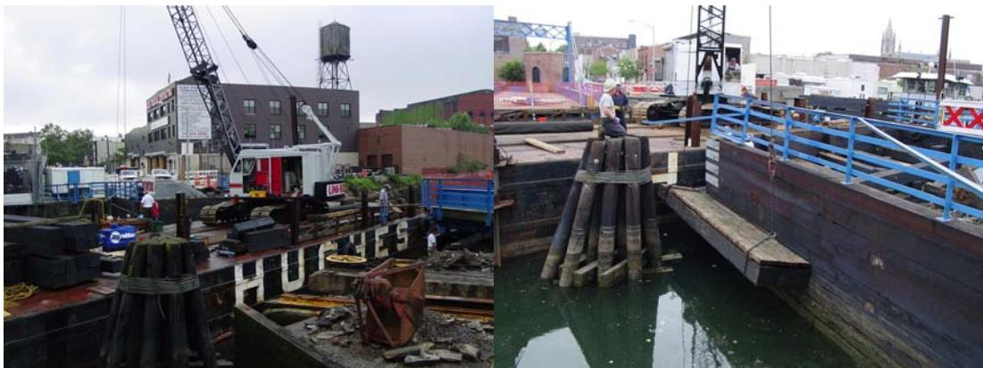
Work Barge Used During Carroll Street Bridge Repairs. Work Platform From Which the Timbers Were Replaced.
