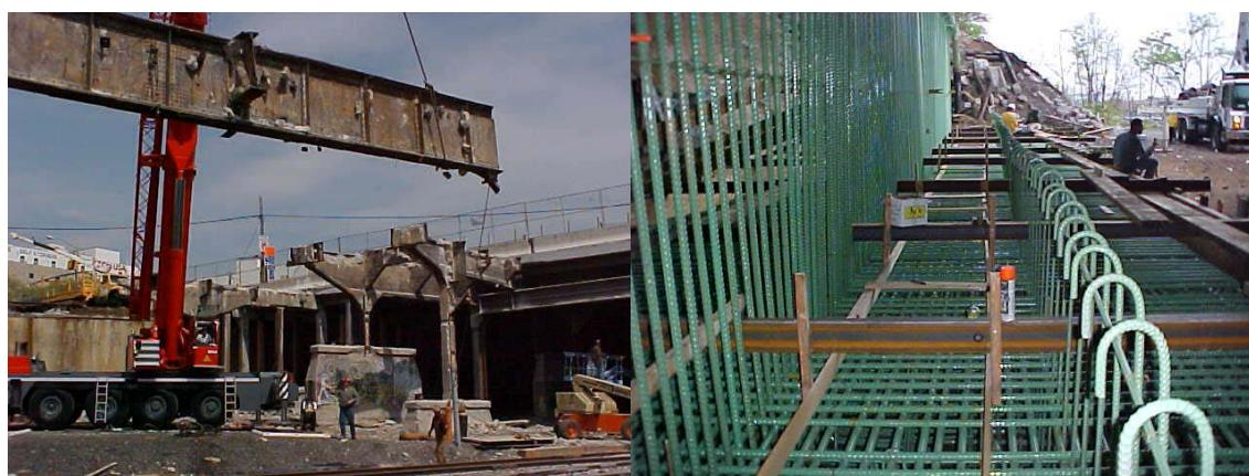
Demolition of the 2<sup>nd</sup> Avenue Bridge Superstructure. Abutment Footing and Stem Reinforcement.
