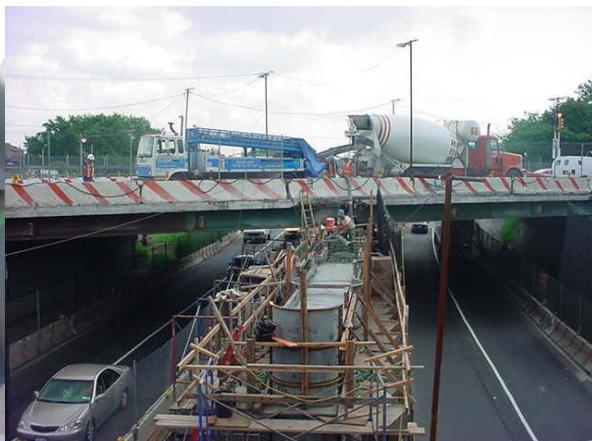
Construction of North Abutment Wall of the Cross Bay Boulevard Bridge. Placing Concrete for the Pier Cap.
