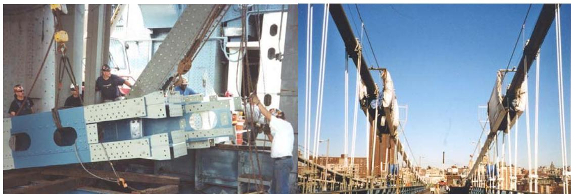
Contract #10 Installing a New End Frame on the Main Span Side of the Brooklyn Tower. Painting Containment Structures on the Cables of the Manhattan Approach Span.
