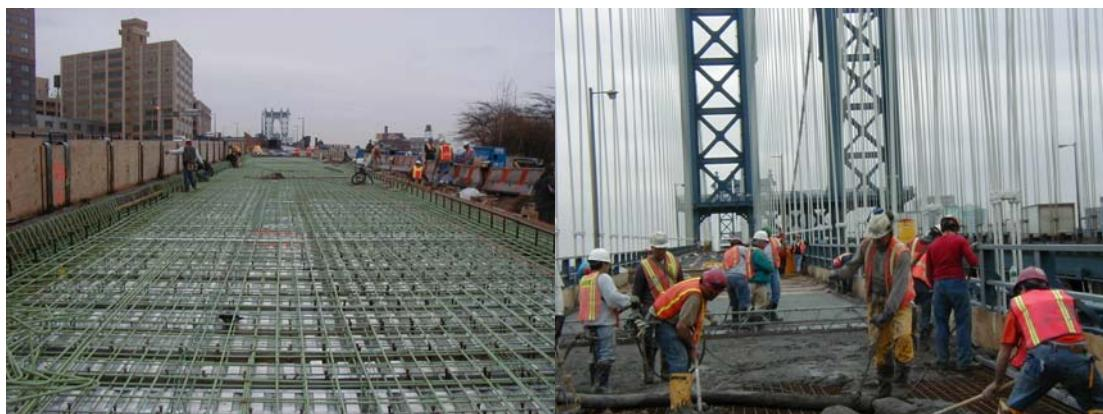
Preparing the Brooklyn Elevated Structure Grid Deck for Concrete Placement. Placing Concrete on the Manhattan Side Span Grid Deck of the North Upper Roadway.
