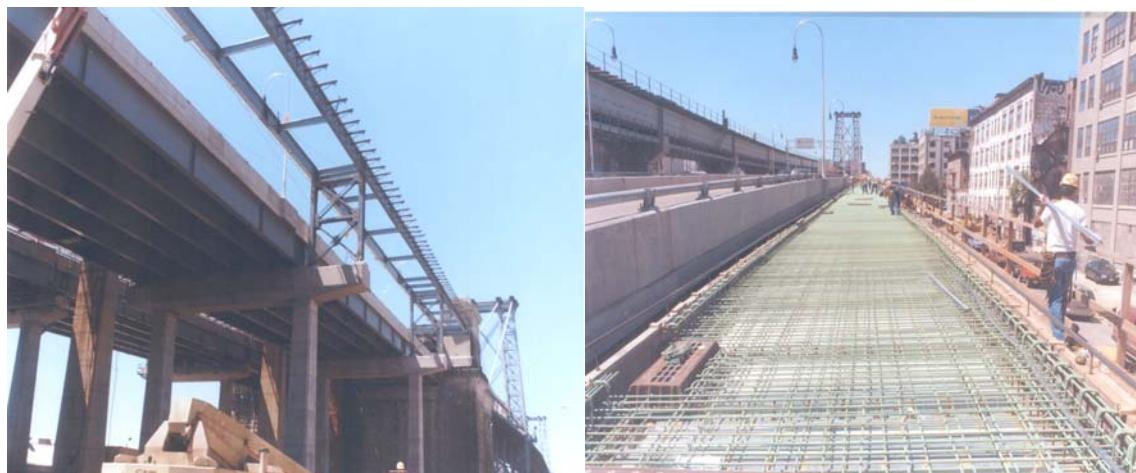
Contract #7 Bikeway Steel Erection & Rebar Installation
