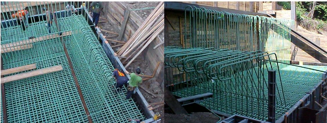
Installation of Abutment Footing and Stem Reinforcement for the 14<sup>th</sup> Avenue Bridge
