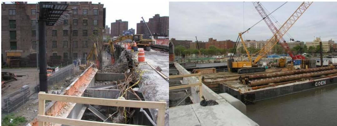
Third Avenue Bridge Stairway Demolition. Working on the River to Construct a Temporary Platform.
