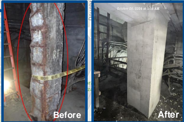
Clark Street Column & Beam Repair
