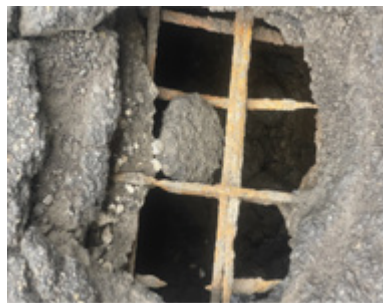
Deck through holes over Old Fulton Street
