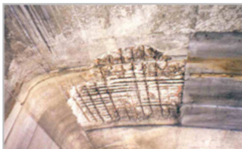
Typical joint condition along the triple cantilever
