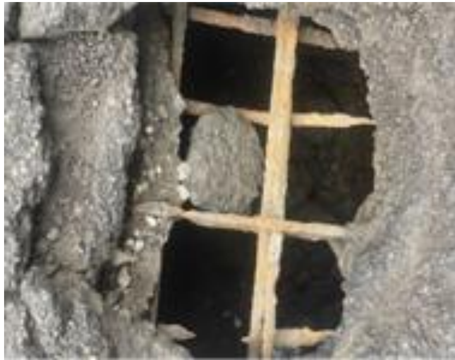
Deck through holes over Old Fulton Street
