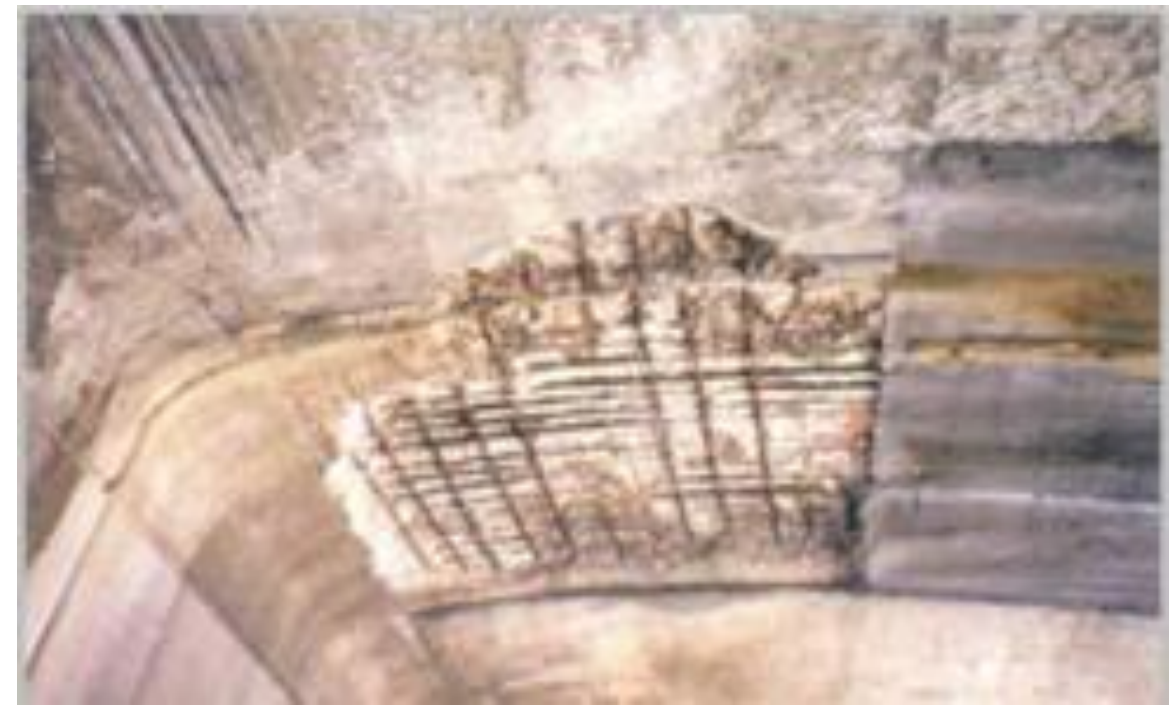
Typical joint condition along the triple cantilever
