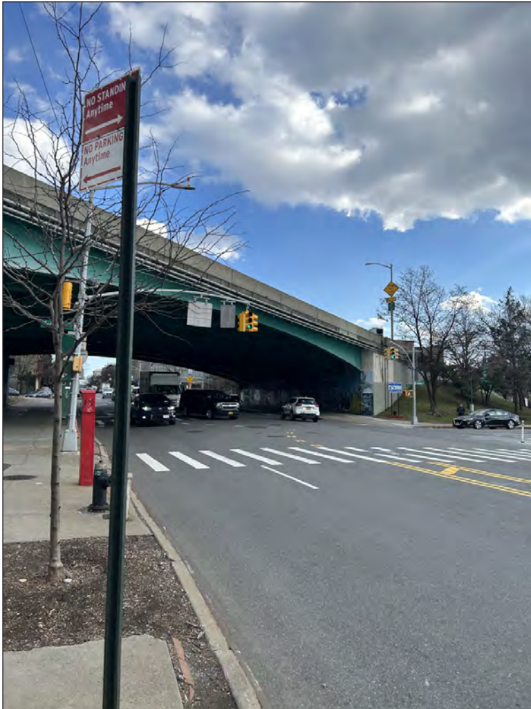
BQE Passing Above Atlantic Avenue at Columbia Street, Looking East 1
