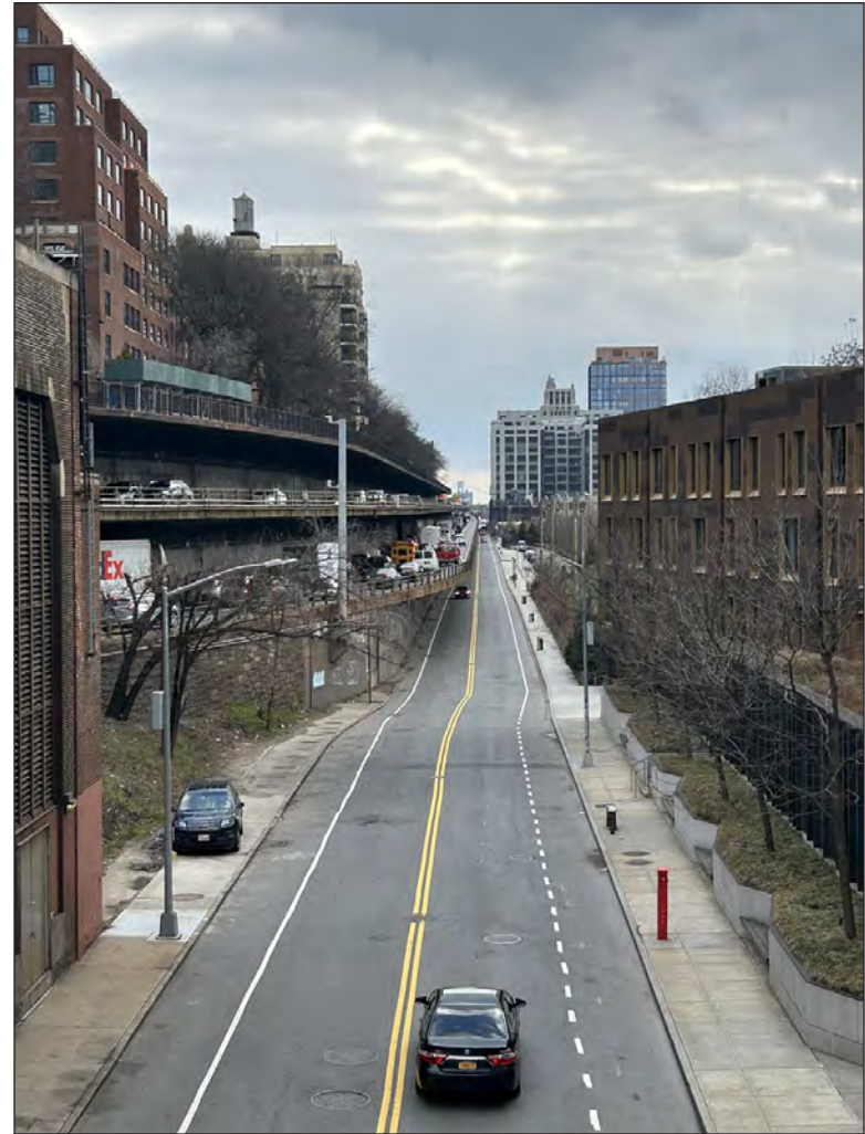
The Triple Cantilever Structure, Looking South 8
