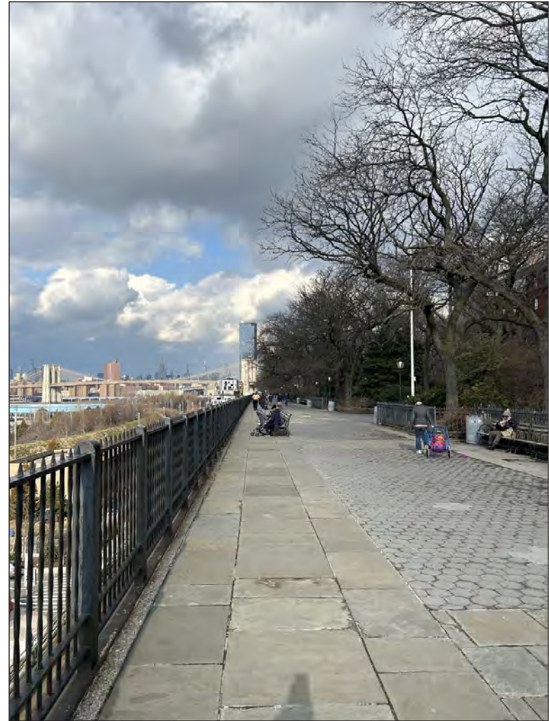
View along the Promenade, Looking North 6
