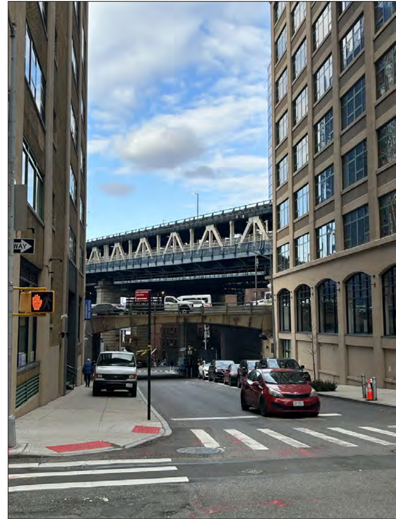
View Along Pearl Street with BQE and Manhattan Bridge, Looking North 12
