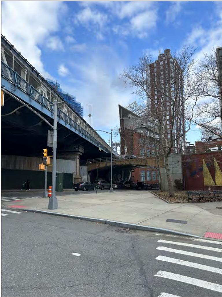
BQE Passing Beneath Manhattan Bridge and Above Jay Street, Looking North 13
