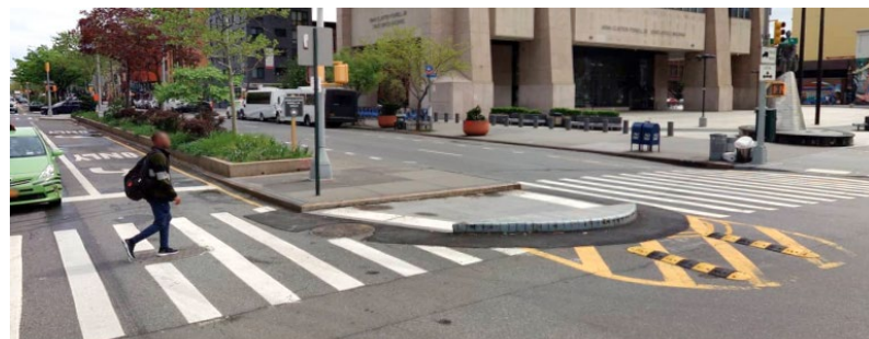
Concrete Median with Left-turn Traffic Calming Adam Clayton Powell Jr. Blvd, MN
