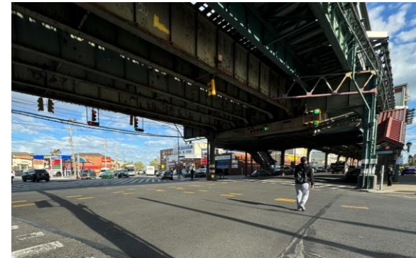
Pedestrian crossing outside cross walk at Ave X and McDonald Ave.
