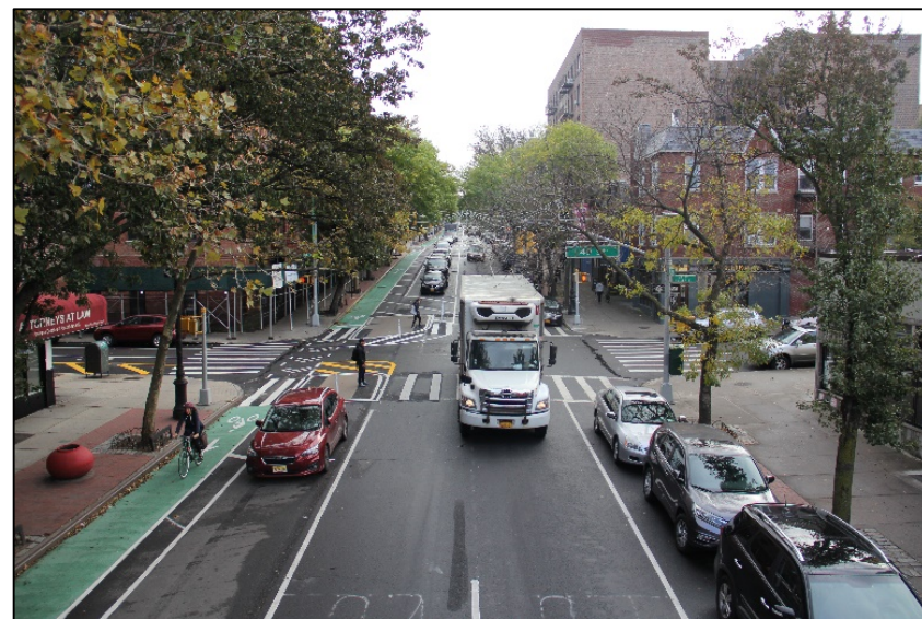
Existing conditions (above) and one-way street with protected bike lane and loading changes implemented on Skillman Ave, QN (below)
