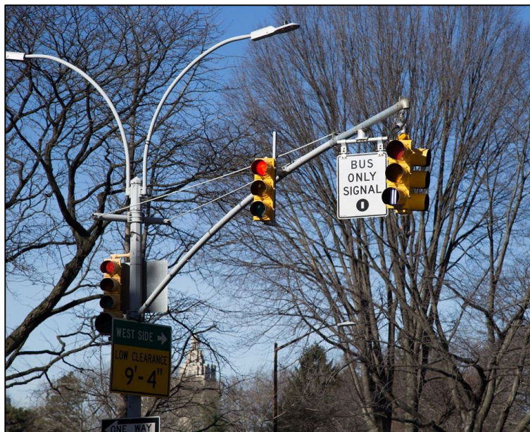
Example Bus Queue Jump Signal: 79 th St and 5 th Ave, Manhattan
