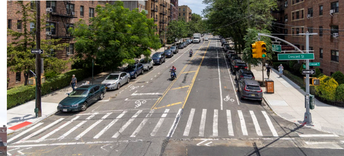
31 Ave at Crescent St Facing east BEFORE
