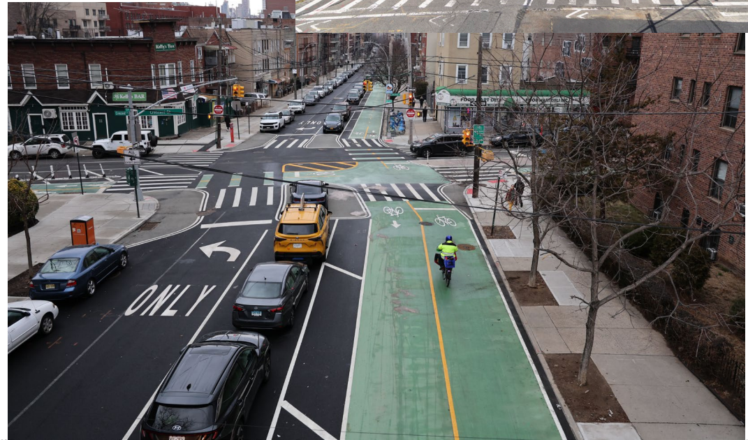
31 Ave at Crescent St Facing west AFTER
