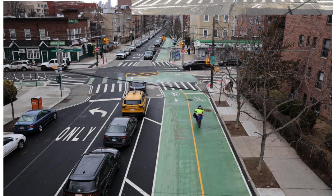
31 Ave at Crescent St Facing west AFTER
