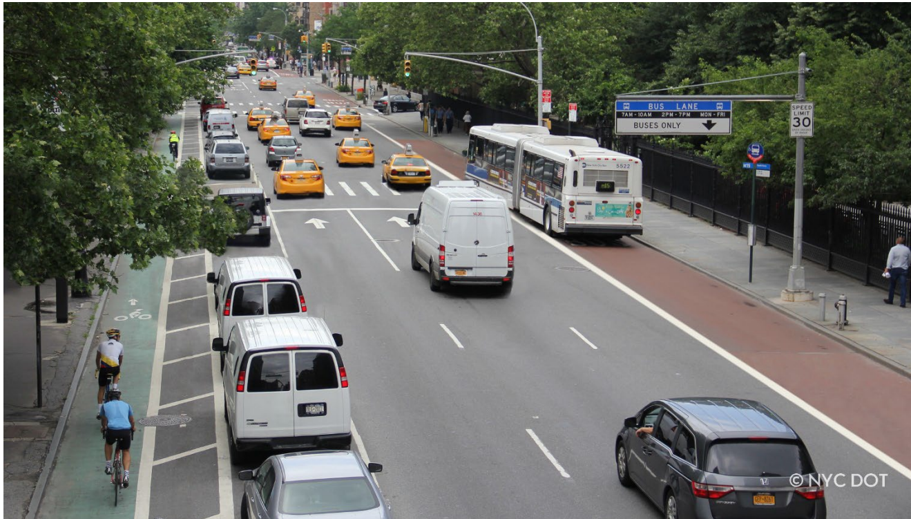
2 nd Ave at Stuyvesant Square with curbside protected bike lane and curbside bus lane
