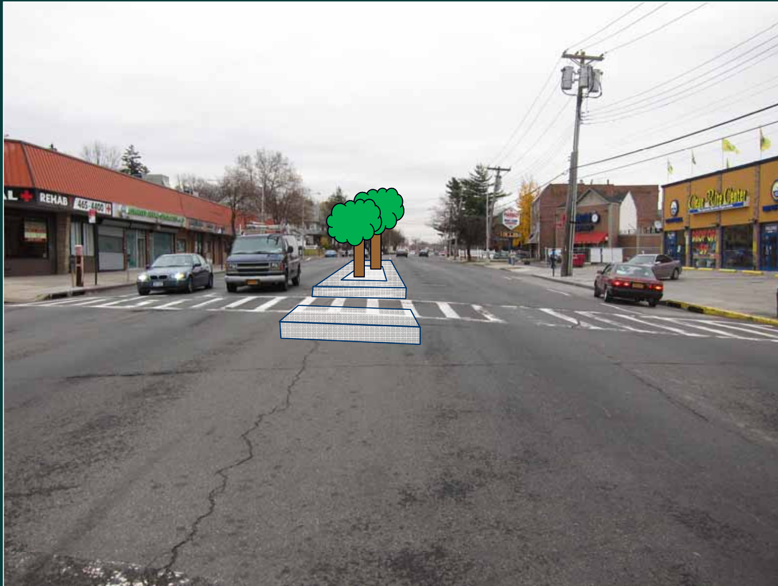
Hillside Avenue at 197 th Looking East
