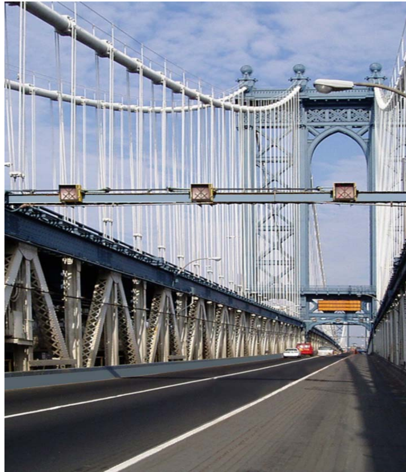
Manhattan Bridge - Contract 14
