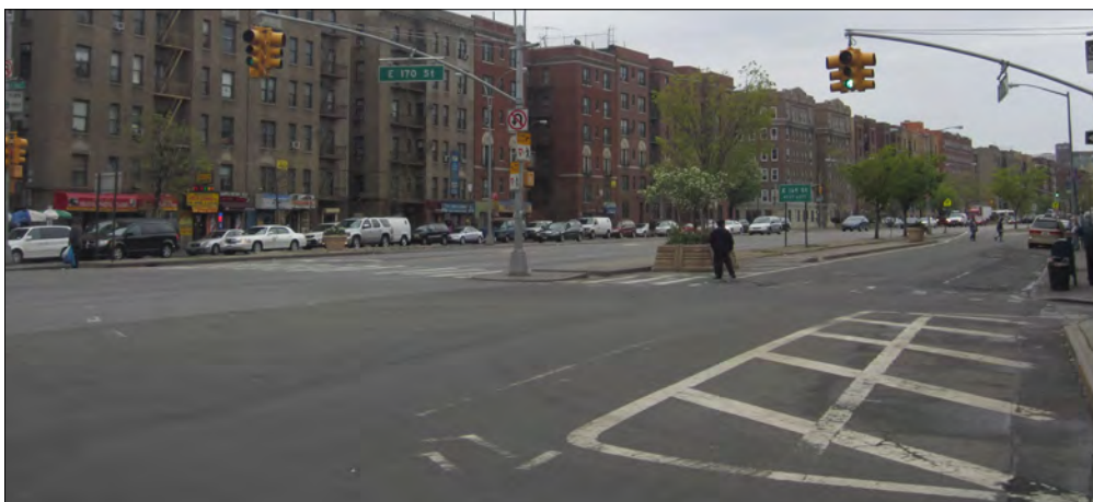
Before: Wide crossing and faded markings
