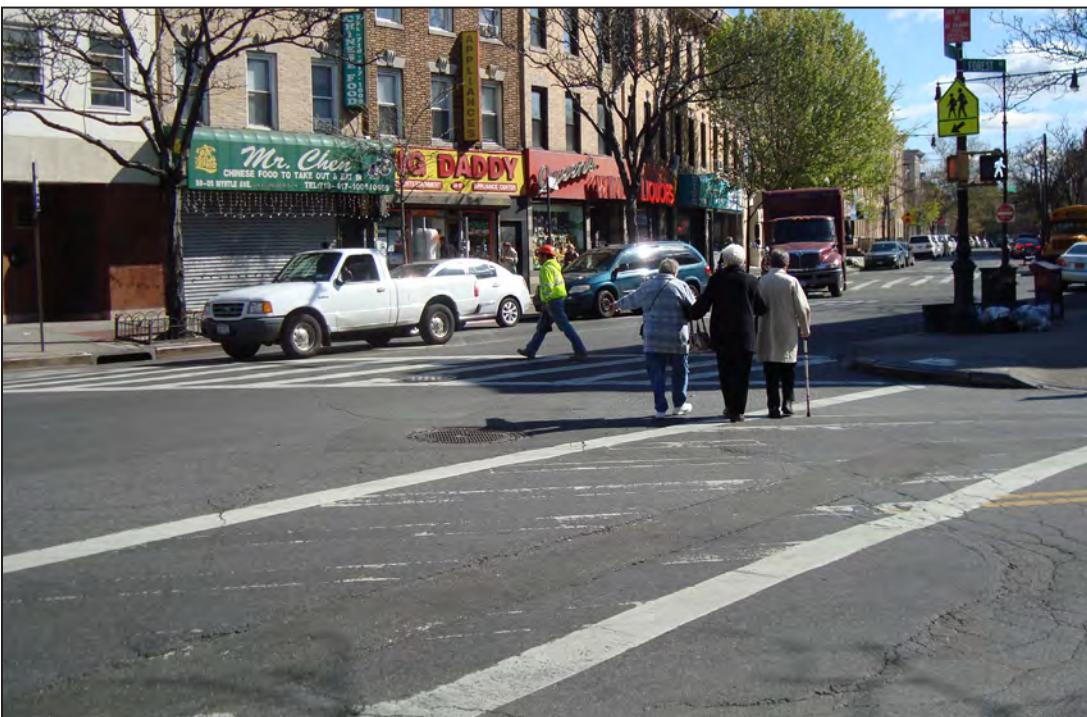
Before: Skewed intersection and crosswalks
