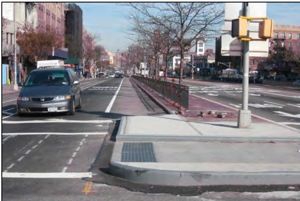
After: Median tip expansion at Grand Concourse and E 183rd Street
