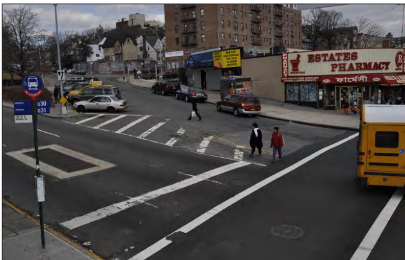
Before: Wide intersection with many vehicle-pedestrian conflicts
