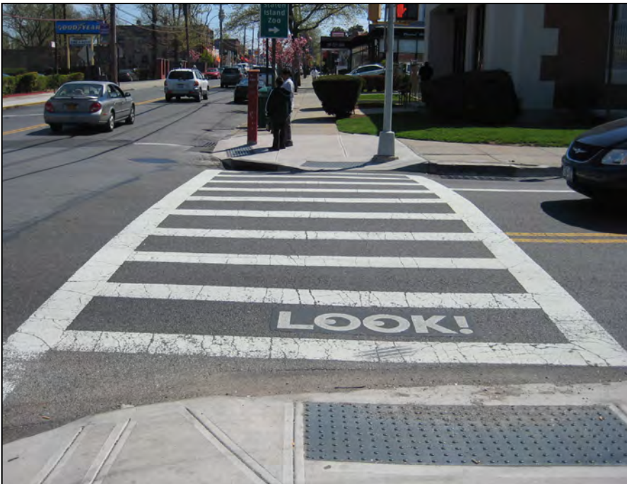
LOOK markings in place
