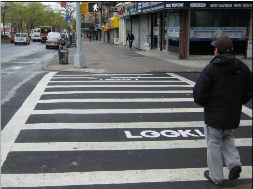
LOOK markings in place
