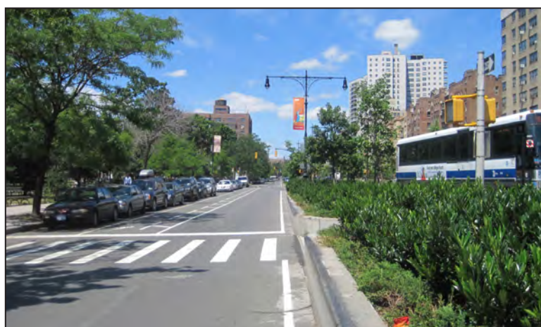
After: Example of widened landscaped medians (at 161st Street and Grand Concourse)
