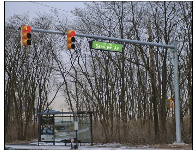
New traffic signal pole with oversized mast arm at Father Capodanno Boulevard and Seaview Avenue. In addition, an illuminated street name sign is affixed to the mast arm
