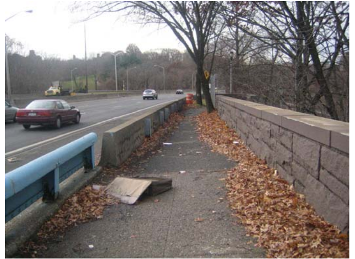
Pedestrian Overpass looking south
