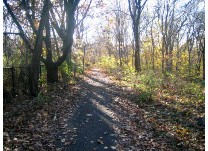
Path west of the Major Deegan Expressway to which the bridge would connect (looking south)
