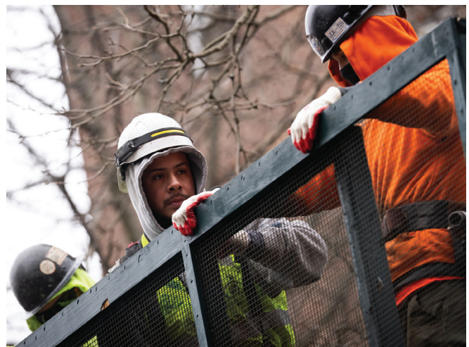
Workers take down a shed. Credit: Mayoral Photography Office
