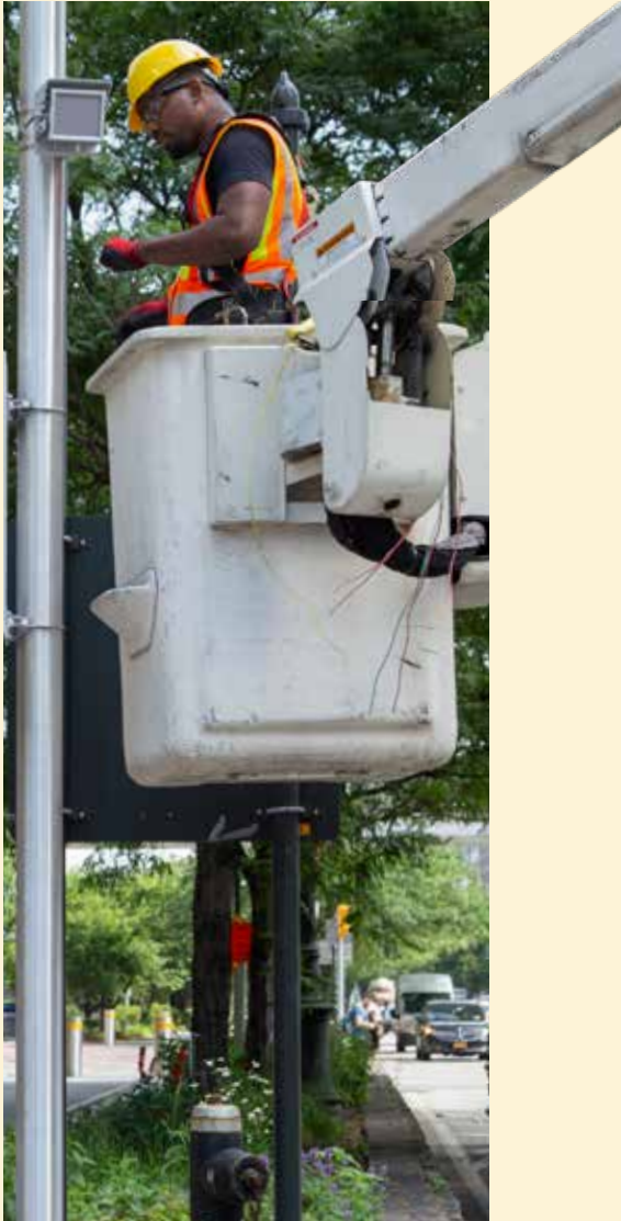
A DOT employee installs a speed camera
