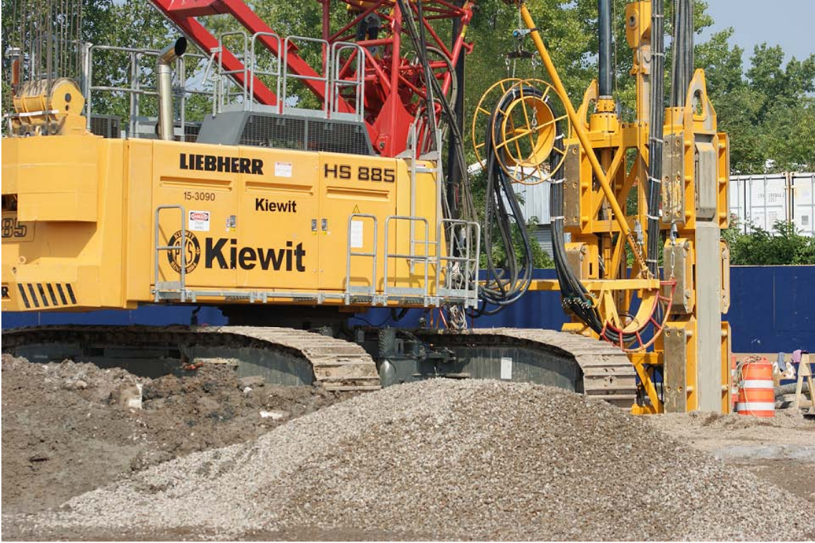
Excavation for installation of slurry wall panel
