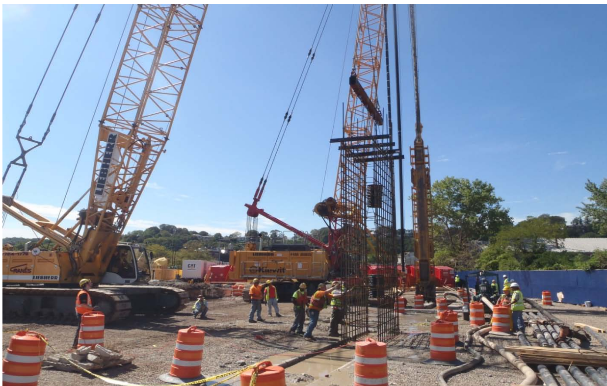
Slurry wall panel being placed at shaft site
