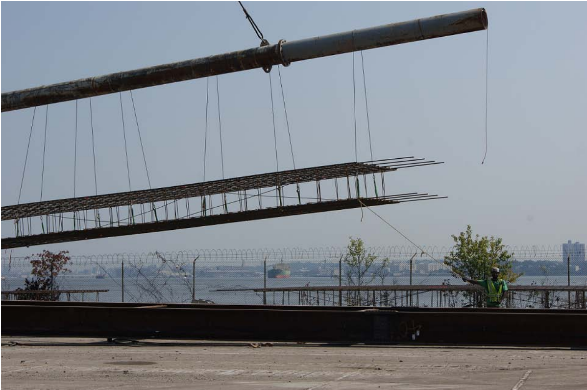
Lifting of slurry wall panel onto lifting frame
