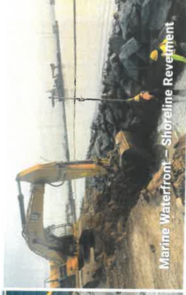
Marine Waterfront – Shoreline Revetment
