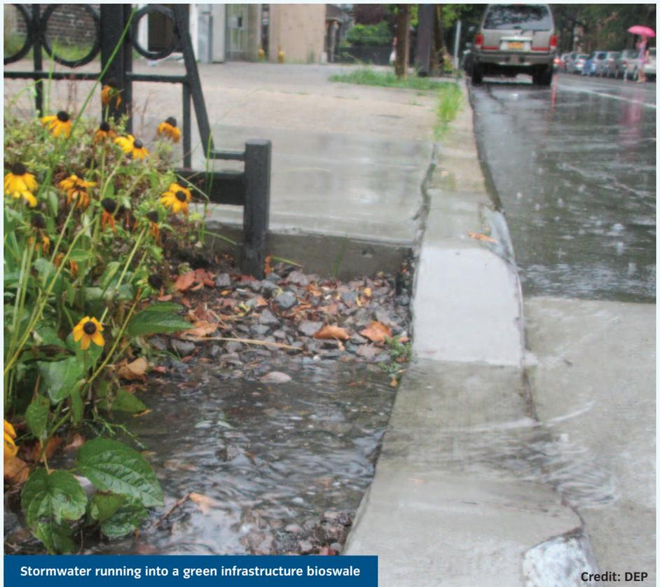
Stormwater running into a green infrastructure bioswale
