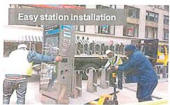
Citi Bike stations are free-standing and battery and solar-powered. Stations are installed in less than an hour and do not require any digging, construction or road work.
