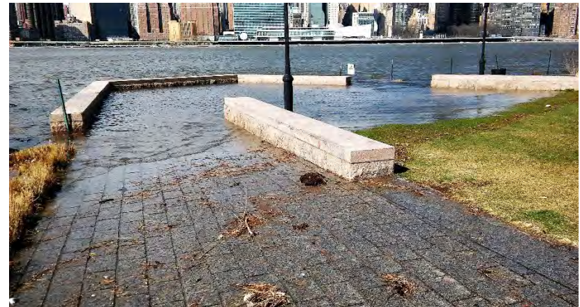
“Sunny Day Flooding” along the waterfront parks at Queens West (Source: Hunters Point Community Coalition, 2018)
