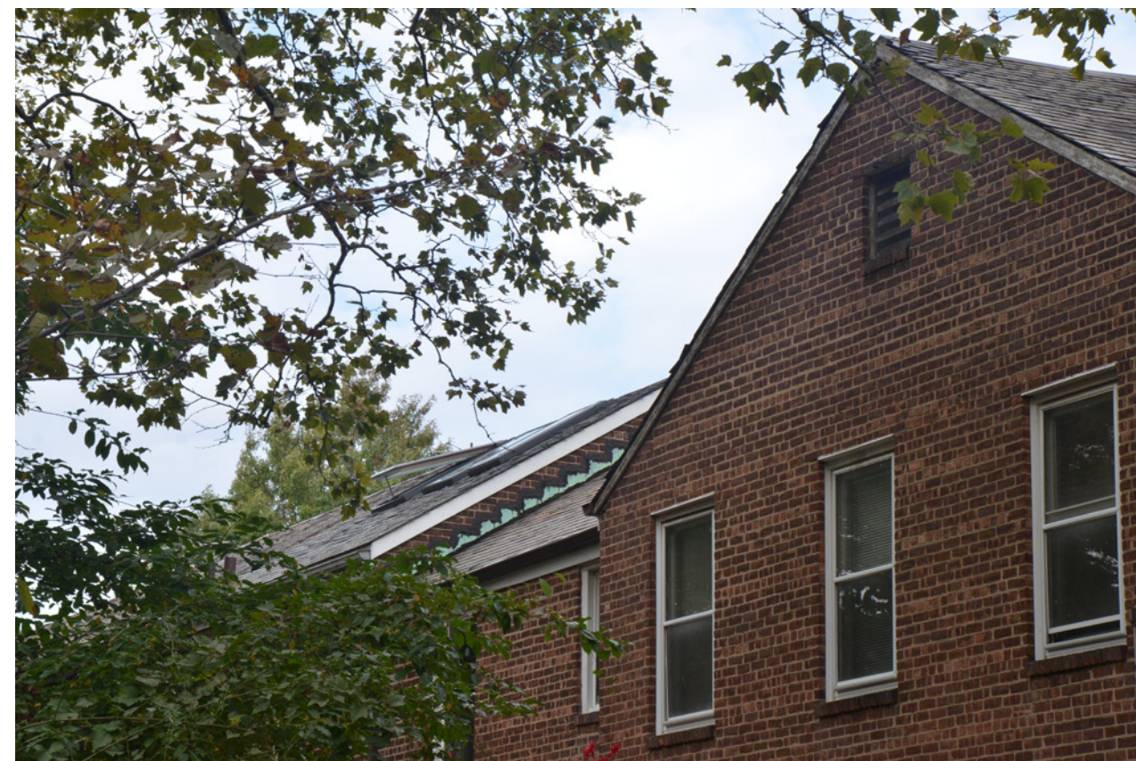
3. 40-02 44th Street - Rear Visible from 44th Street
