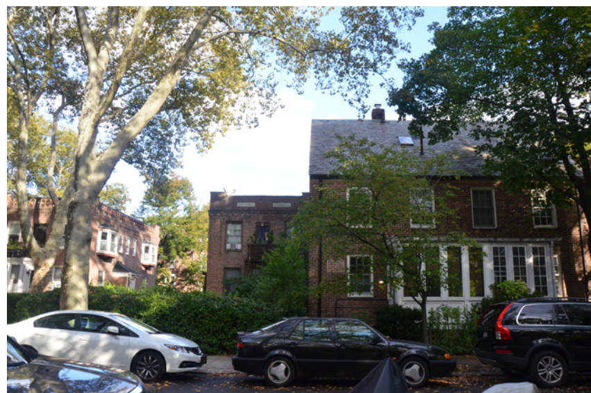
1. 39-27 46th Street - Front Visible from 46th Street
