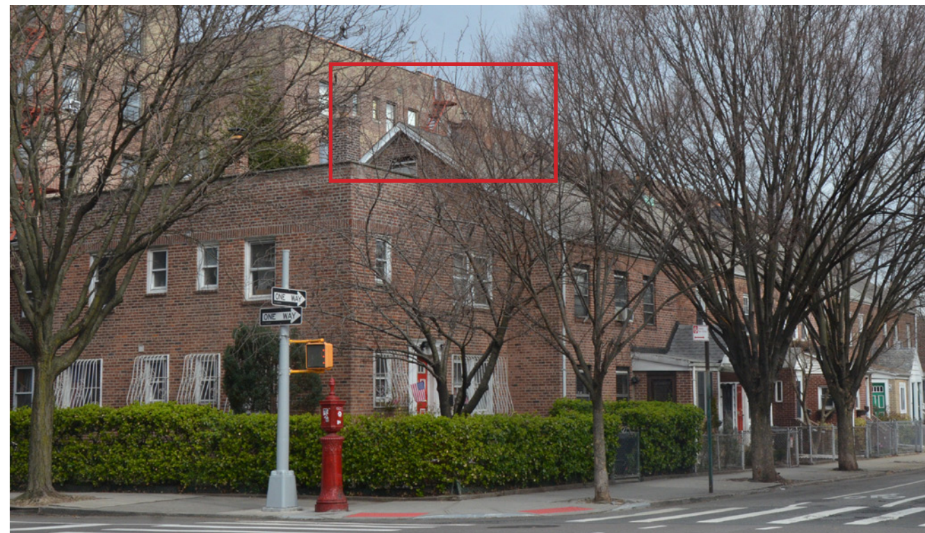
VIEW FROM 43RD STREET SIDEWALK, SE CORNER March 2023 - Skylights will not be visible, pitch of roof will obscure
