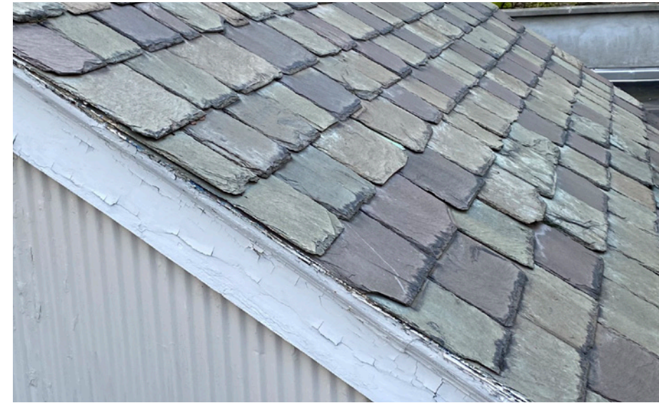
EXISTING SLATE ROOF MATERIAL
