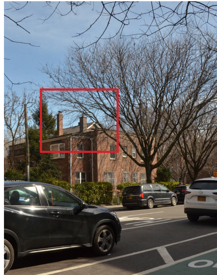
4. Rear view from 43rd Avenue (March 2023)
