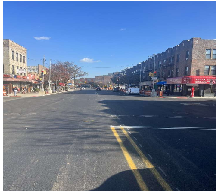
Permanent Asphalt – Grand Avenue between 71 st Street and Mazeau Street
