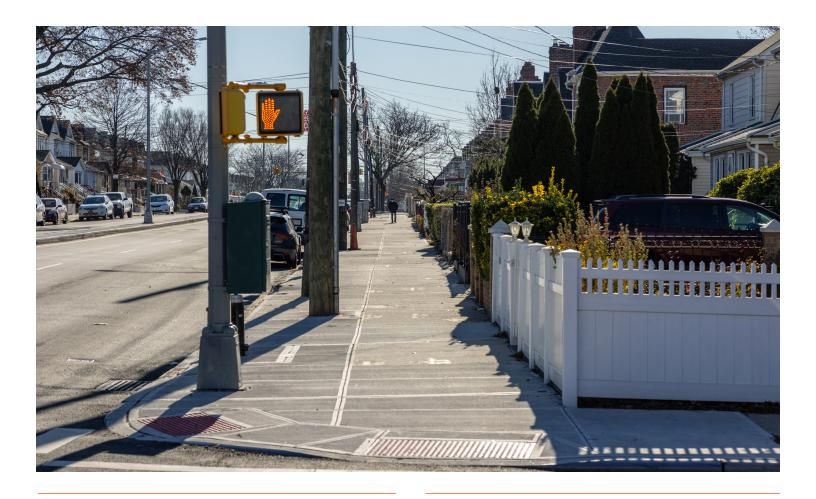
The City of New York has installed new concrete sidewalk outside your property. Please help us prevent cracks and defects in the concrete: For the first month after installation, please spray water onto the new concrete daily. This will reduce the chance of cracks forming on the surface. (Do not spray water if it might freeze in the winter.)
