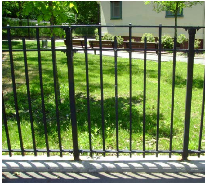
4'-0" Ht. Steel Bar Perimeter Fence
