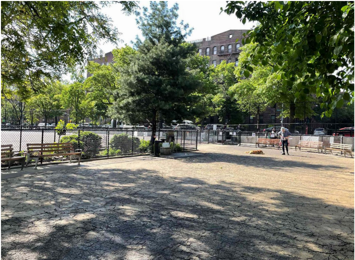
10 - Dog run for all dogs, asphalt with color seal coat cracking and in poor condition
