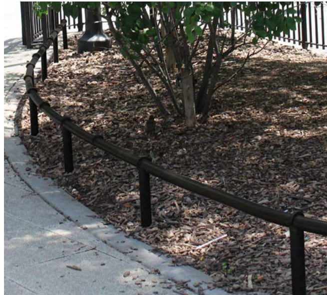
1'-0" Ht. Garden Pipe Railing Powder Coated: Black
