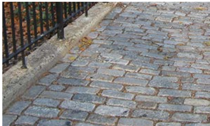
Granite Block Paving (Remove & Reinstall with Mortared Block)
