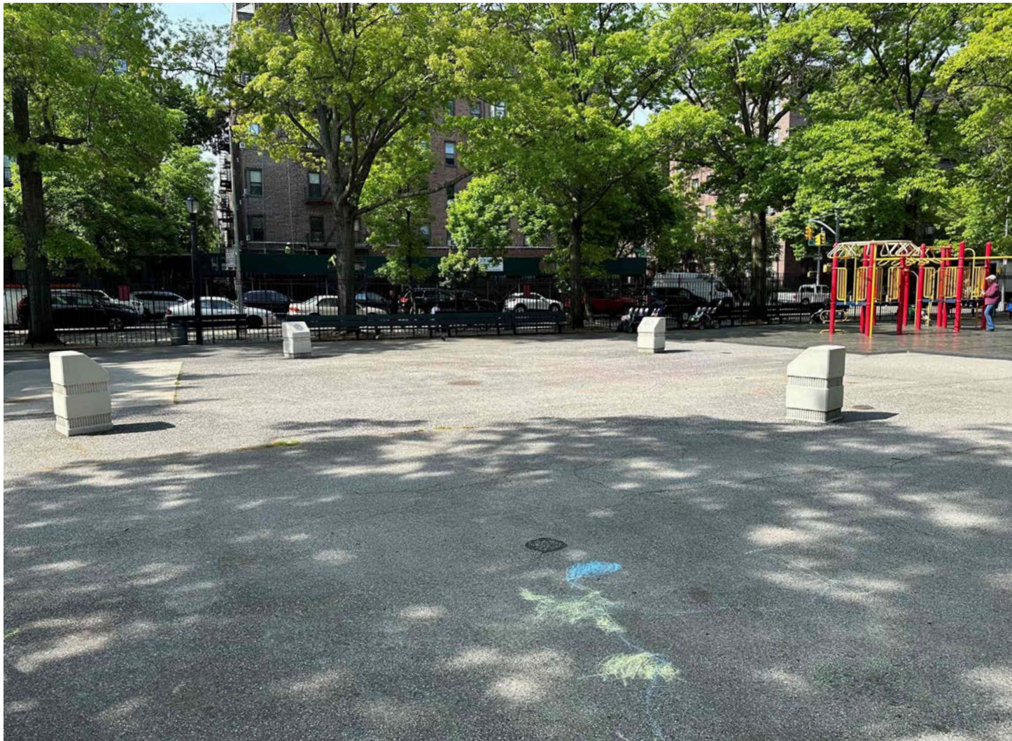
5 - Spray shower area with precast concrete spray bollards and asphalt pavement
