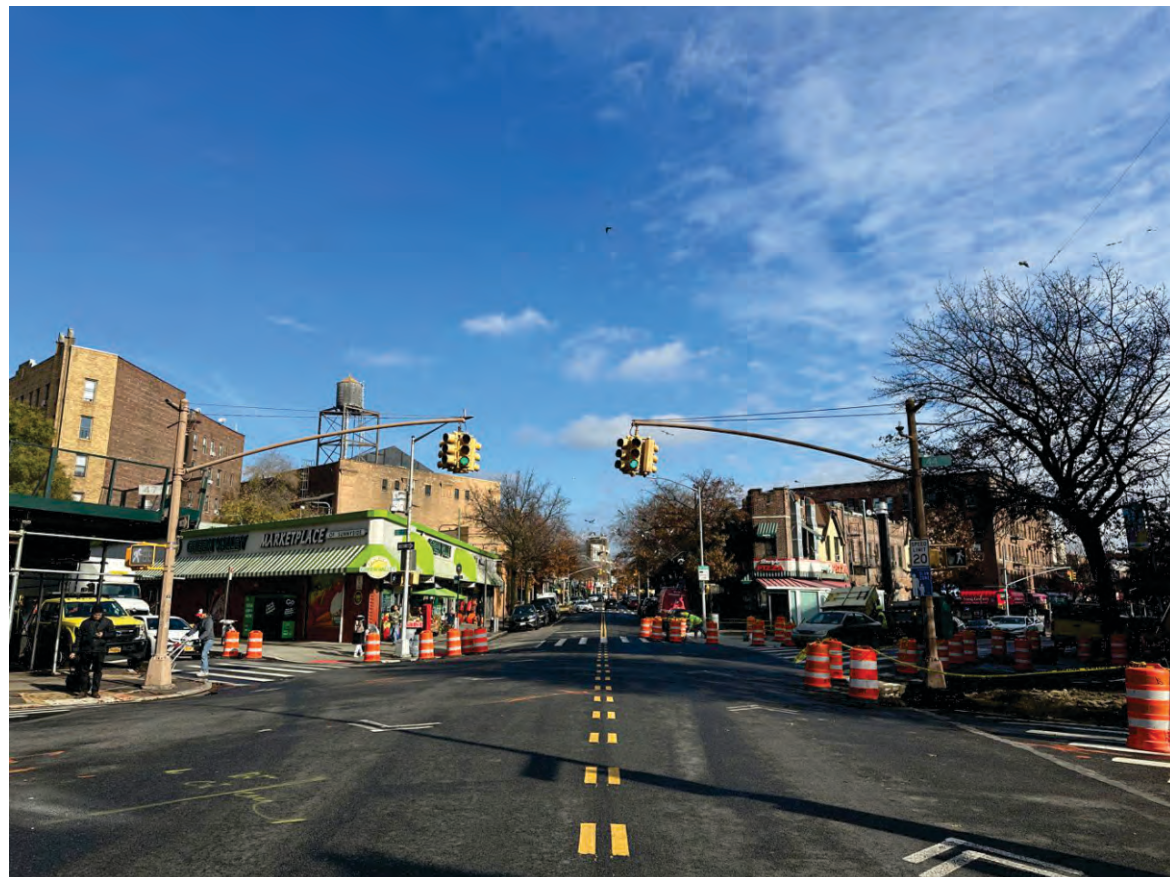
18. View of Greenpoint Avenue facing northeast from 44th Street (Project Area at left).
