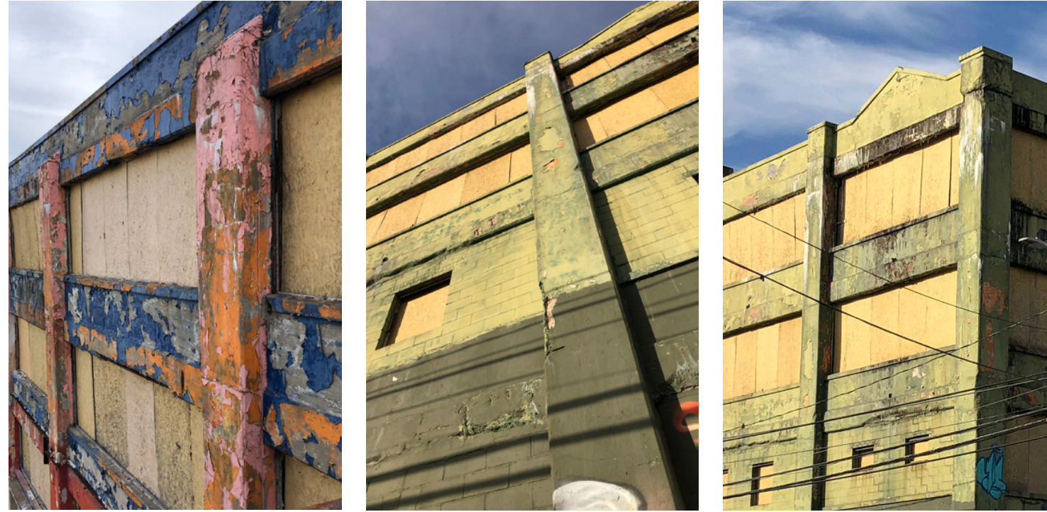
Existing Condition of Paragon Paint Building
