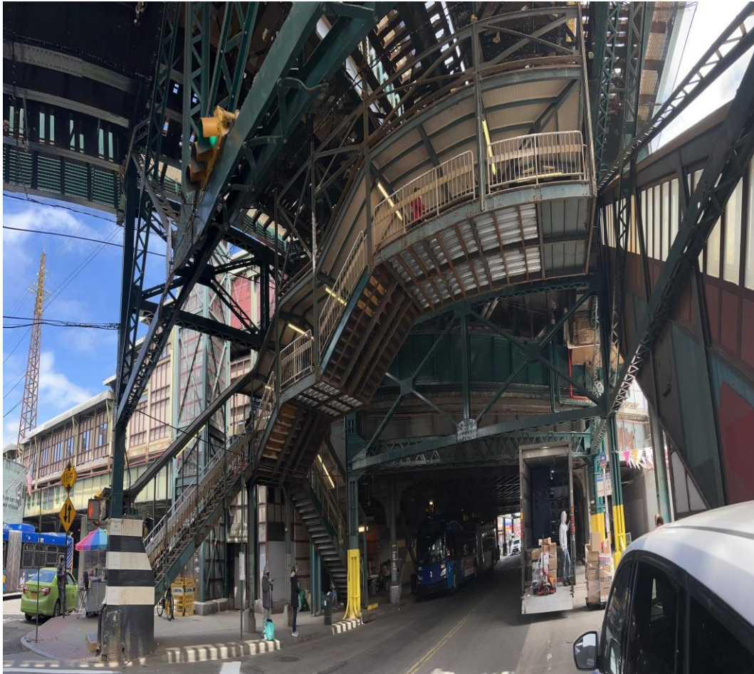
61st Woodside Street to Mezz Stairs
