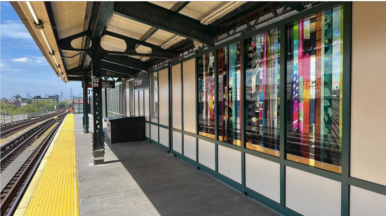
Completed 52 St Manhattan Bound Platform
