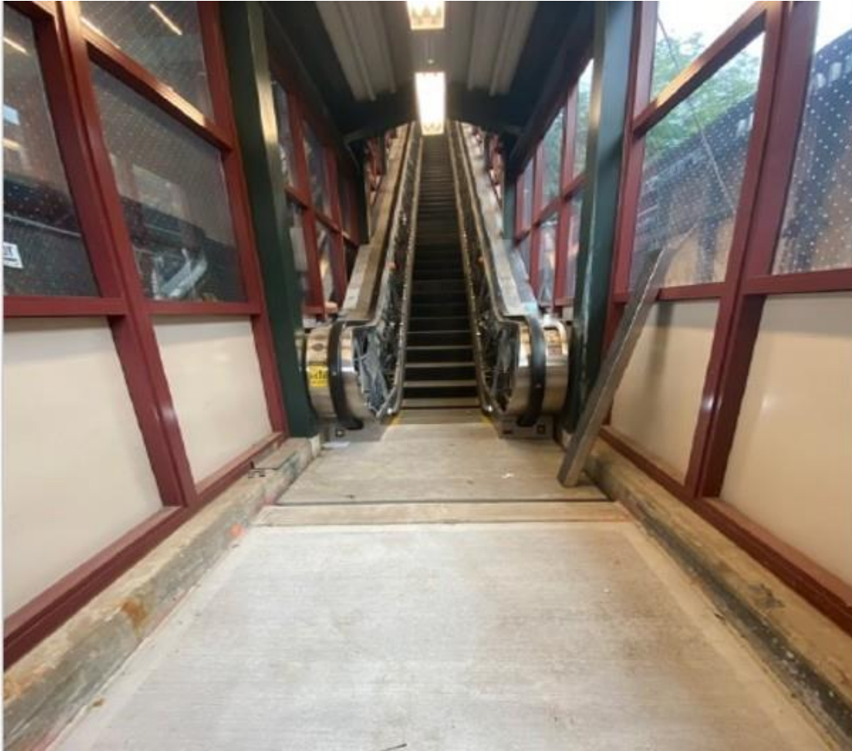
New Escalator and storefront build-up
