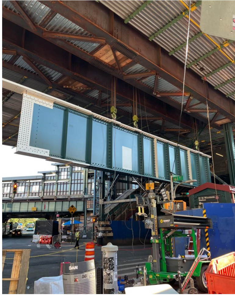
New Steel girder replacement- 95Ft long
