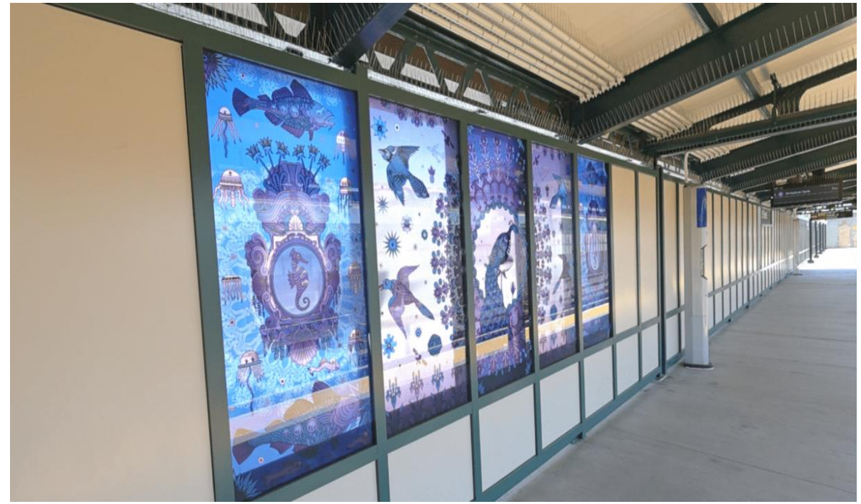
Completed 69 St Manhattan Bound Platform
