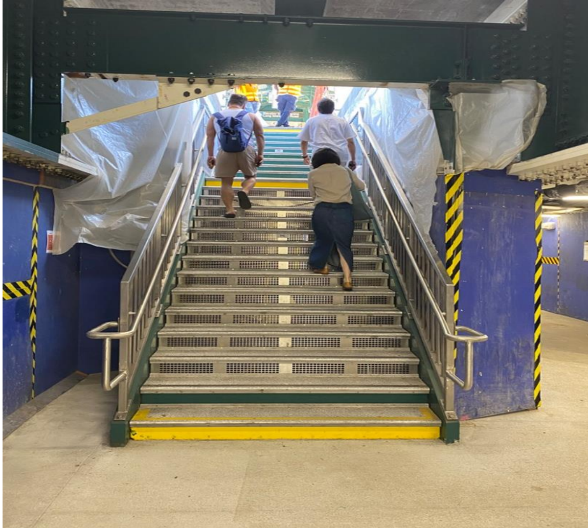
New ADA Compliant Stairs - East
