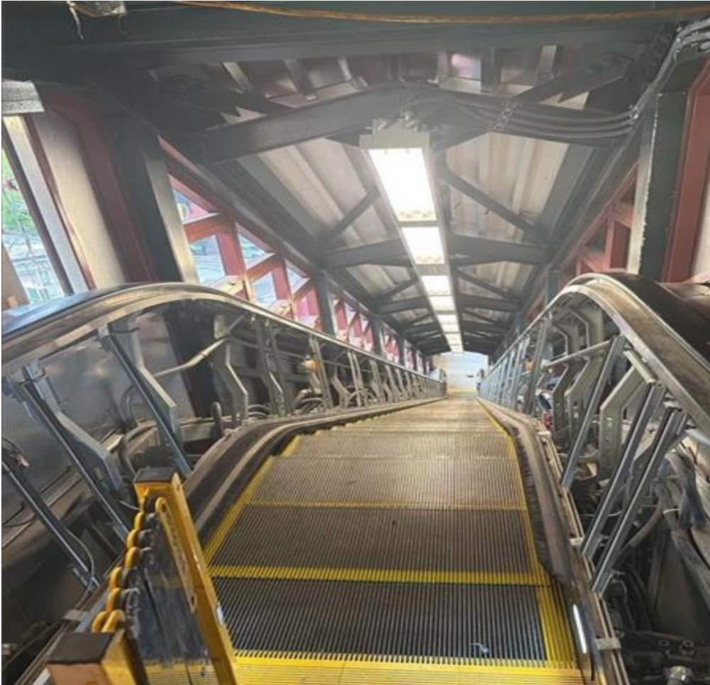
New Escalator Construction Work in Progress
