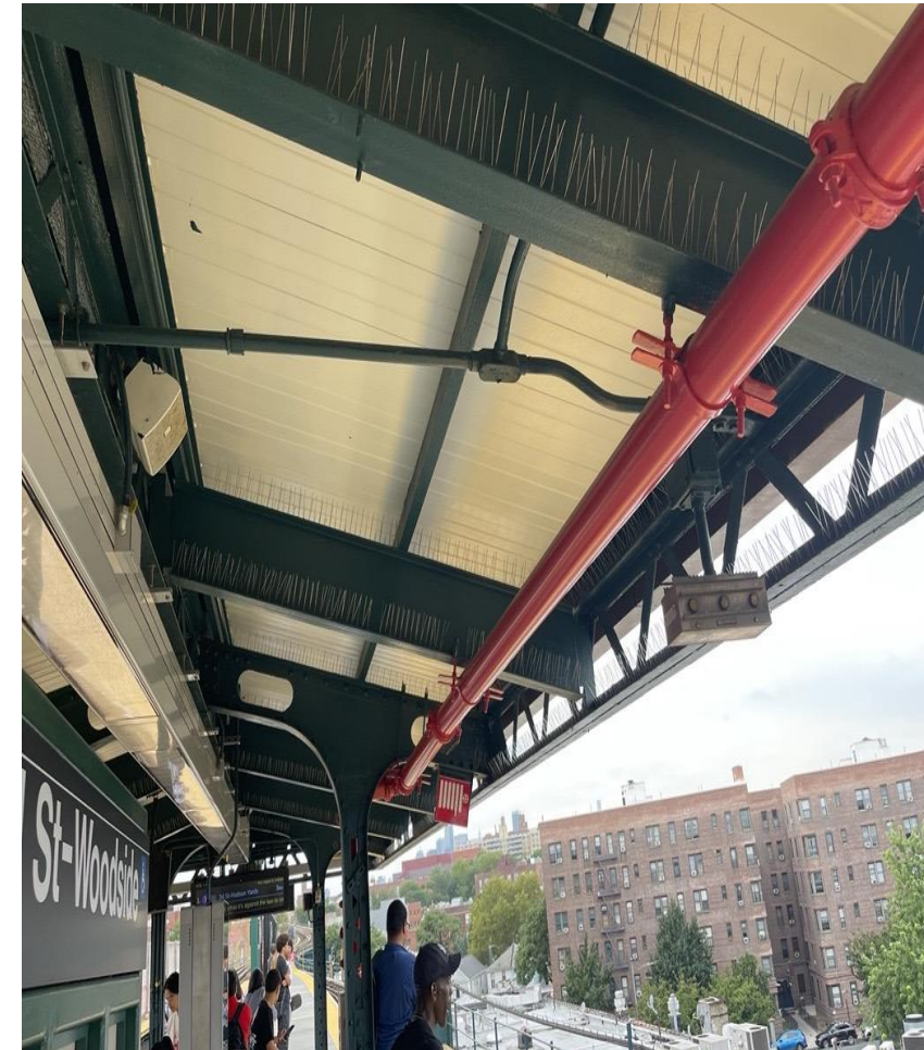
New Bird Spikes and Netting
