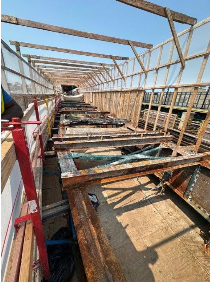
52 St Flushing Bound Platform
