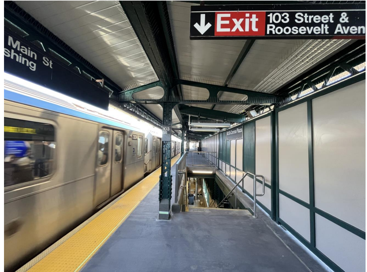
Completed Flushing Bound Platform
