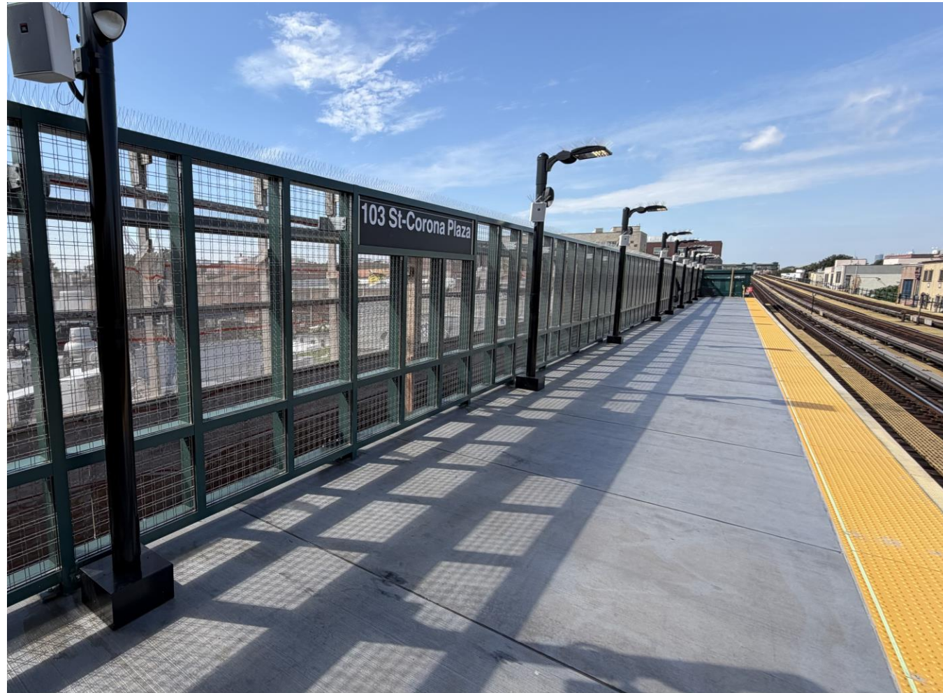
Completed Flushing Bound Platform
