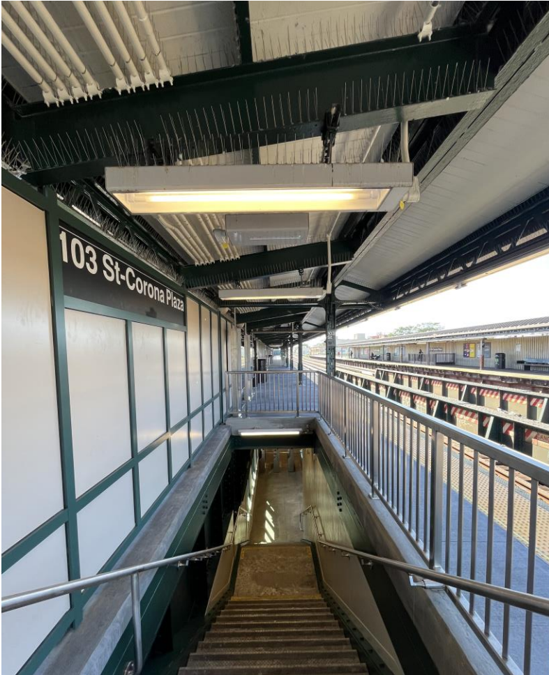
Completed Flushing Bound Platform
