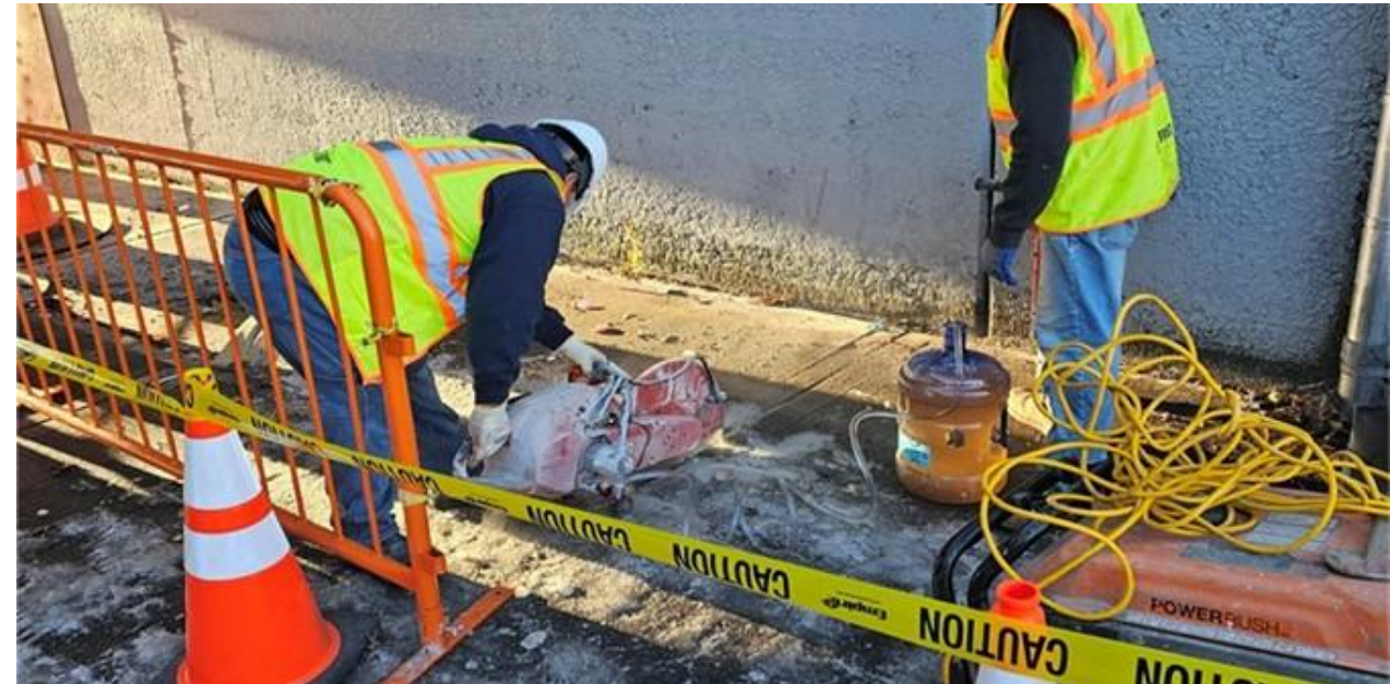
Test Pit Operations on Cypress Avenue
