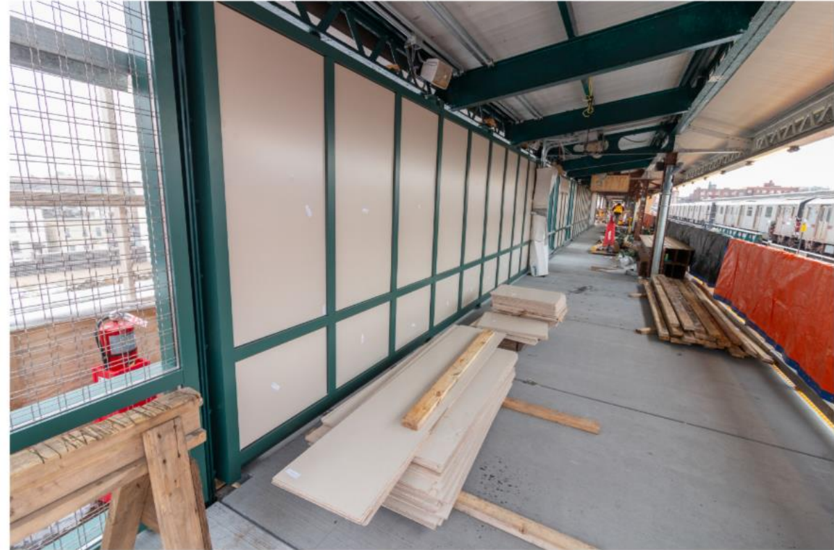
69 th Street SB Platform windscreen with fill-in Installation
