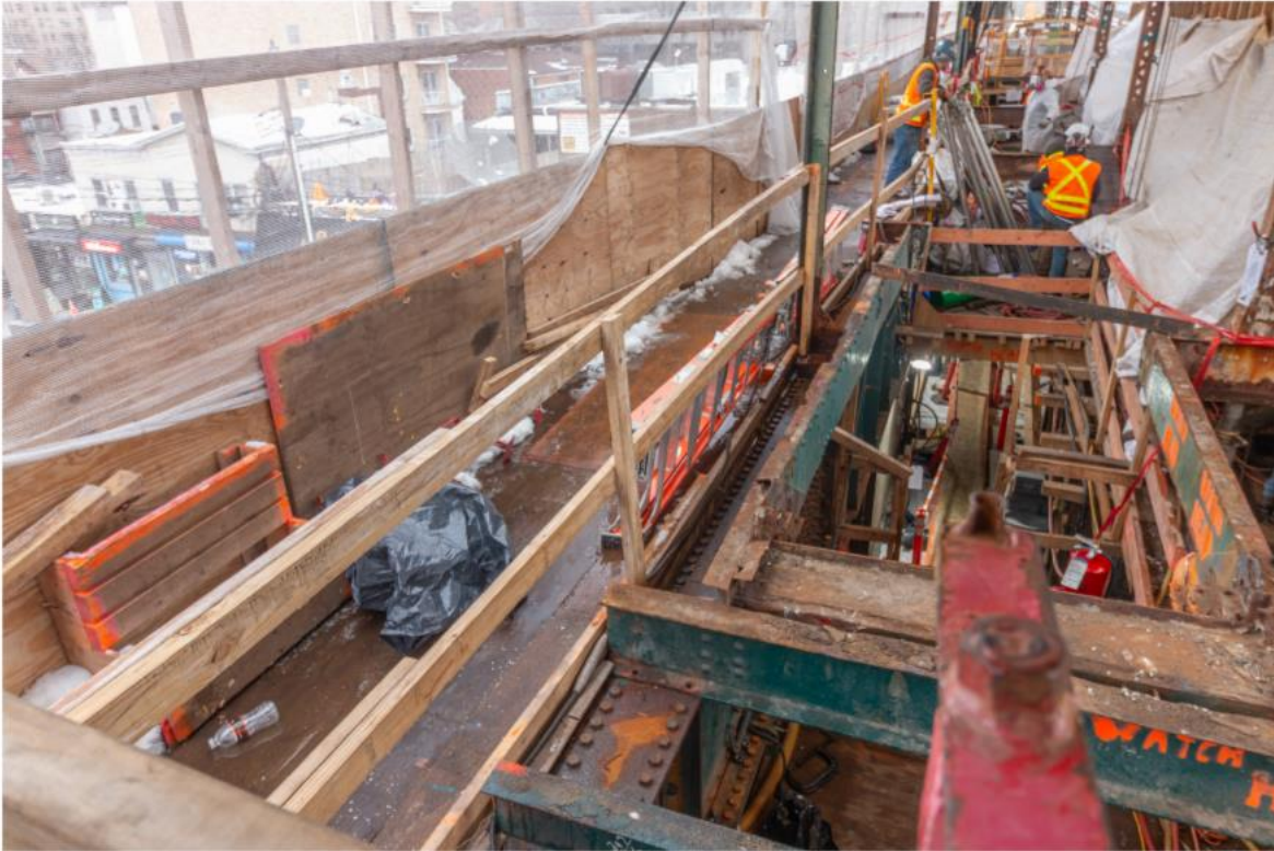
69 th Street SB Platform Continuation of Thru-span repair
