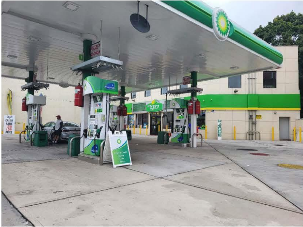
Front view of lot on Borden Avenue
