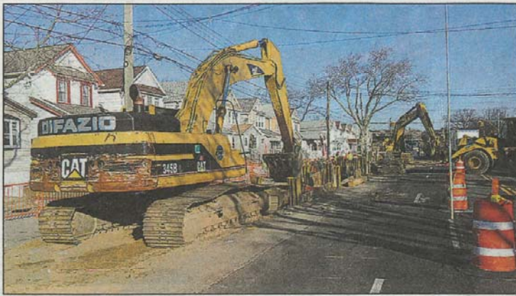
Construction workers on Francis Lewis Boulevard continue project QED-976 — installation of a trunk water main and a sewer line up Francis Lewis and along 90th Avenue in Queens Village. The $48 million project is scheduled to be completed in summer 2020. PHOTO BY MICHAEL GANNON
