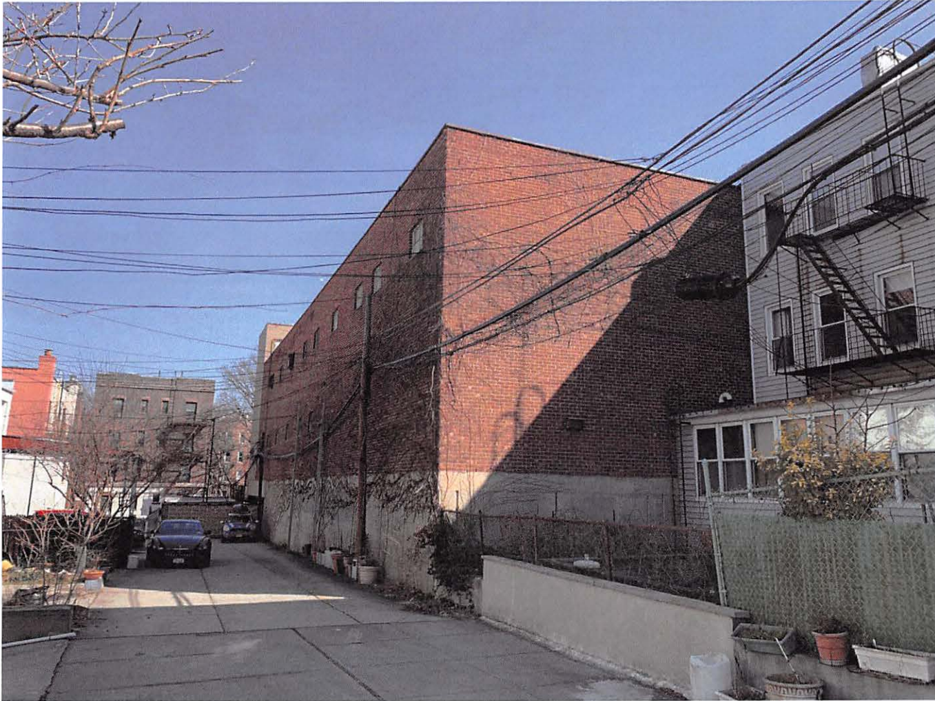
EXISTING REAR WALL OF SCHOOL From Alley
