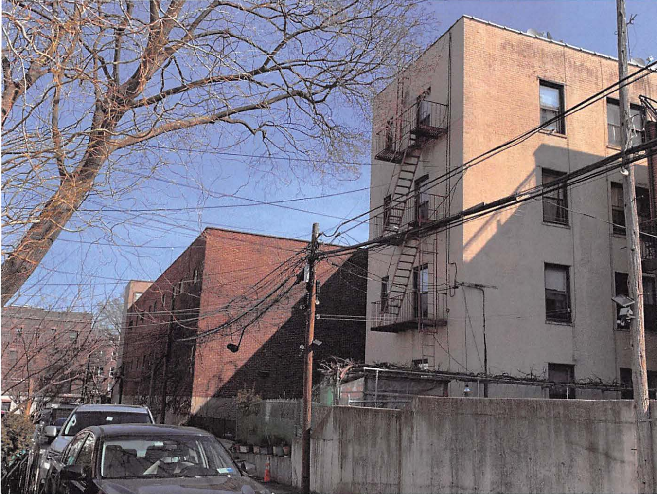
EXISTING REAR WALL OF SCHOOL From Alley
