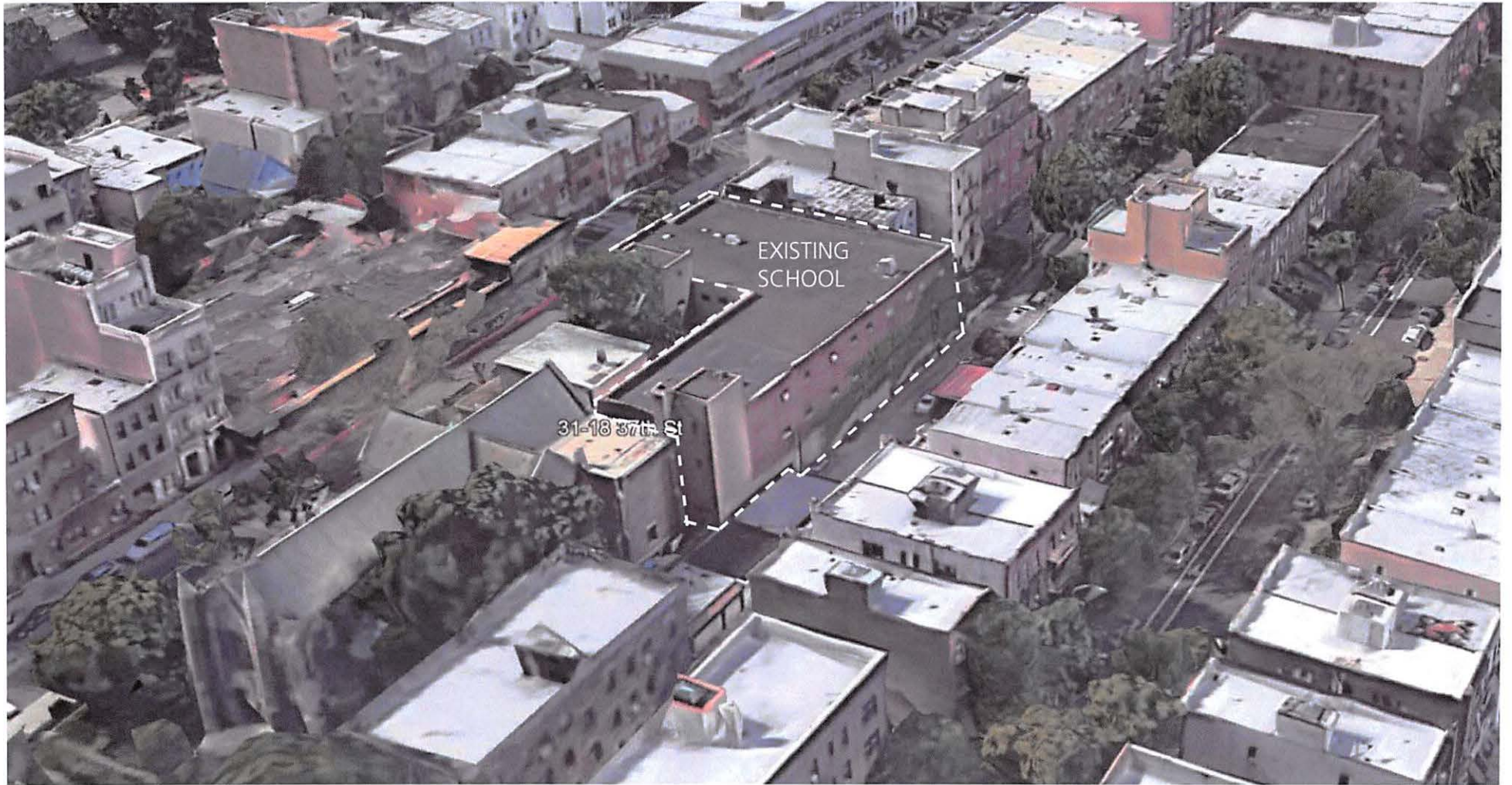
EXISTING SCHOOL View of Rear Wall From Northwest
