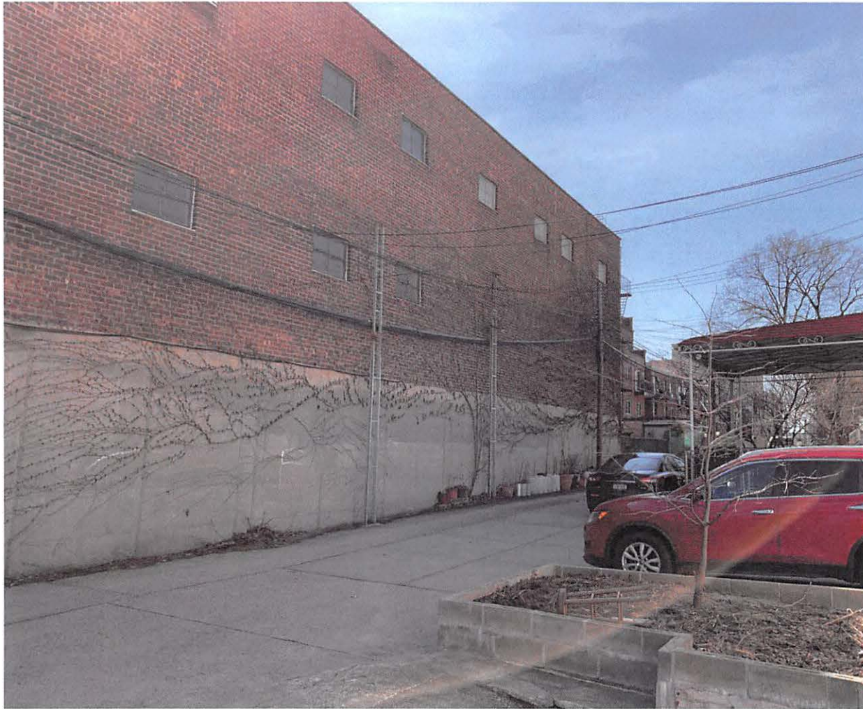
EXISTING REAR WALL OF SCHOOL From Alley
