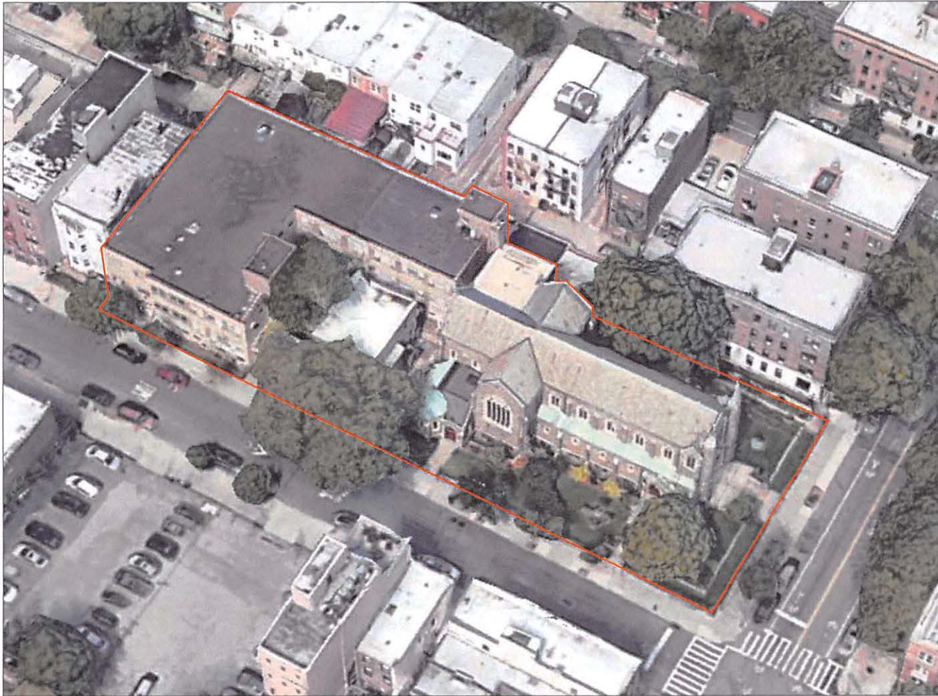
SITE - AERIAL VIEW FROM EAST
