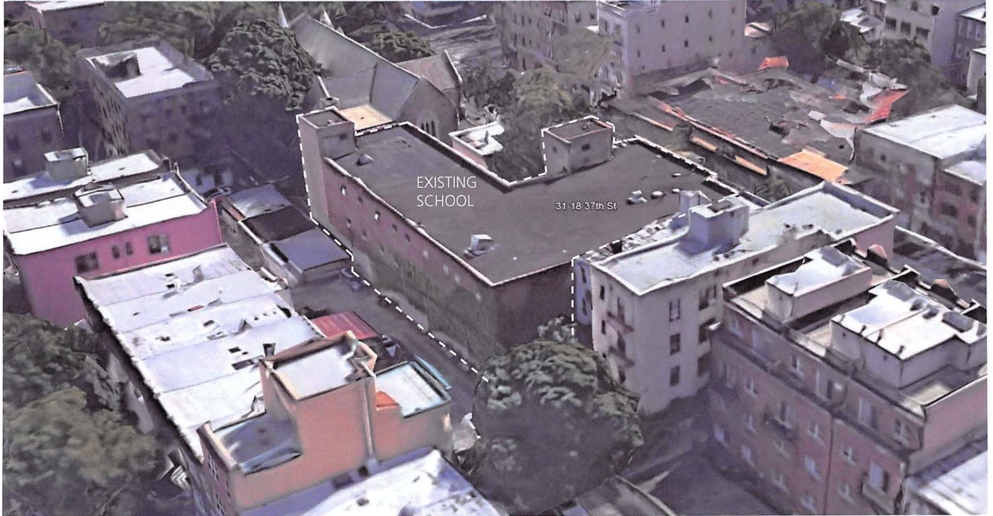
EXISTING SCHOOL View of Rear Wall From Southwest
