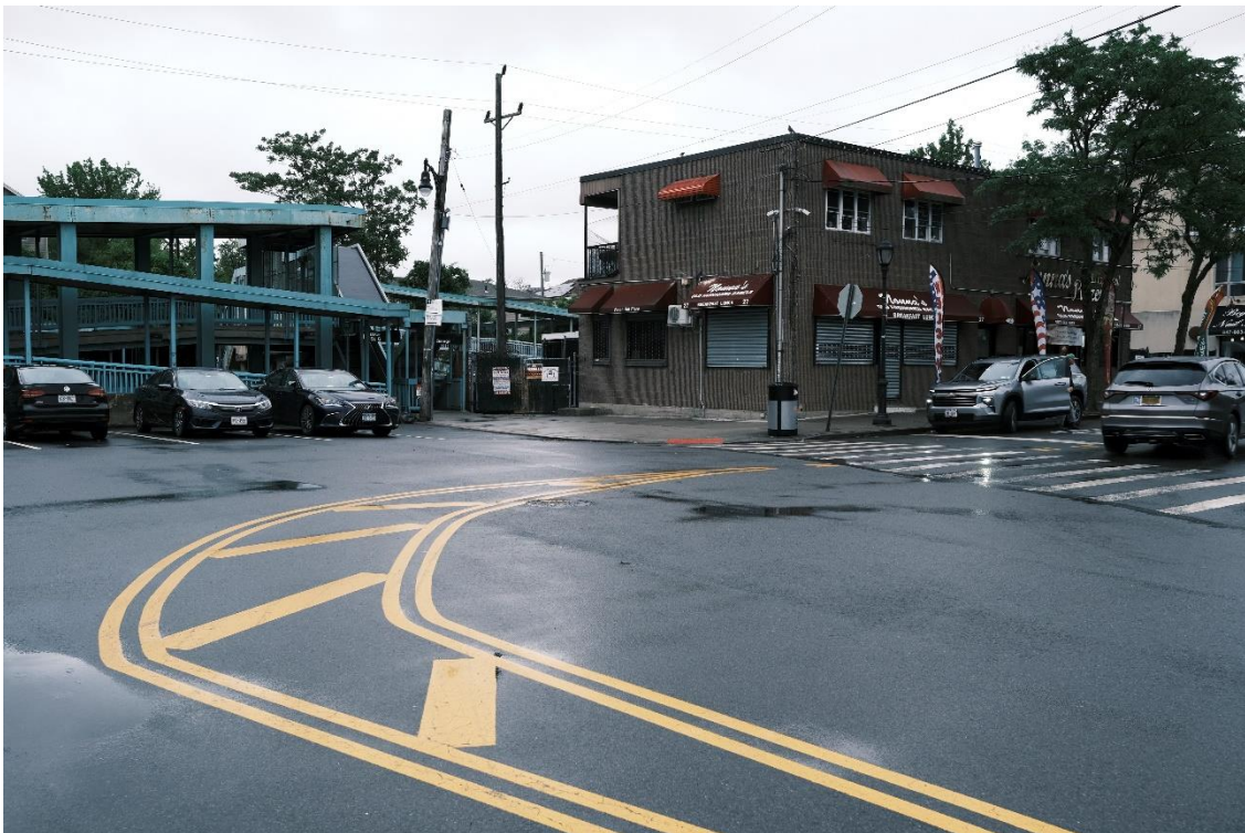
Image 3: Great Kills SIR Station – Accessible Ramp and Parking Area
