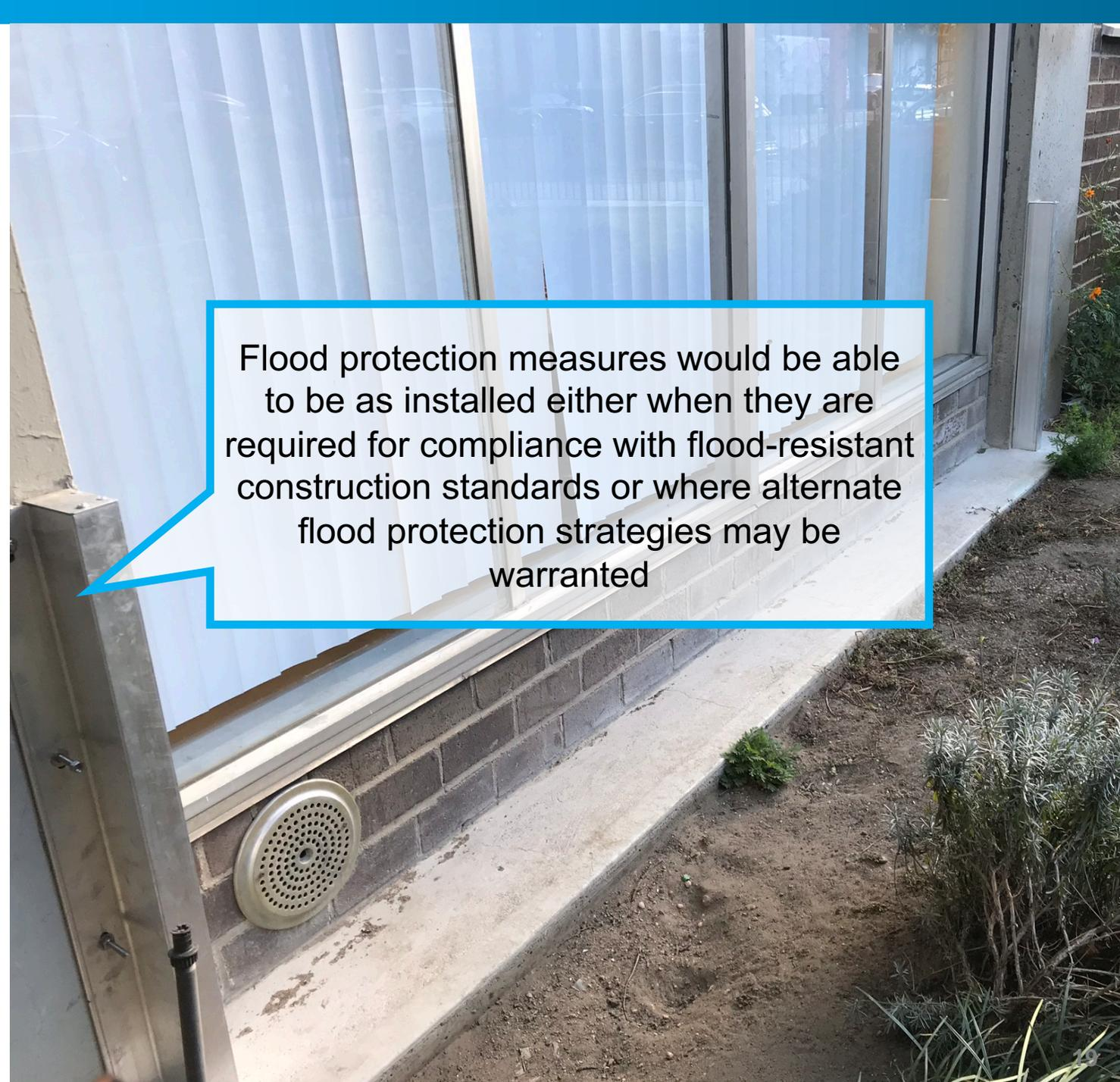
Flood protection measures would be able to be as installed either when they are required for compliance with flood-resistant construction standards or where alternate flood protection strategies may be warranted
