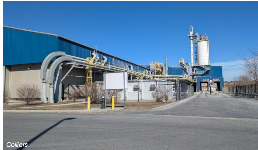
Concrete Batching Facility
