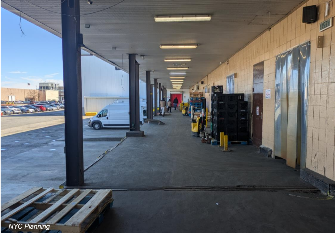
An example outdated industrial building with low ceiling heights and insufficient operational space
