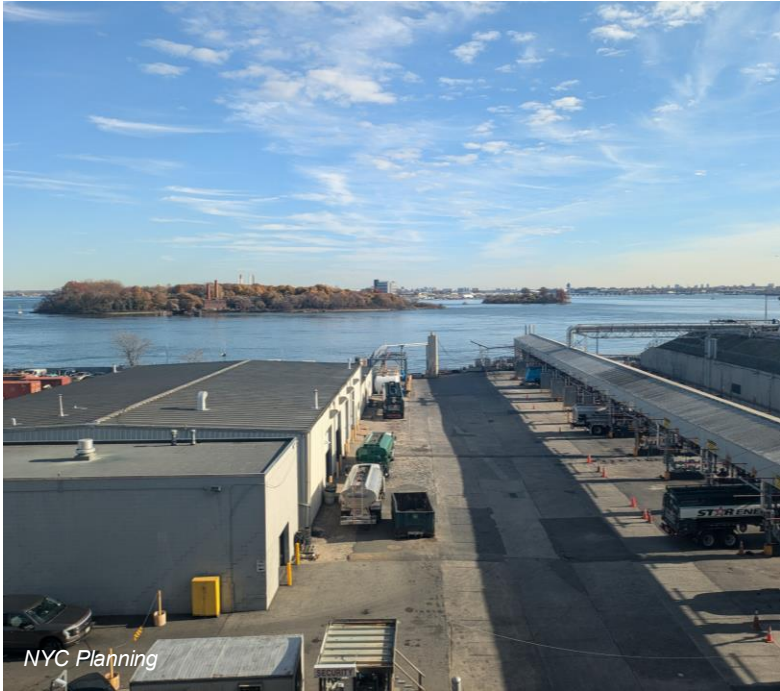
Blocked off waterfront access
