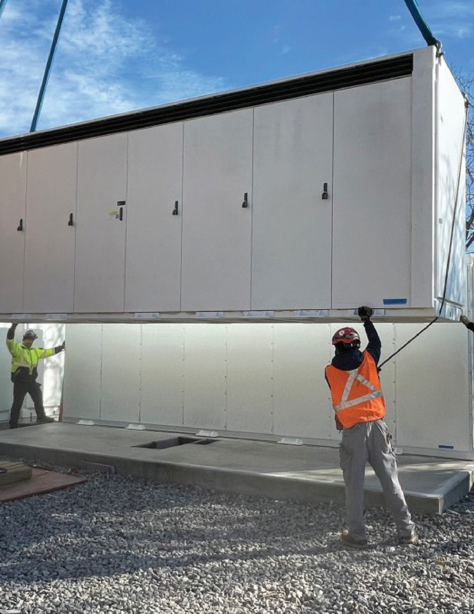
◀ Figure 1: NineDot Energy installs a battery storage system in NYC. Source: NineDot Energy
