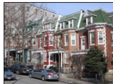
Attached homes on Perry Avenue in a proposed R5B area
