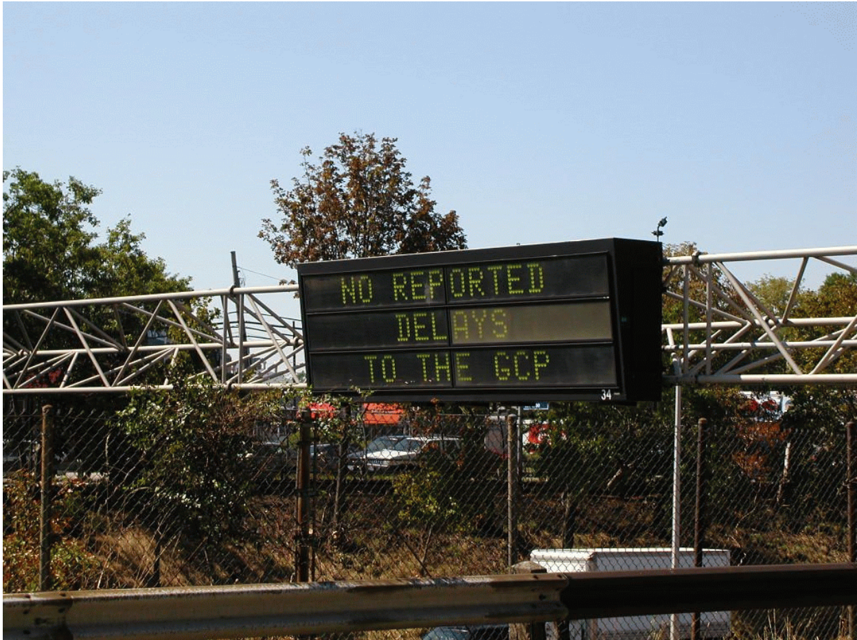
Figure 3 VMS on the Long Island Expressway, displaying real-time traffic information.
